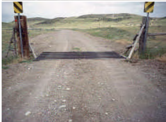
Example of good work done to reshape a roadway approaching a cattle guard and maintaining a very smooth crossing.
