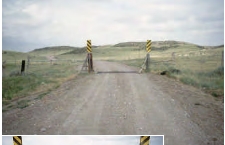
Example of good work done to reshape a roadway approaching a cattle guard and maintaining a very smooth crossing.
