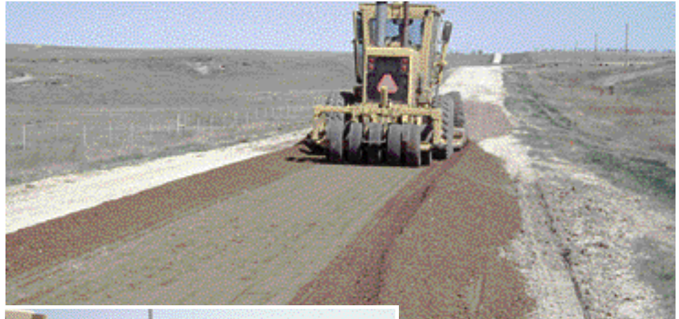
A grader-mounted roller being used on a rural gravel road. This department owns three of these units.
