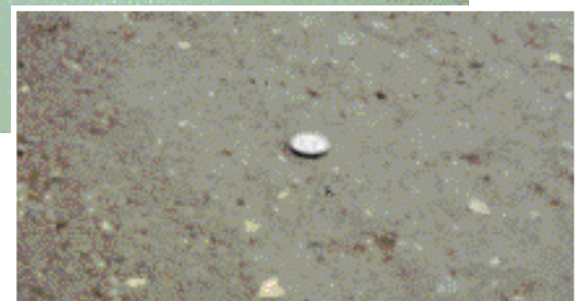
Notice the good blend of stone, sand and fine-sized particles tightly bound together on this road surface.
