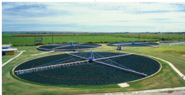
Trickling Filters
