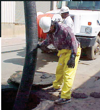
Sewer line maintenance
