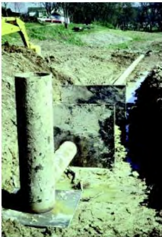
Figure 22 Drop-inlet pipe spillway with antiseep collar
