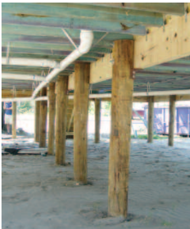
Round timber piling
