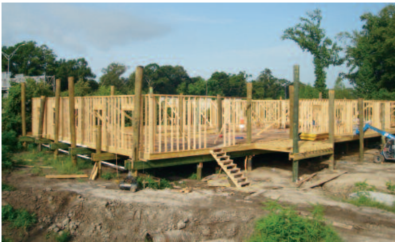
Round Timber piling and glulam floor beams
