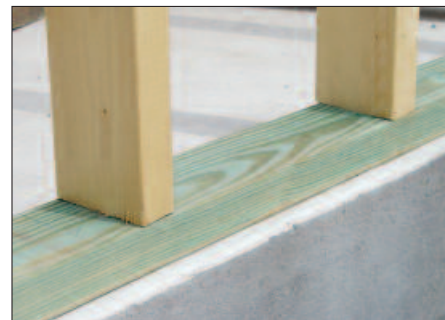
Building codes require that wood components in contact with concrete, masonry, or the ground be pressure treated or naturally durable.
