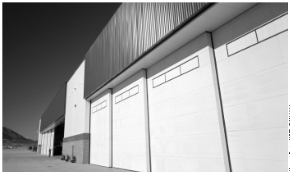
Figure 6. The transpired collector on the Avum Hangar at Fort Carson, Colorado.
