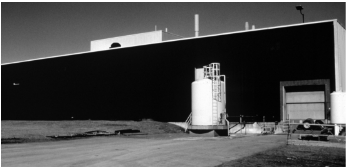
Figure 12. The transpired collector on the GM Battery Plant in Oshawa, Canada.
