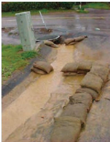
Figure 5. Make sure storm drain inlets are protected.
