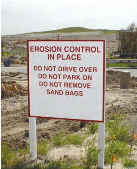
Figure 4. Use signage to help educate construction staff.
