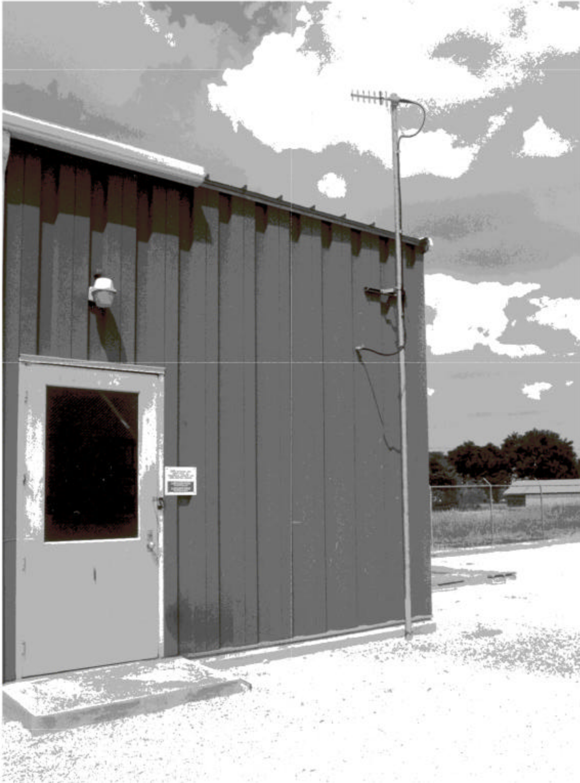
Figure 17-6: MAS Microwave Antenna on Substation Control House
