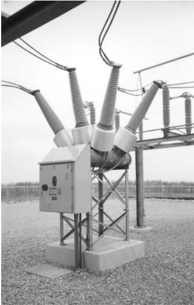
Figure 5-2: "Dead Tank" Breaker (Courtesy of Mitsubishi)
