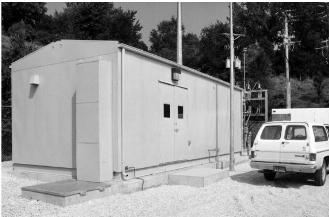
Figure 16-1: Pre-Engineered Metal Control Building (Coffeyville, KS)
