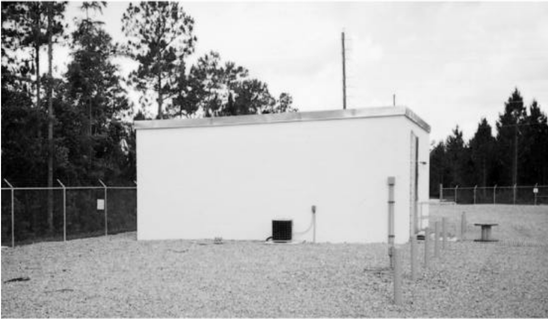
Figure 16-2: Typical Masonry Block Control Building
