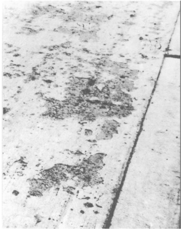
Figure 5-4. Light scale.
