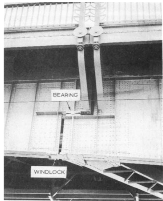
Figure 3-13. Bearing support for a suspended span.
