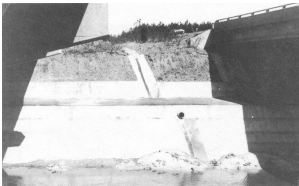
Figure 5-38. Concrete slope protection.
