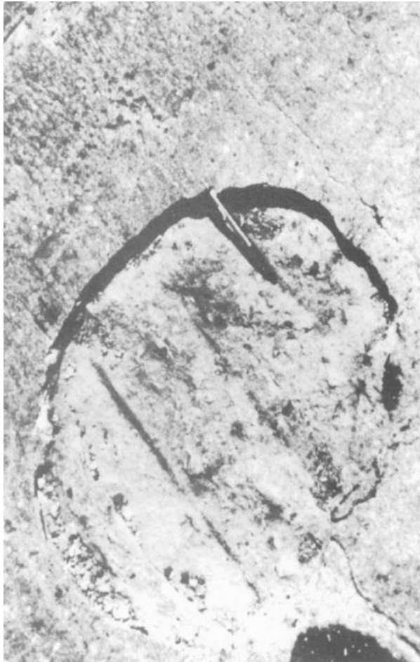
Figure 5-8. Large spall.
