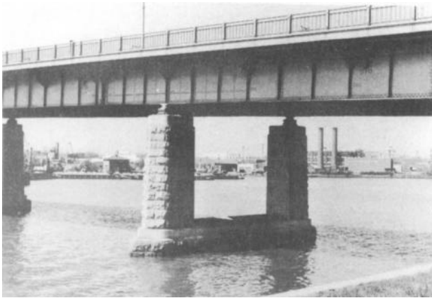
Figure 6-1. Nonload path redundant bridges.
