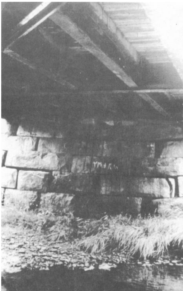
Figure 5-20. Differential settlement.
