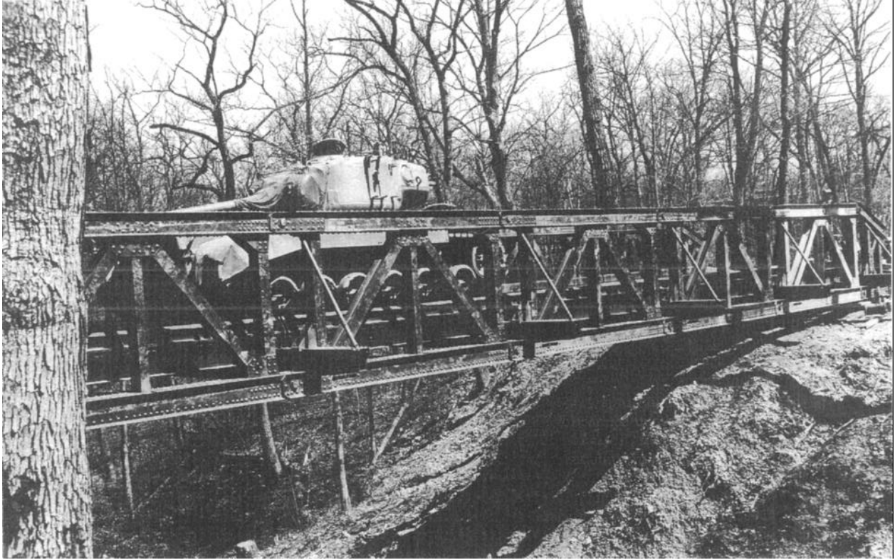
Figure 2-8. T6 aluminum fixed bridge.
