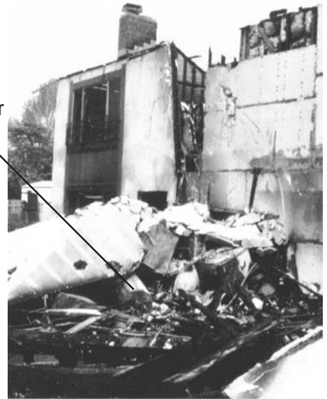
Figure 7 - The unbraced water heater in this home fell during an earthquake; the resulting fire destroyed the home.
