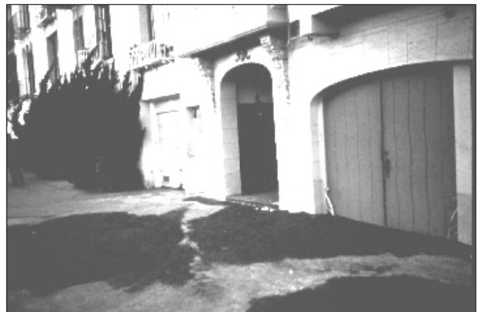
Figure 36 - Loma Prieta Earthquake, October 17, 1989. Lateral spreading, liquefaction and sand boils caused extensive damage in the Marina District of San Francisco, about 60 miles away from the epicenter.
