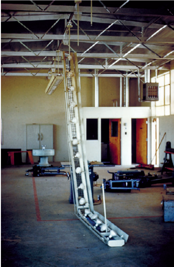
Figure 4-16: Overturned shop equipment and failed light fixtures, Kern County, CA, 1952
