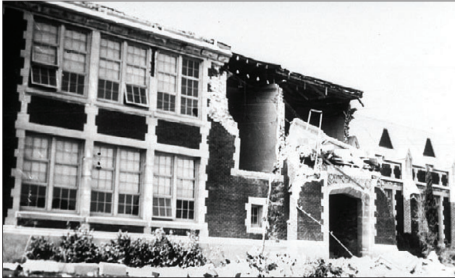
Figure 4-12: Damage to the John Muir School, Long Beach, CA, 1933
