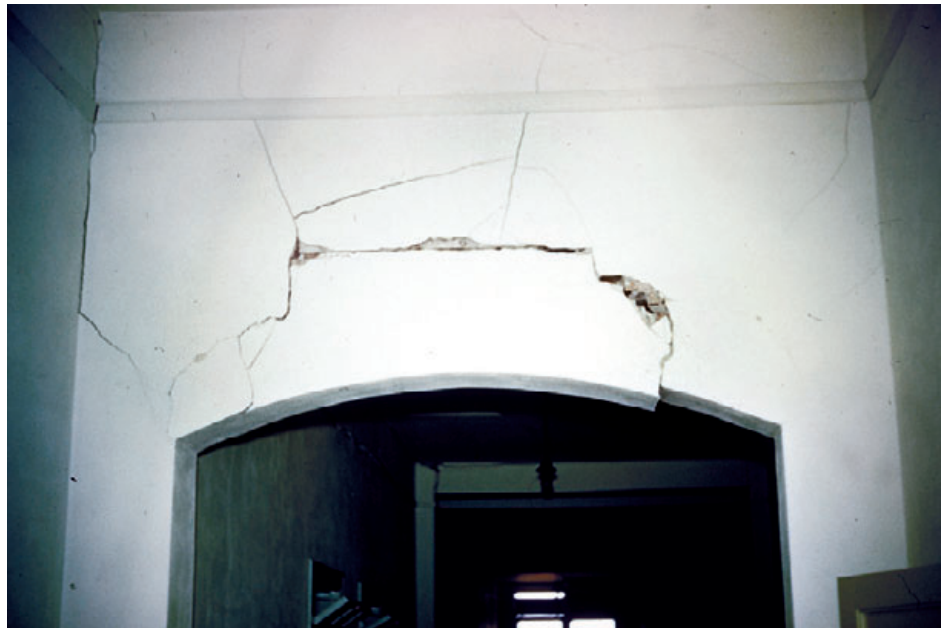
Figure 4-15: A heavy corridor lintel ready to fall, Emerson School, Bakersfield, Kern County, CA, 1952
