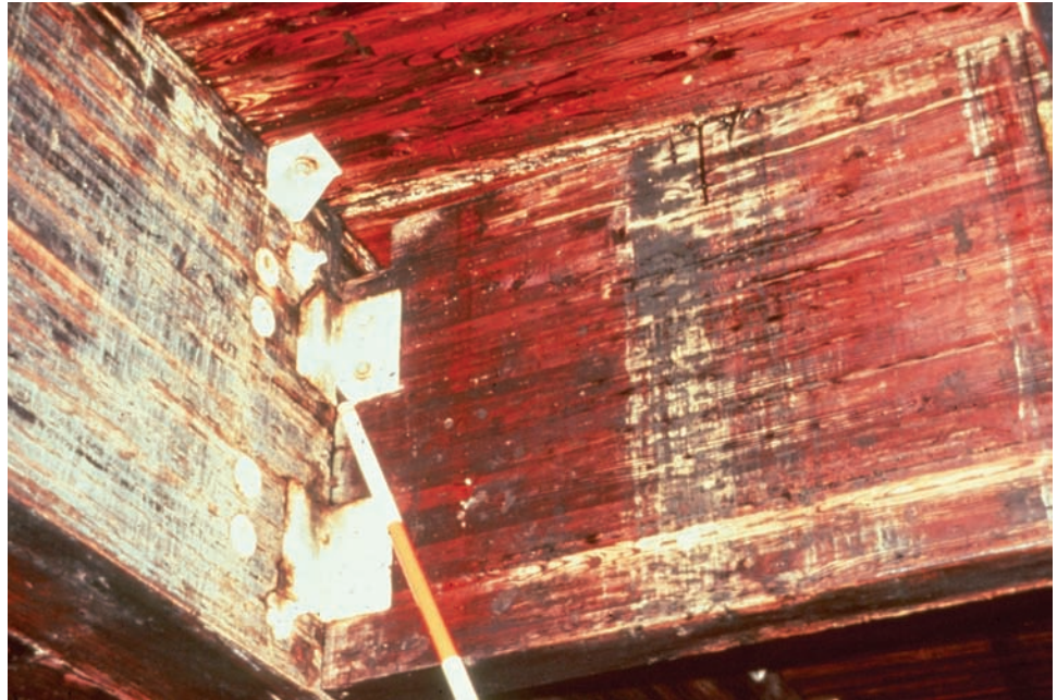
Figure 6.2.13 Typical Diaphragm for a Glulam Multi-beam Bridge
