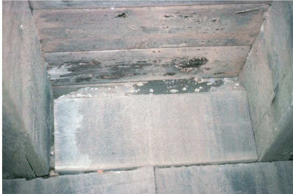
Figure 6.1.14 Typical Timber End Diaphragm
