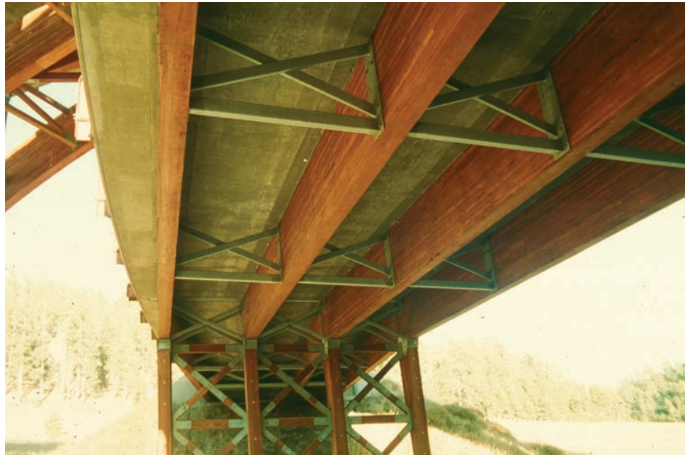
Figure 6.2.14 Glulam Beams with Numerous Fastener Locations
