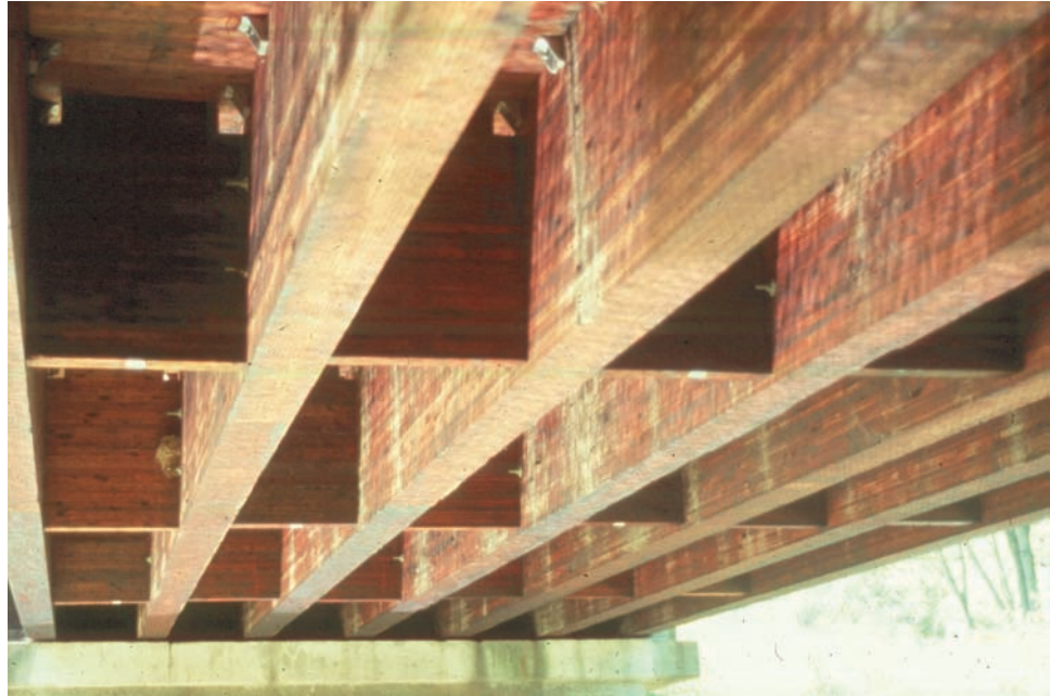
Figure 6.2.2 Underside View of a Glulam Multi-beam Bridge
