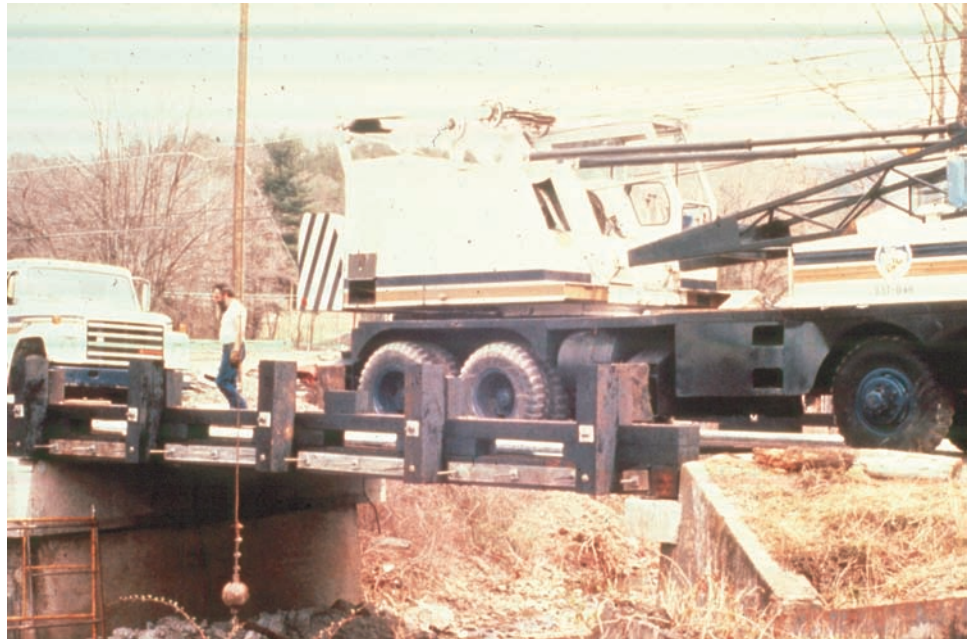
Figure 6.3.3 Stress-Laminated Timber Slab Bridge
