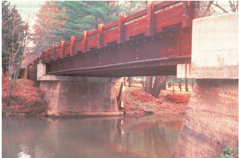
Figure 6.2.1 Elevation View of a Glulam Multi-beam Bridge
