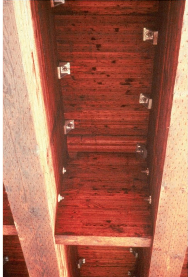
Figure 6.2.8 Typical Glulam Diaphragm
