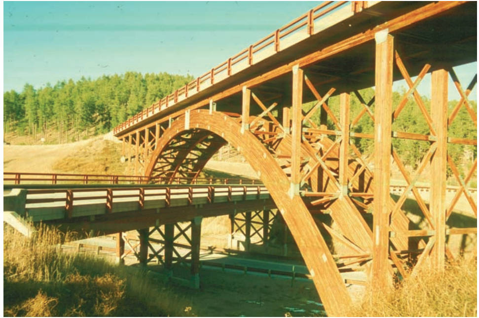
Figure 6.2.6 Glulam Arch Bridge over Glulam Multi-beam Bridge (Keystone Wye interchange, South Dakota)
