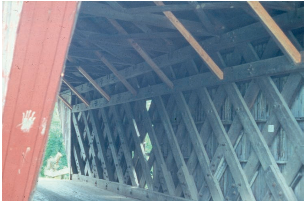
Figure 6.1.10 Town Truss Design
