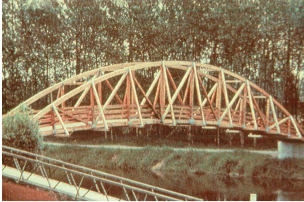
Figure 6.2.4 Bowstring Truss Pedestrian Bridge
