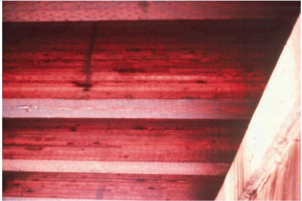
Figure 6.2.10 Close-up View of Glulam Bridge Showing Laminations
