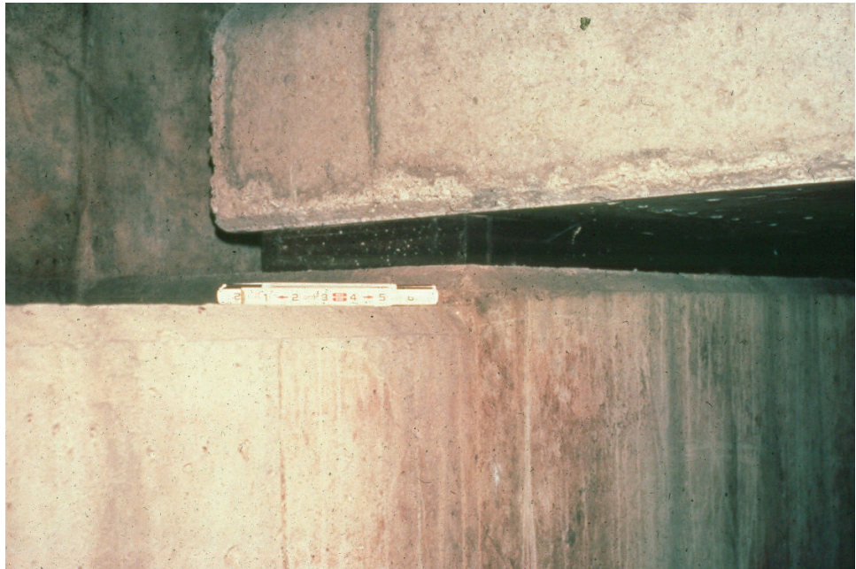
Figure 9.1.13 Plain Neoprene Bearing Pad
