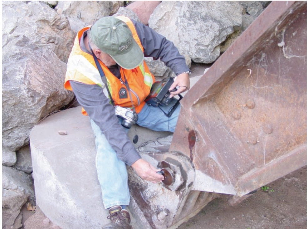
Figure 9.1.21 UT Inspection of a Pin in a Bearing
