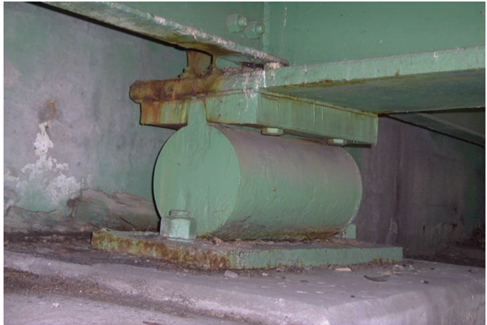
Figure 9.1.7 Single Roller Bearing
