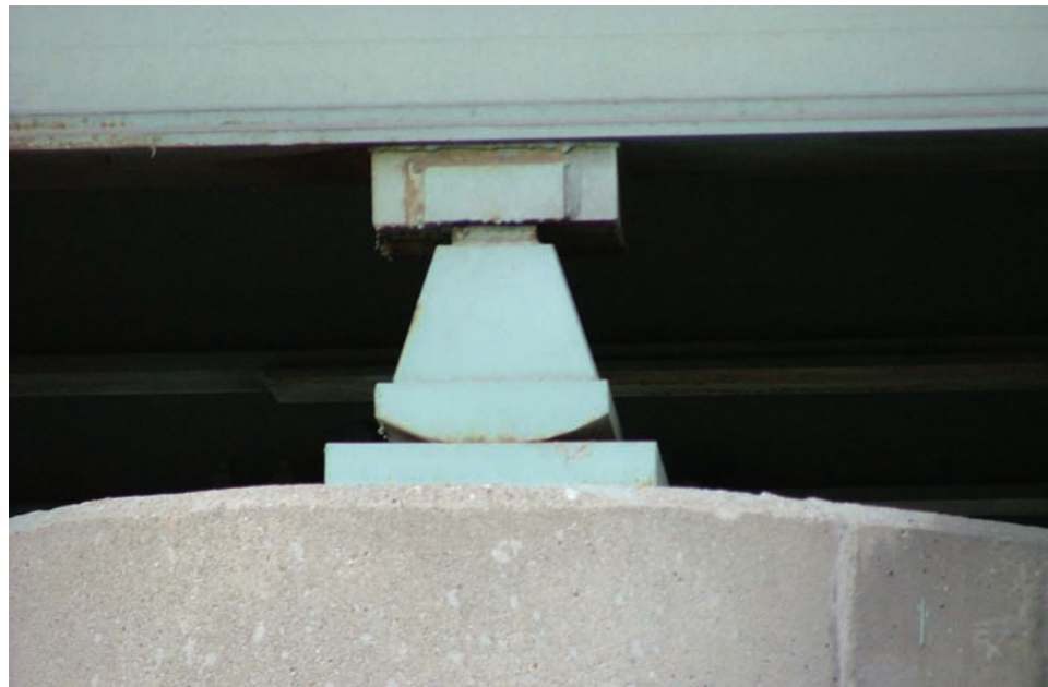
Figure 9.1.9 Rocker Bearing
