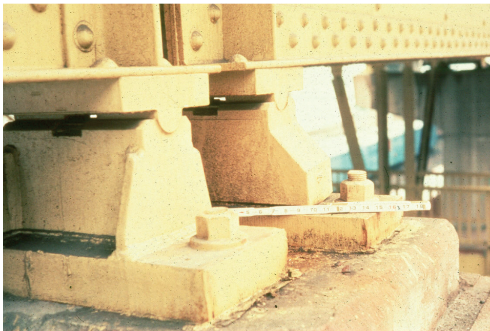
Figure 9.1.2 Fixed and Expansion Bearings
