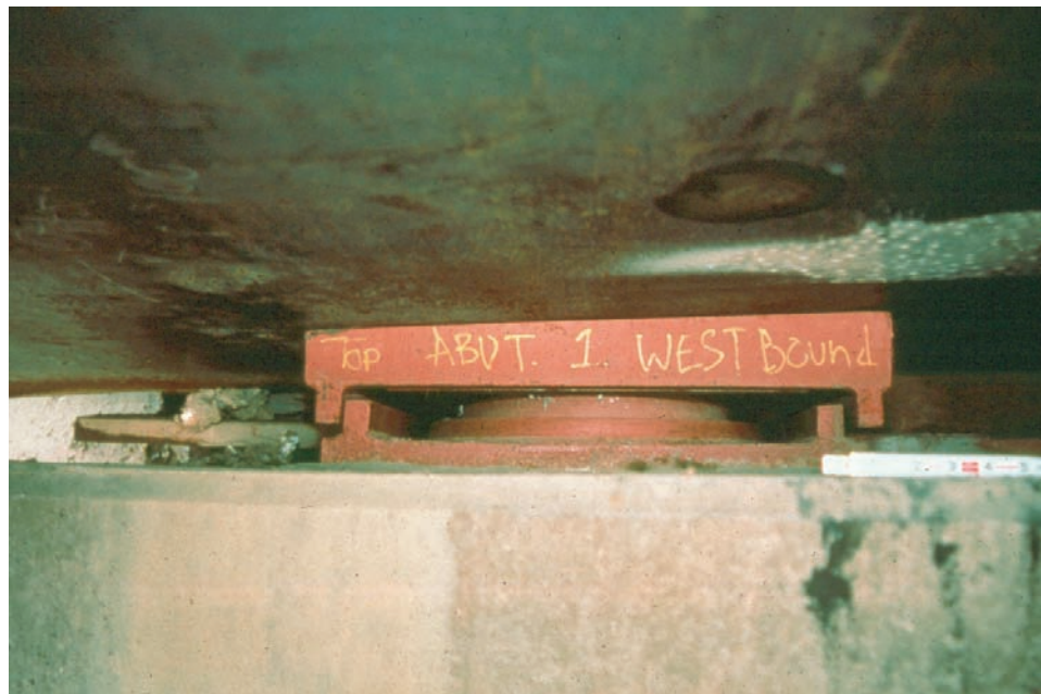
Figure 9.1.18 Pot Bearing
