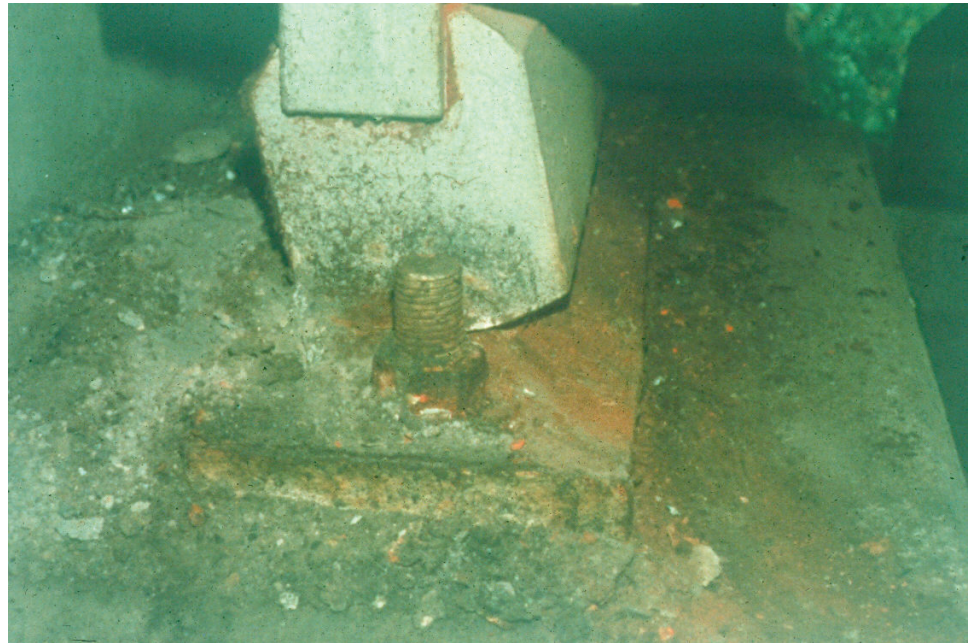
Figure 9.1.10 Segmental Rocker Bearing
