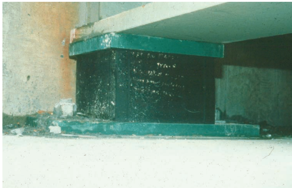
Figure 9.1.16 Lead Core Isolation Bearing
