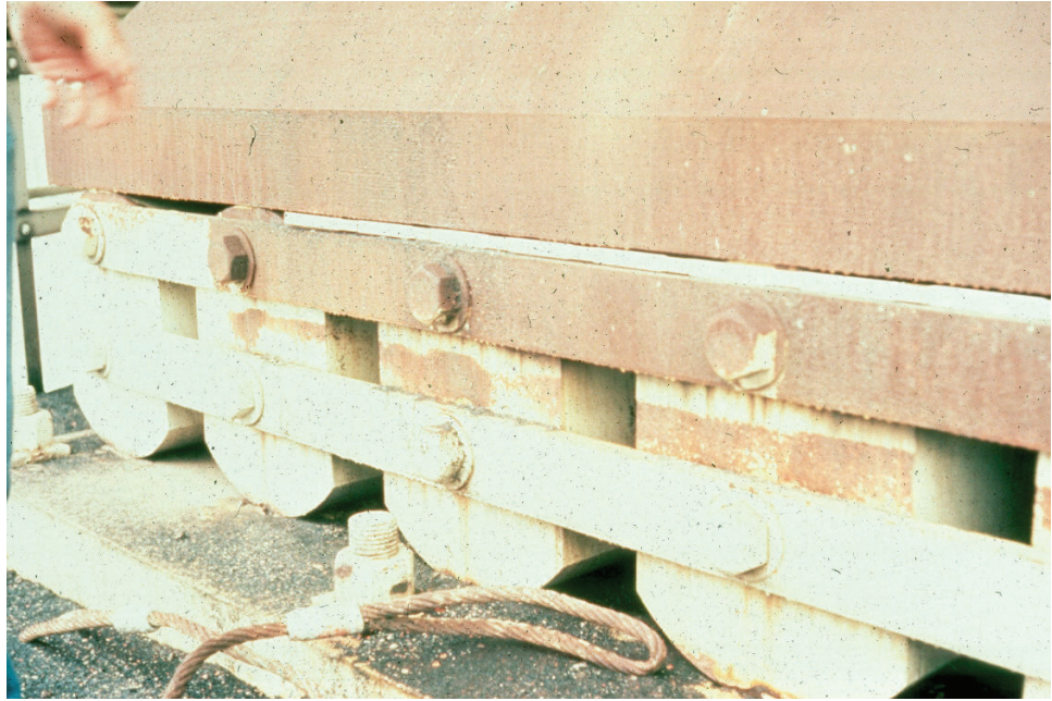
Figure 9.1.11 Segmental Rocker Nest Bearing
