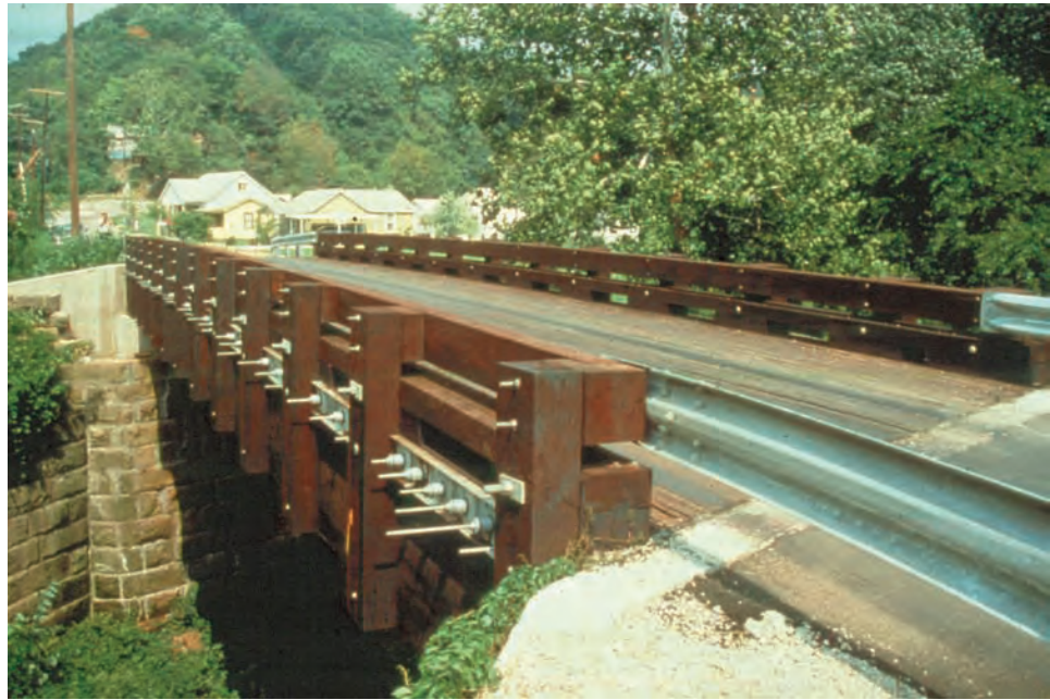
Figure 5.1.4 Stressed-laminated Deck
