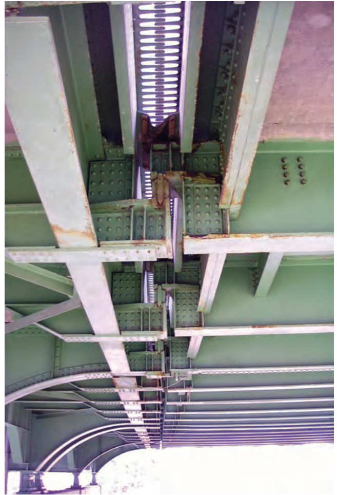
Figure 5.4.20 Support System under a Finger Plate Joint
