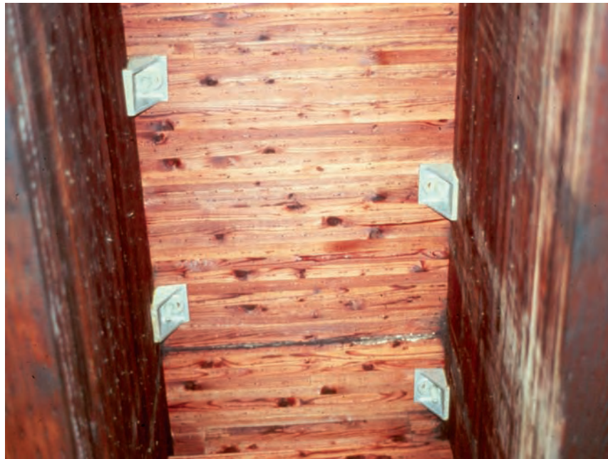
Figure 5.1.3 Glued-laminated Deck Panels
