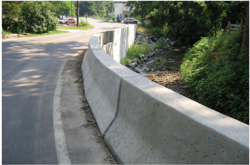
Figure 5.5.4 Acceptable Bridge Rail
