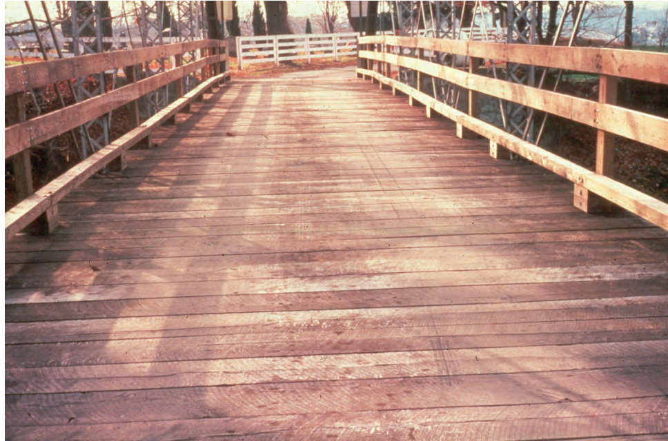
Figure 5.1.1 Plank Deck
