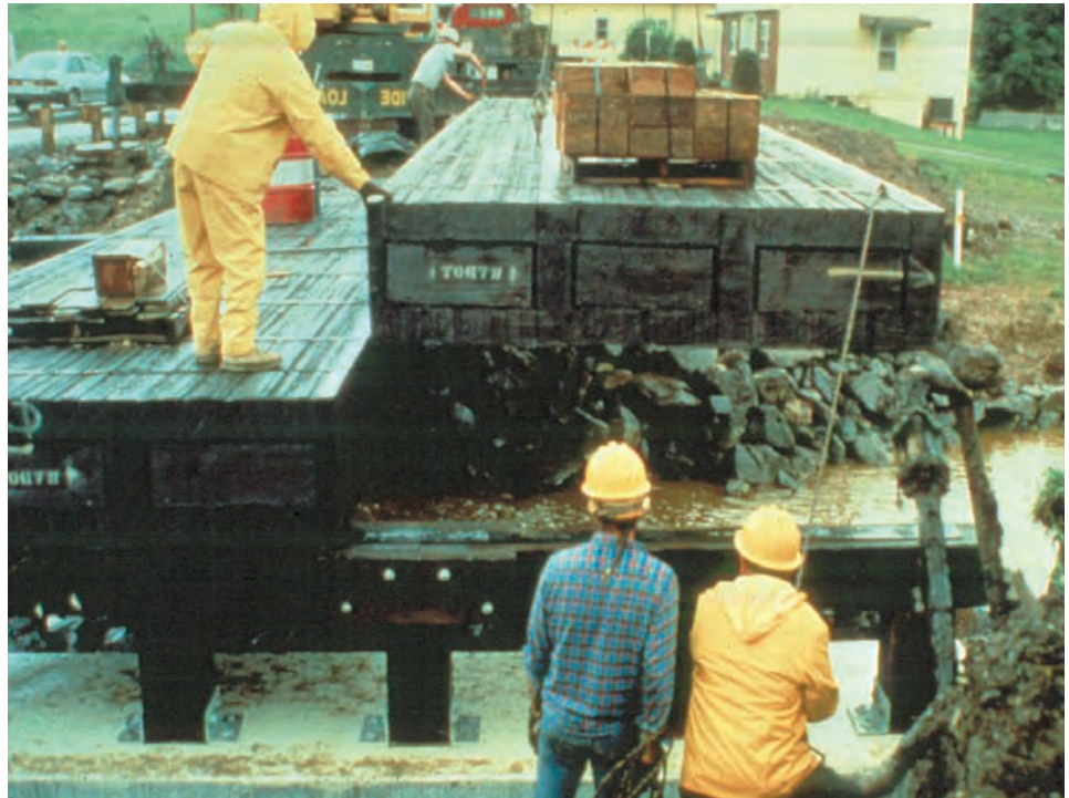
Figure 5.1.5 Structural Composite Lumber Deck Using Box Sections
