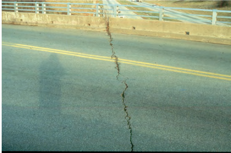
Figure 5.4.19 Asphalt Wearing Surface over an Expansion Joint
