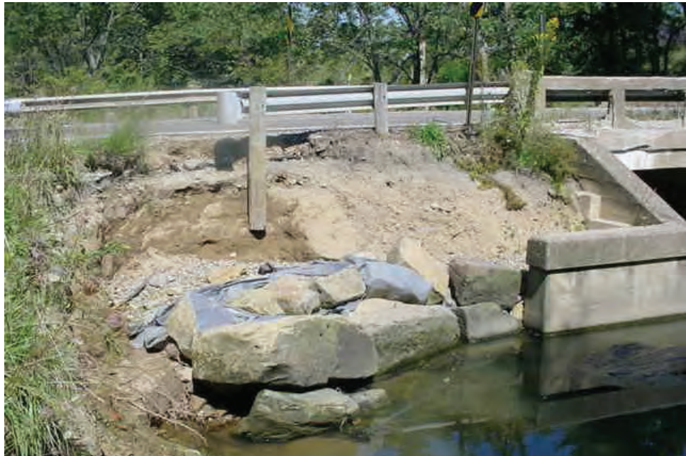
Figure 5.5.12 Erosion Reducing Post Embedment
