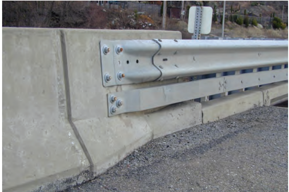
Figure 5.5.13 Proper Nesting of Guardrail at Transition
