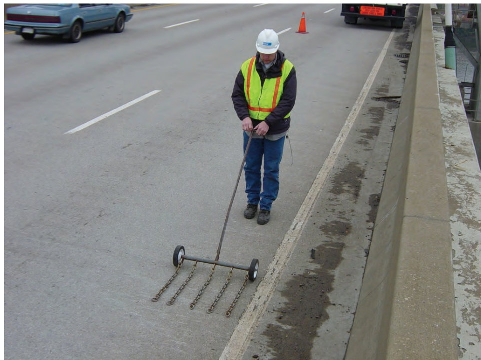
Figure 5.2.10 Sounding for Delaminated Areas of Concrete
