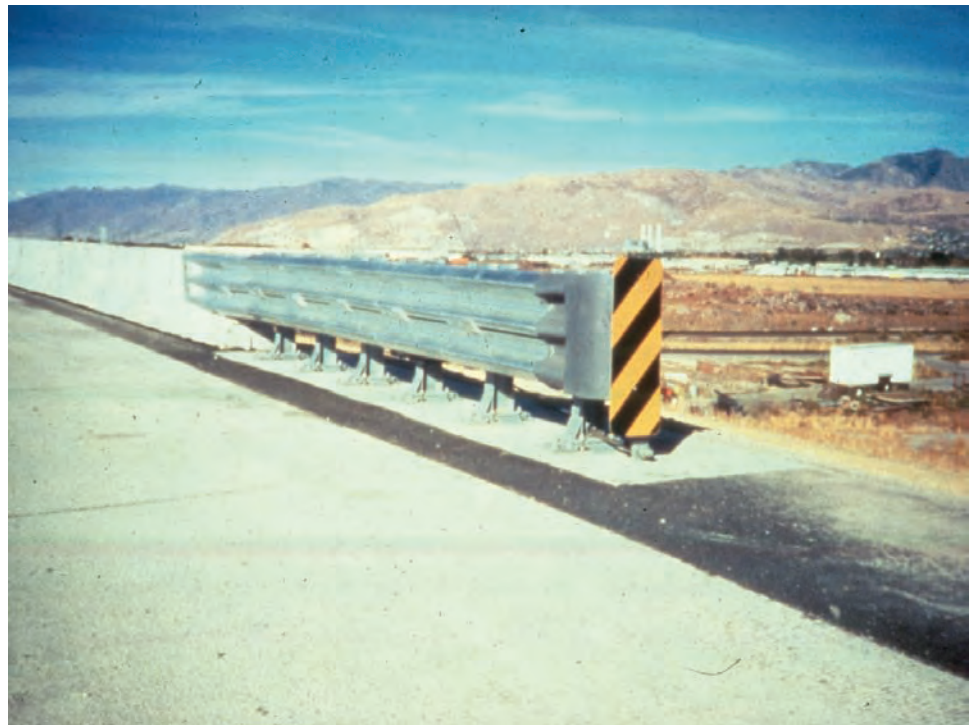
Figure 5.5.1 Bridge Safety Feature
