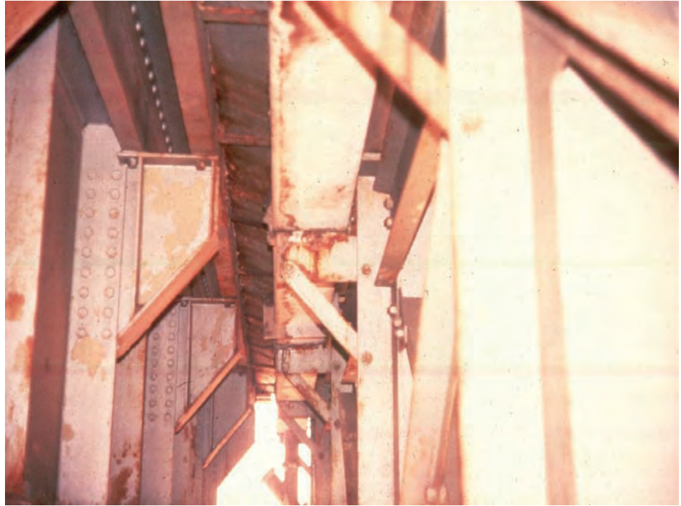
Figure 5.4.5 Supported Finger Plate Joint
