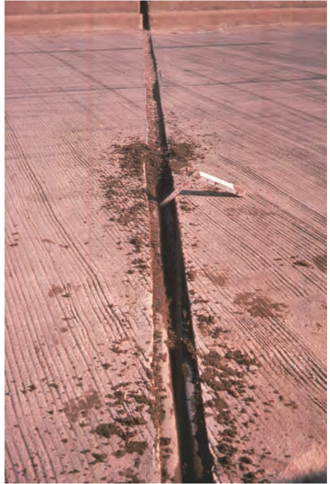
Figure 5.4.16 Dirt in a Compression Seal Joint
