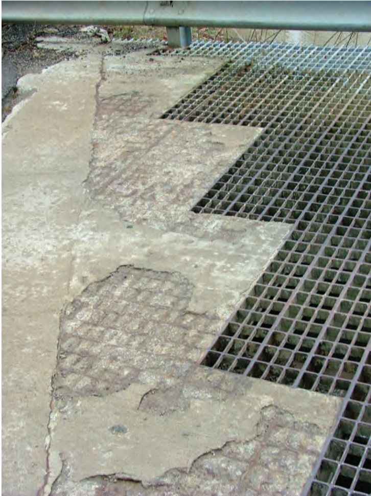
Figure 5.3.5 Filled and Un-filled Steel Grid Deck
