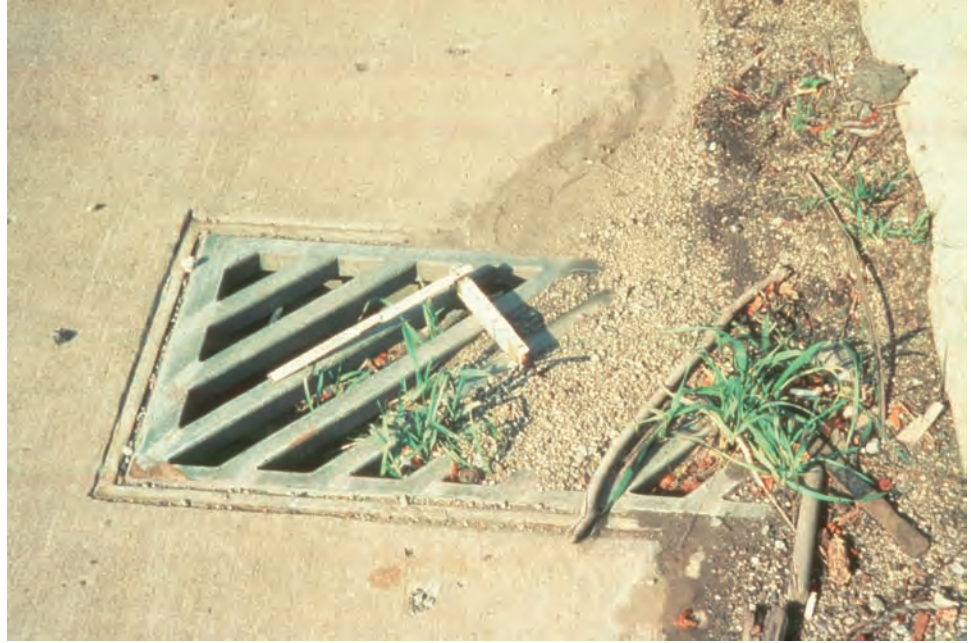
Figure 5.4.13 Bridge Deck Drain
