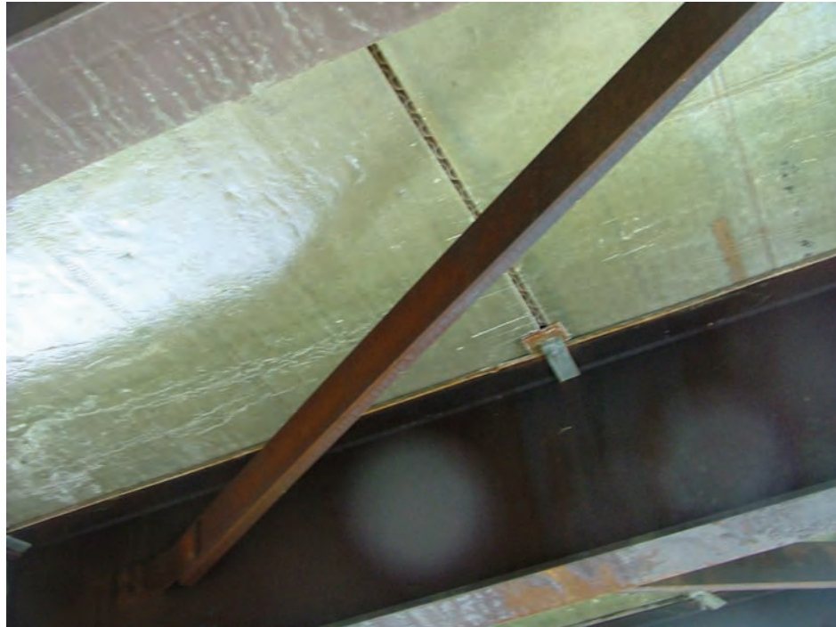
Figure 5.2.3 Fiber Reinforced Polymer (FRP) Deck
