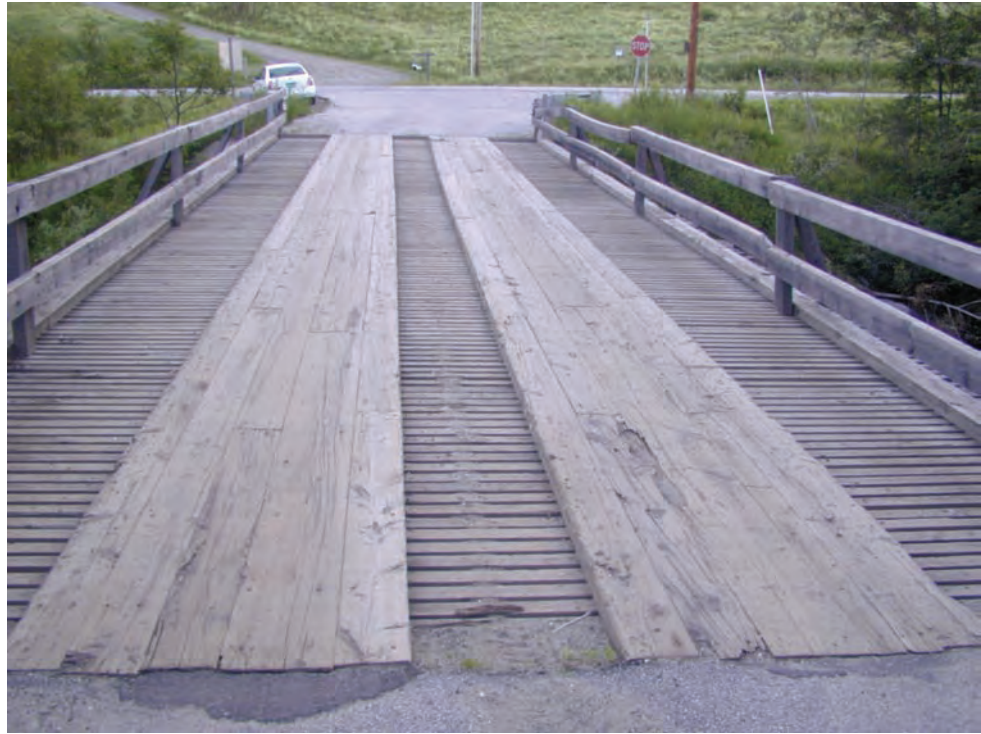
Figure 5.1.6 Timber Wearing Surface on a Timber Deck
