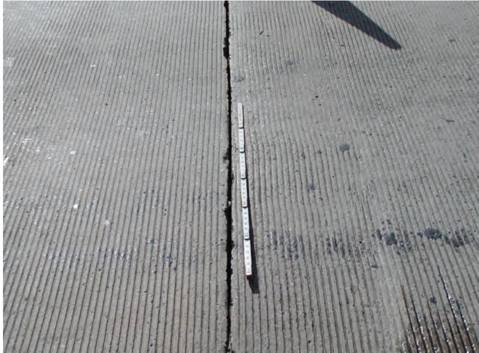
Figure 5.4.1 Formed Joint
