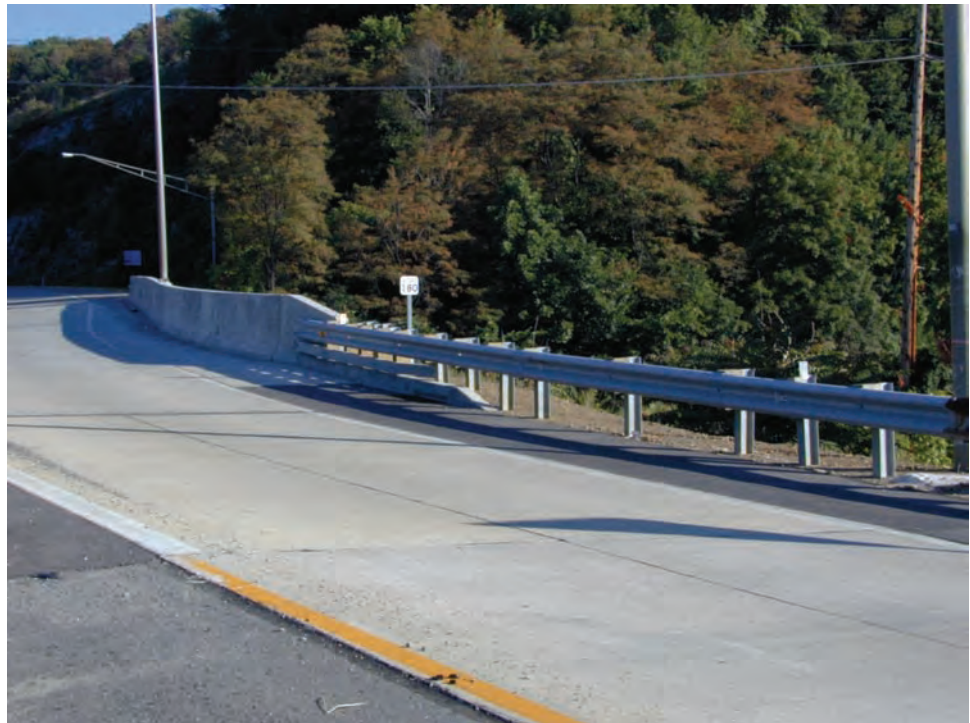
Figure 5.5.7 Approach Guardrail System
