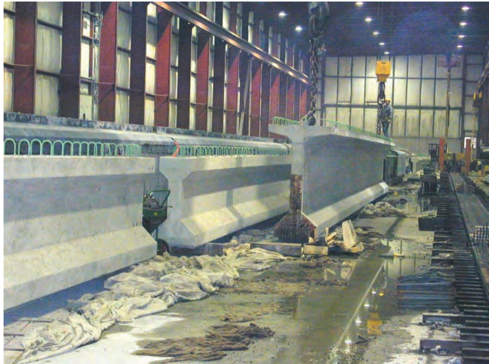
Figure 5.2.7 Prestressed Concrete Beams with Shear Connectors Protruding
