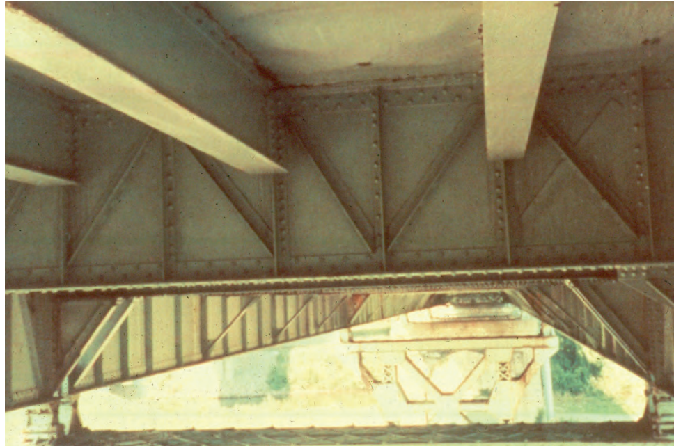
Figure 5.3.2 Underside View of Buckle Plate Deck
