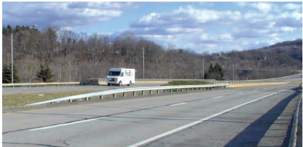
Figure 5.5.3 Bridge Railing, Transition, Approach Guardrail and End Treatment (Turn down end treatment no longer acceptable for this roadway type)
