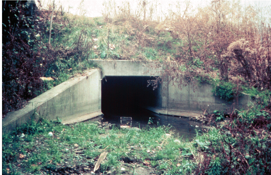
Figure P.3.9 Concrete Box Culvert
