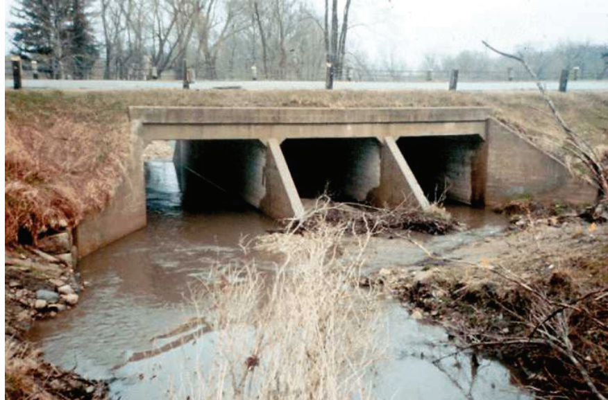
Figure P.3.11 Frame Culvert
