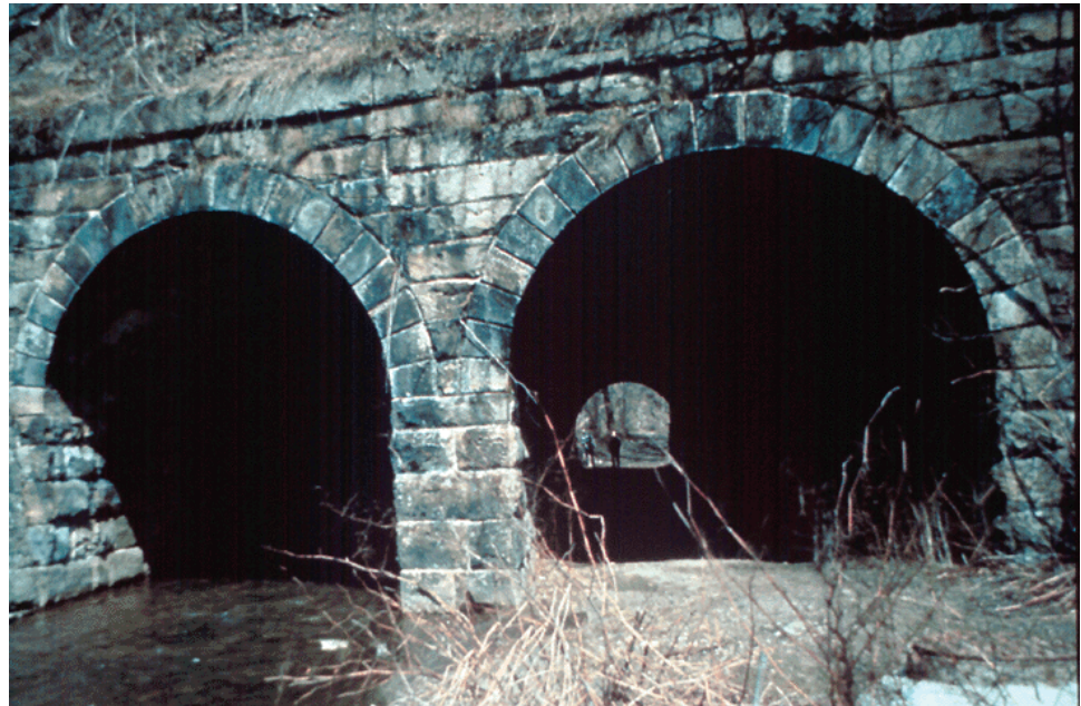
Figure P.3.13 Typical Stone Masonry Arch Culvert
