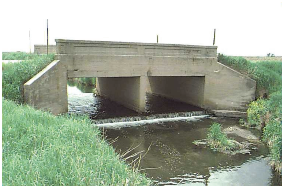
Figure P.3.1 Culvert Structure
