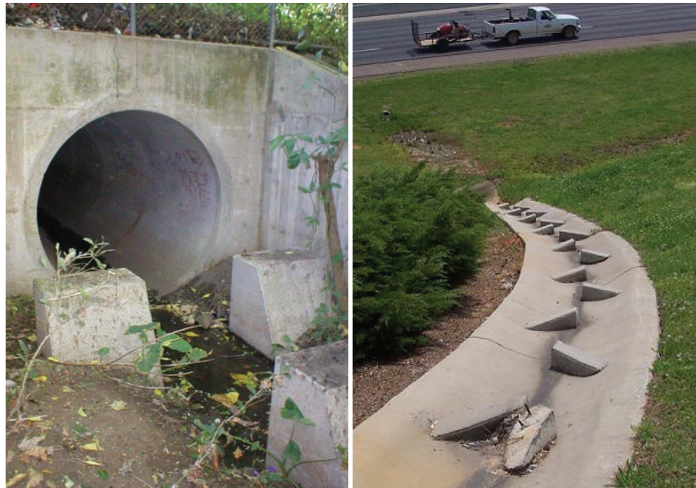
Figure P.3.20 Energy Dissipator
