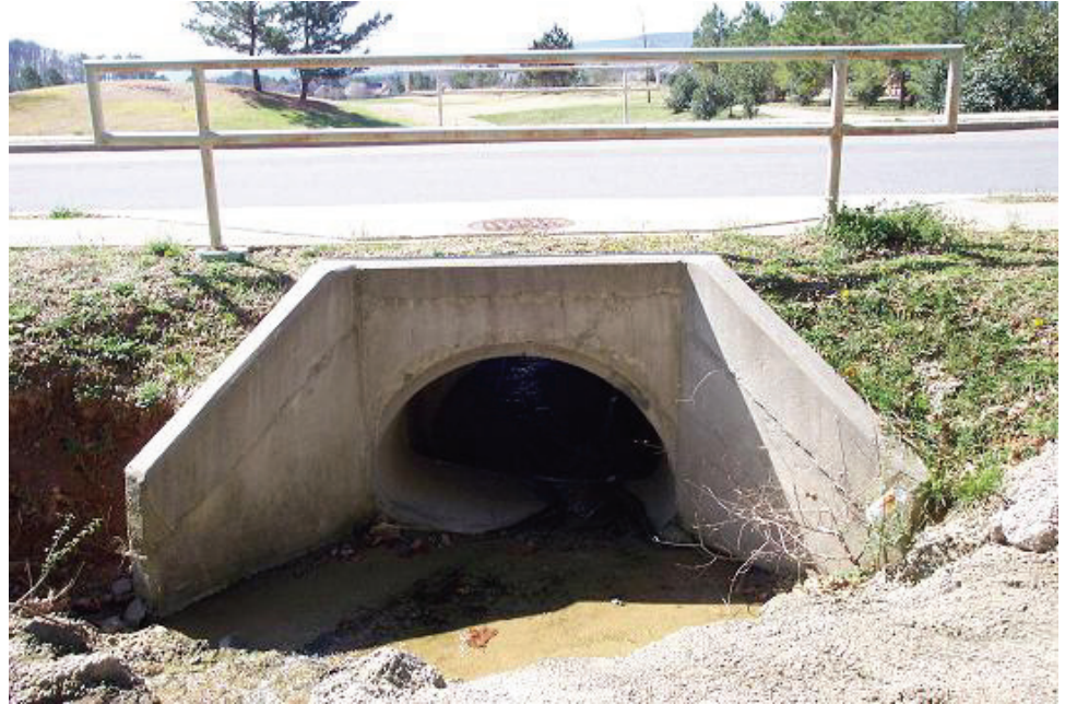
Figure P.3.18 Culvert Headwall
