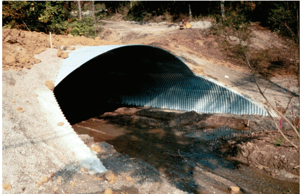
Figure P.3.7 Pipe Arch Culvert
