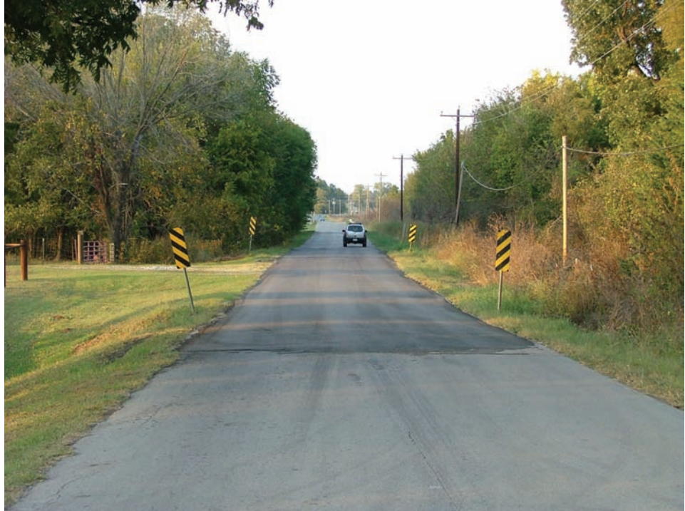
Figure P.3.27 Roadway Over a Culvert
