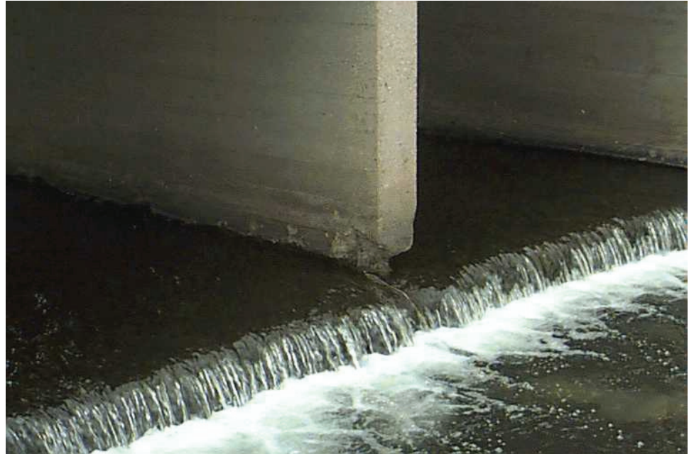
Figure P.3.34 Energy Dissipater
