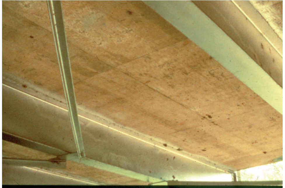
Figure P.1.29 Concrete Deck
