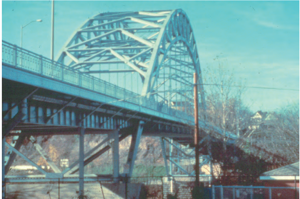
Figure P.1.56 Through Arch Bridge
