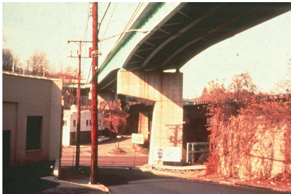
Figure P.1.4 Unusual Concrete Shapes
