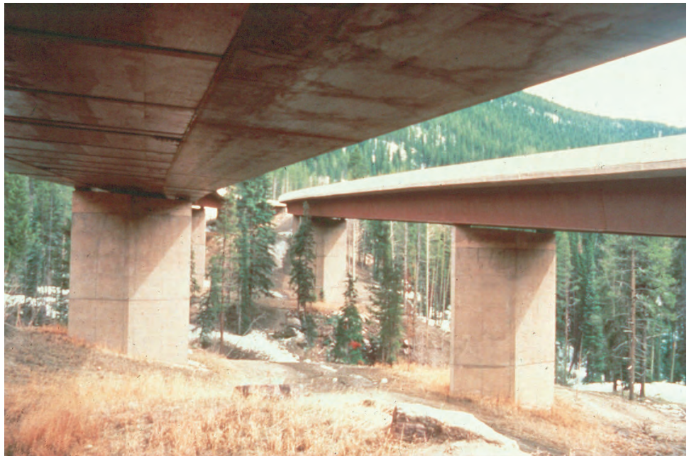
Figure P.1.52 Steel Box Girder Bridge
