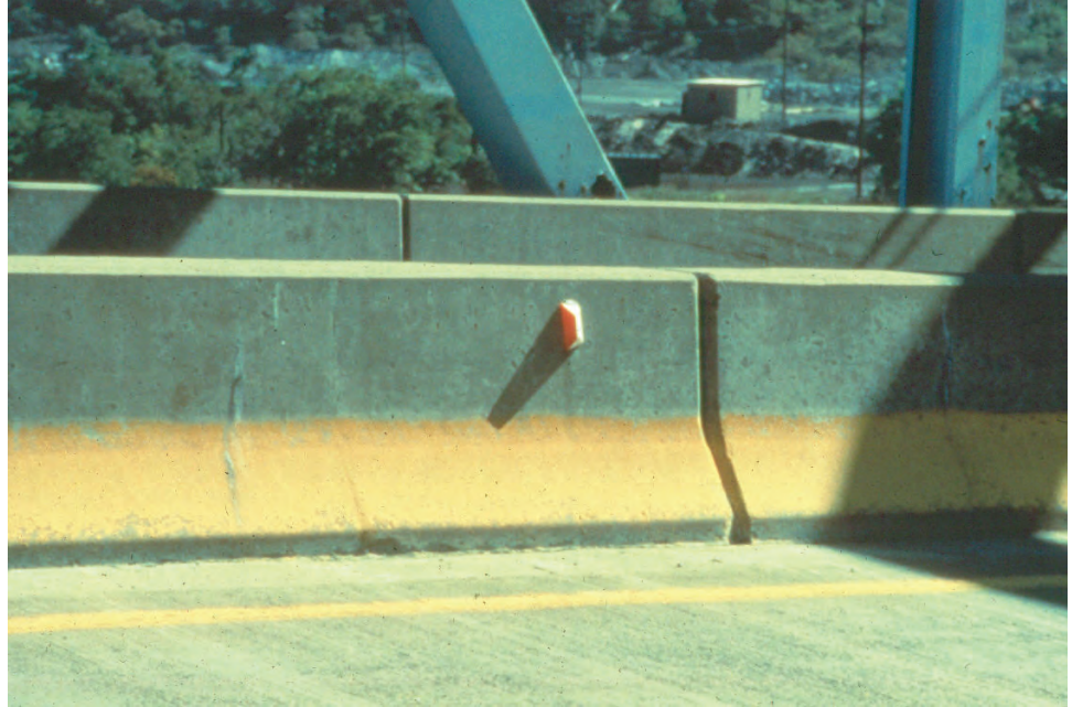
Figure P.1.36 New Jersey Barrier
