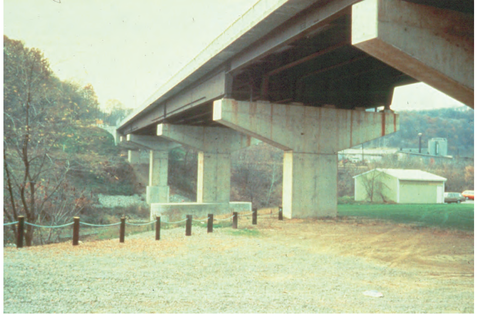
Figure P.1.74 Cantilever or Hammerhead Pier
