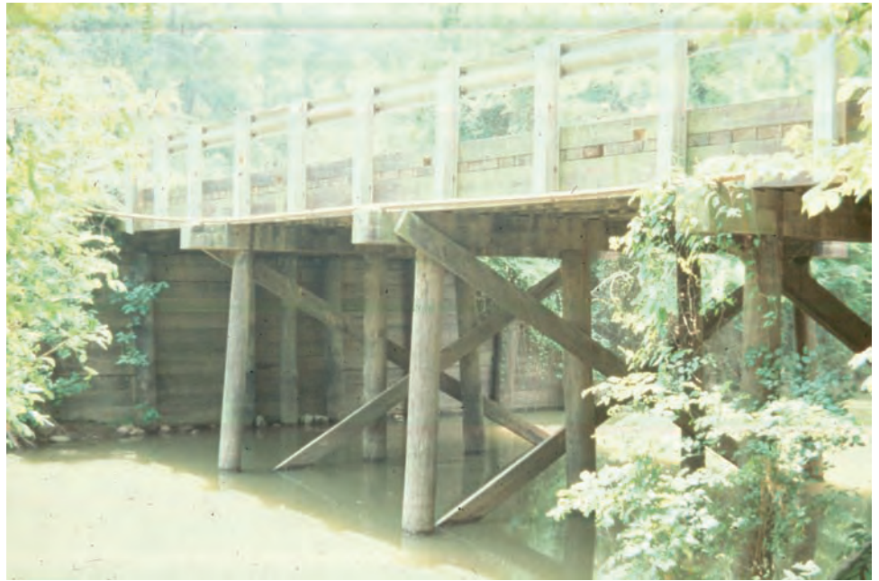
Figure P.1.46 Timber Beam Bridge
