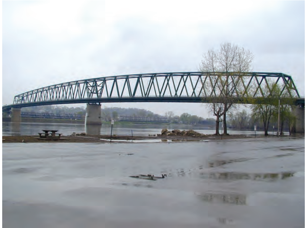
Figure P.1.54 Through Truss Bridge
