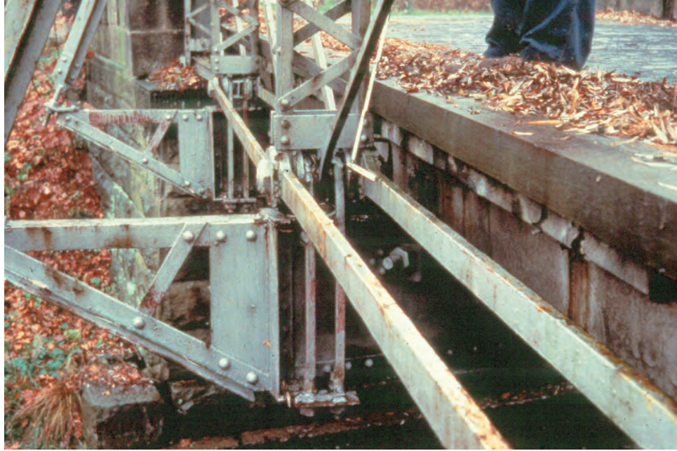
Figure P.1.18 Pin-Connected Truss Members
