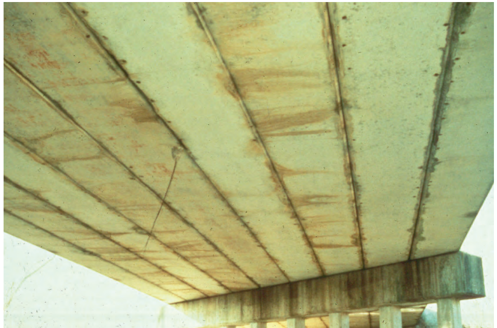
Figure P.1.51 Adjacent Box Beam Bridge
