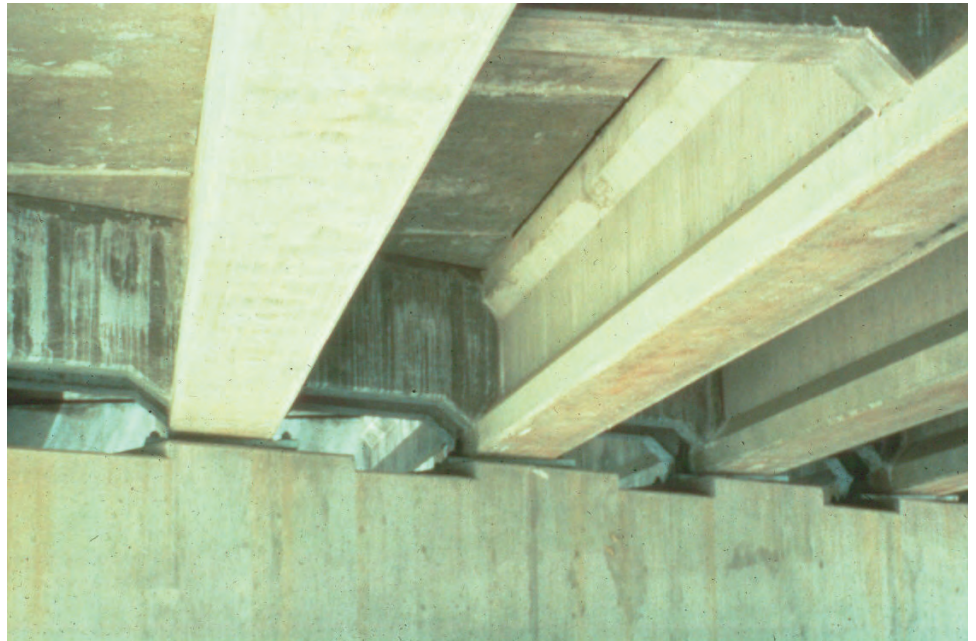
Figure P.1.47 Prestressed Concrete Multi-Girder Bridge
