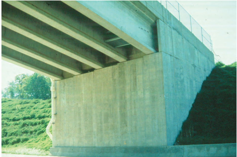
Figure P.1.65 Concrete Abutment
