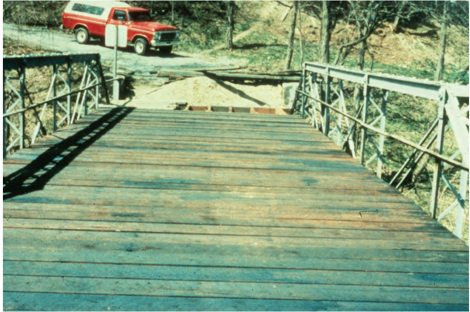
Figure P.1.28 Plank Deck
