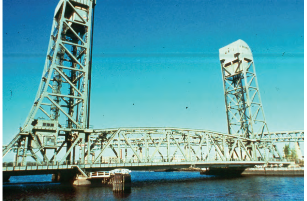
Figure P.1.61 Lift Bridge
