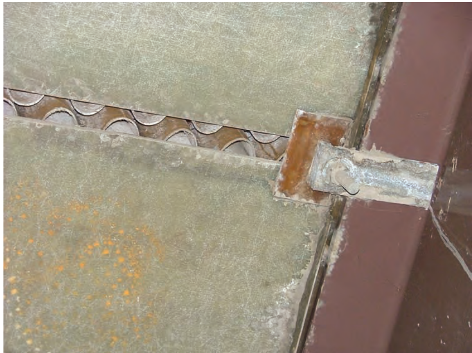
Figure P.1.31 Fiber Reinforced Polymer (FRP) Deck
