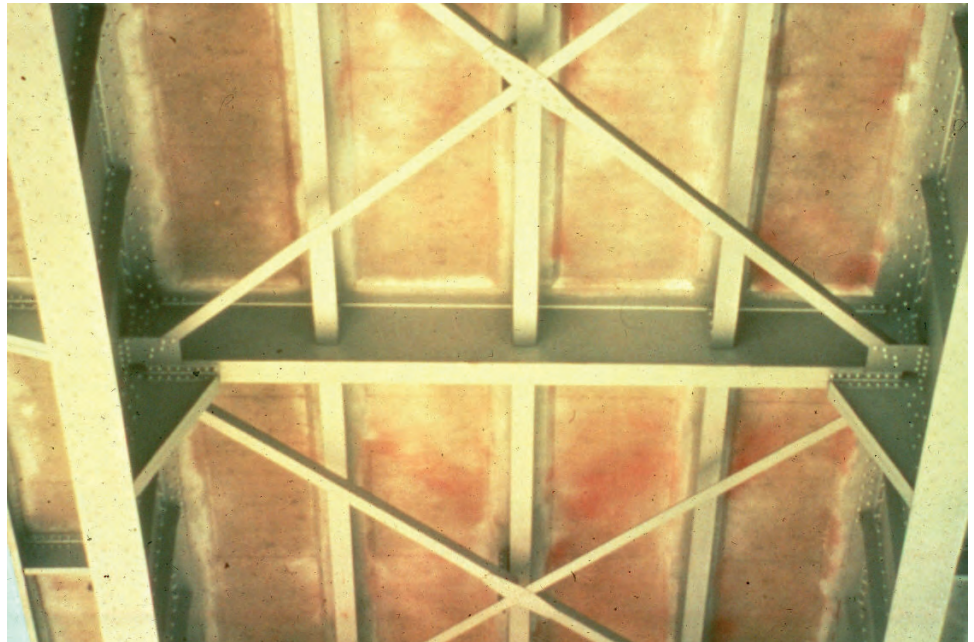
Figure P.1.39 Floor System
