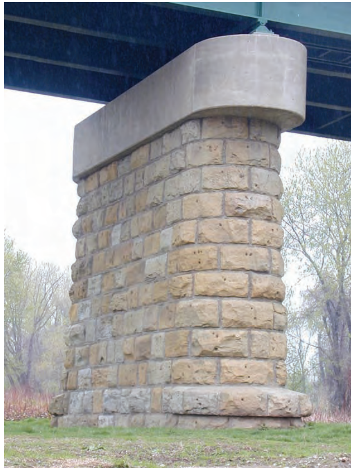
Figure P.1.71 Solid Shaft Pier
