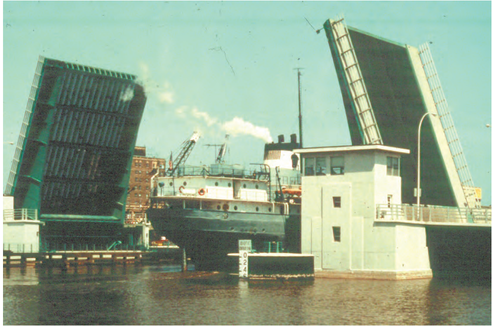
Figure P.1.59 Bascule Bridge
