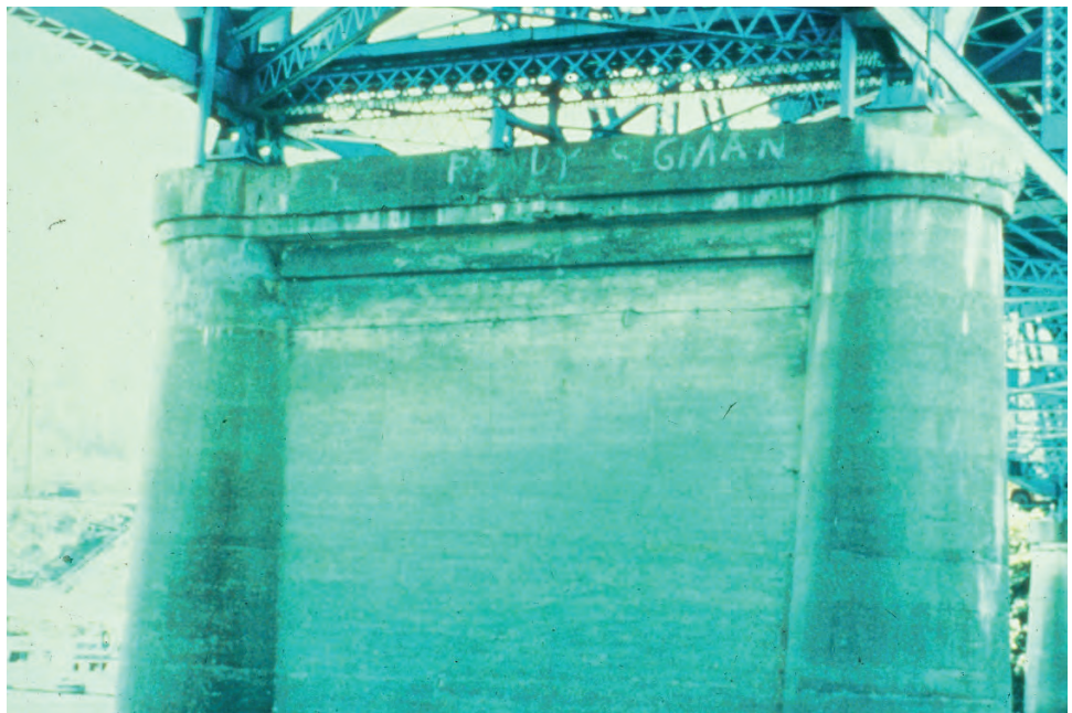
Figure P.1.73 Column Pier with Web Wall
