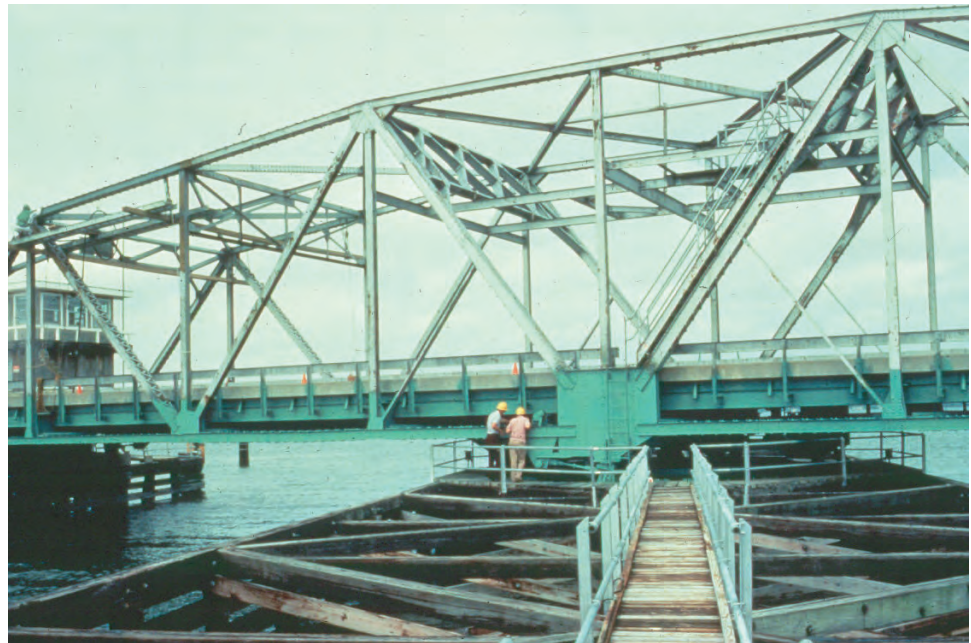
Figure P.1.60 Swing Bridge
