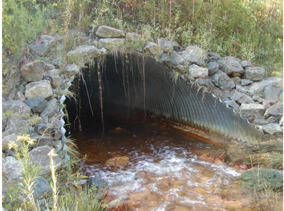
Figure P.1.63 Culvert
