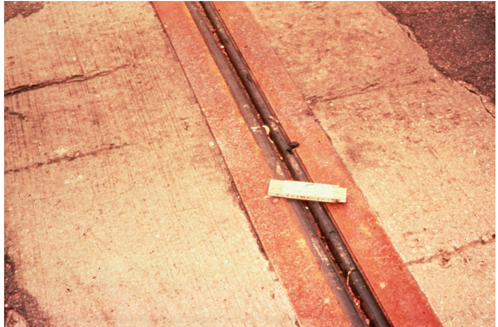
Figure P.1.34 Top View of an Armored Compression Seal in Place
