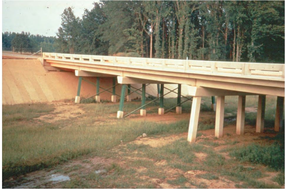
Figure P.1.76 Pile Bent
