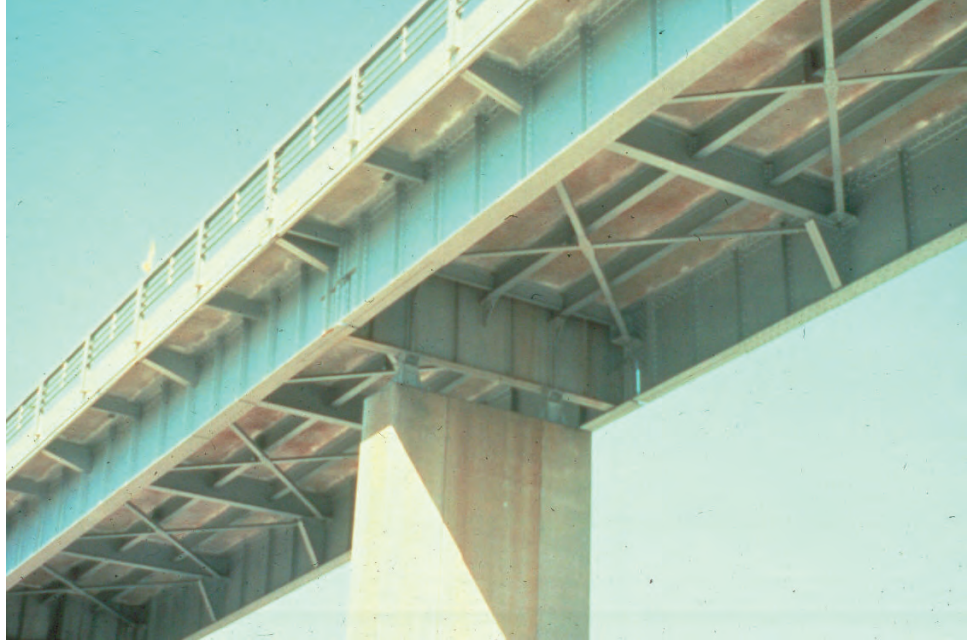
Figure P.1.48 Girder Floorbeam Stringer Bridge
