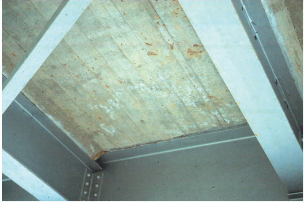
Figure P.1.25 Underside View of a Bridge Deck
