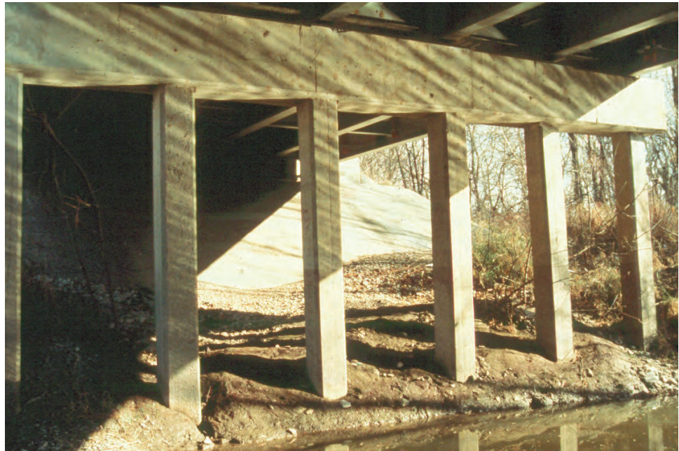
Figure P.1.8 Concrete Pile Bent
