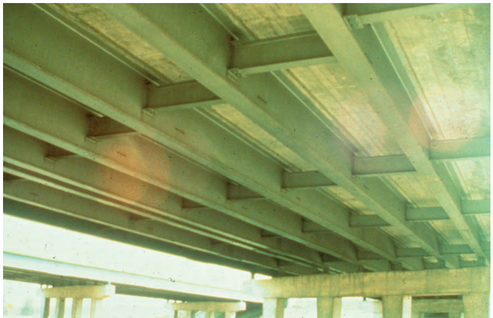
Figure P.1.41 Diaphragms
