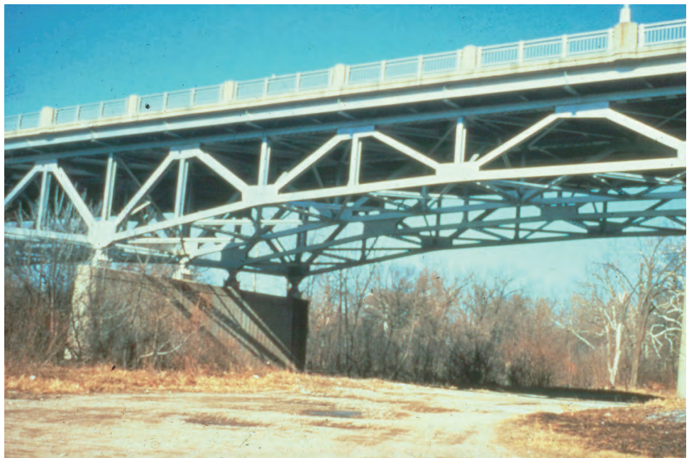
Figure P.1.53 Deck Truss Bridge
