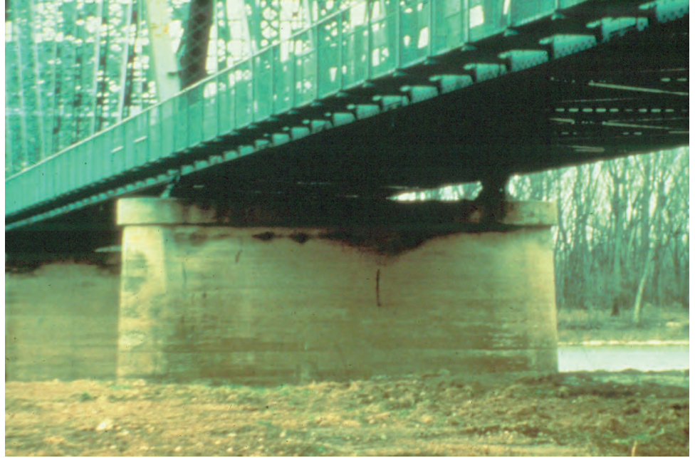
Figure P.1.70 Solid Shaft Pier
