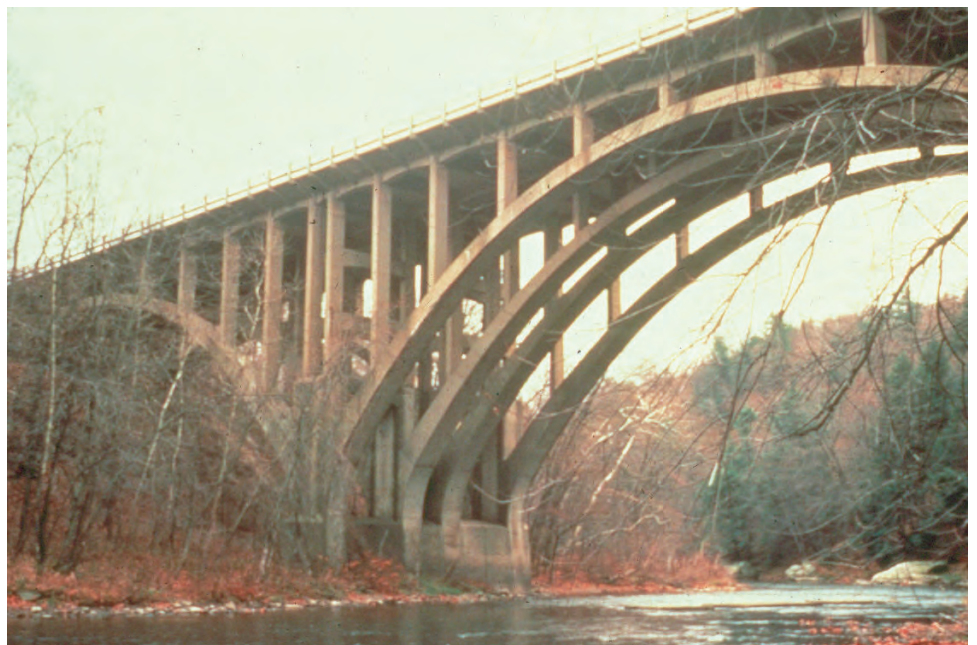
Figure P.1.55 Concrete Deck Arch Bridge
