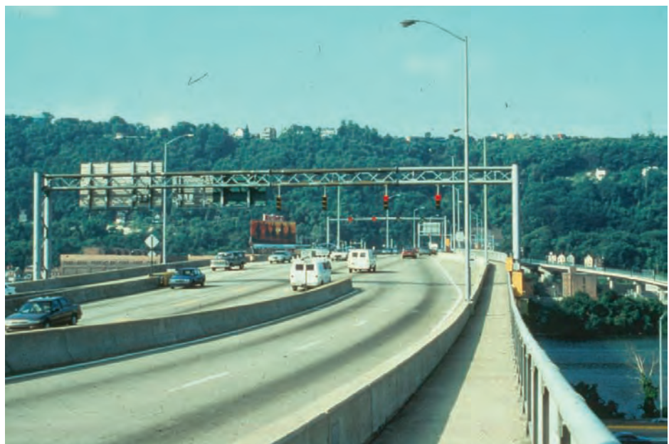
Figure P.1.38 Bridge Lighting
