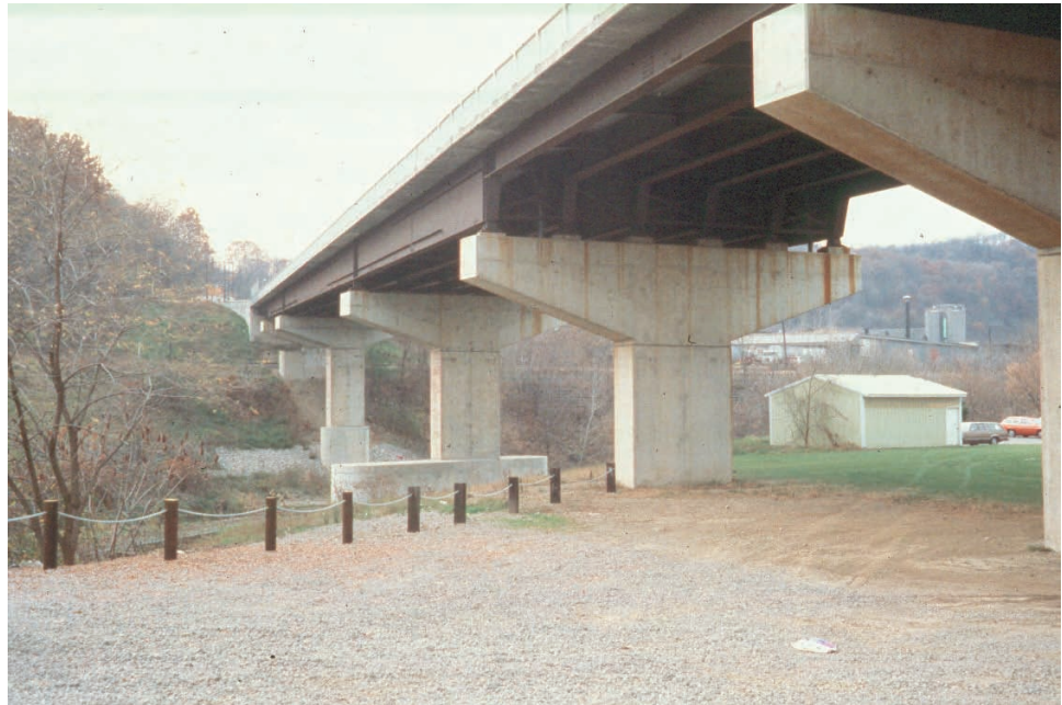
Figure 10.2.7 Cantilever Pier
