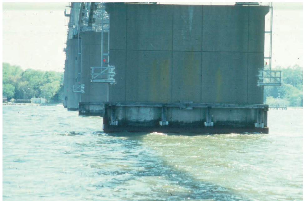
Figure 10.2.54 Steel Fender
