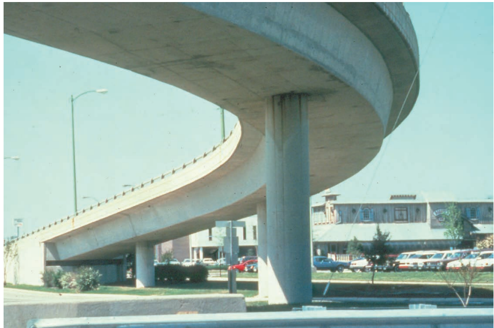
Figure 10.2.3 Column Pier
