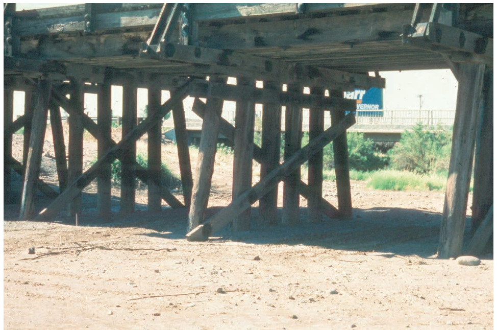
Figure 10.2.16 Timber Pile Bent
