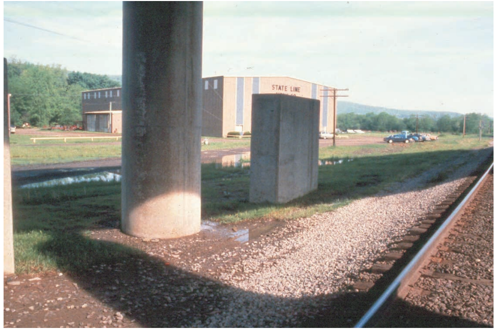
Figure 10.2.26 Concrete Block Dolphin
