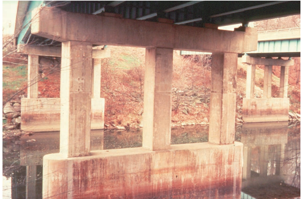
Figure 10.2.25 Collision Wall
