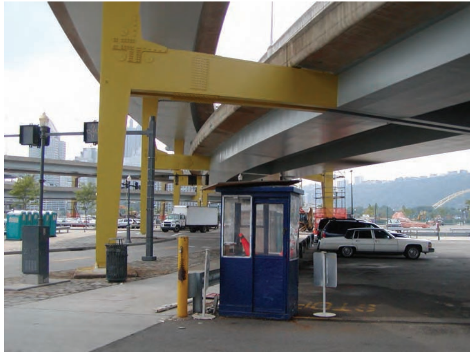
Figure 10.2.52 Fracture Critical Steel Bent
