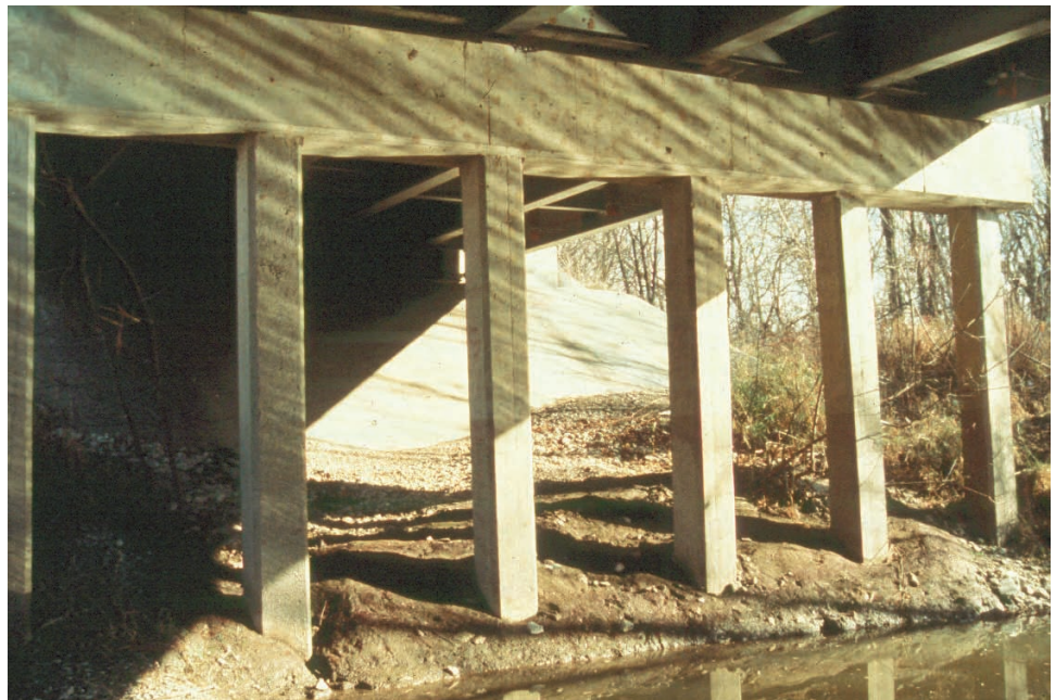
Figure 10.2.9 Concrete Pile Bent
