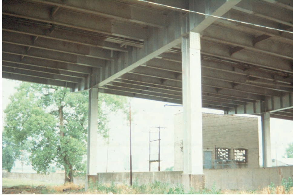
Figure 10.2.43 Steel Column Bent with Cantilever
