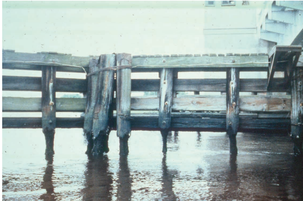
Figure 10.2.55 Timber Fender System
