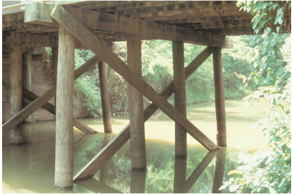
Figure 10.2.46 Timber Bent Columns in Water
