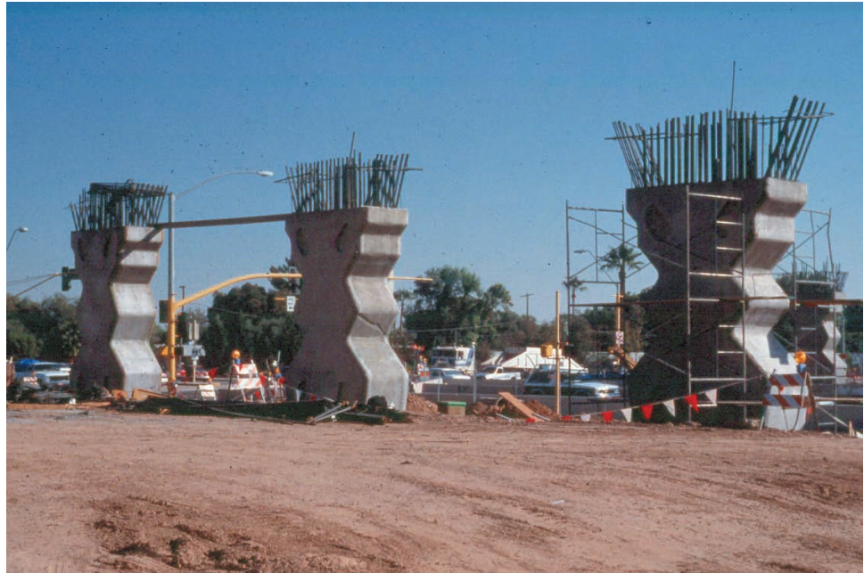
Figure 10.2.13 Reinforced Concrete Piers under Construction
