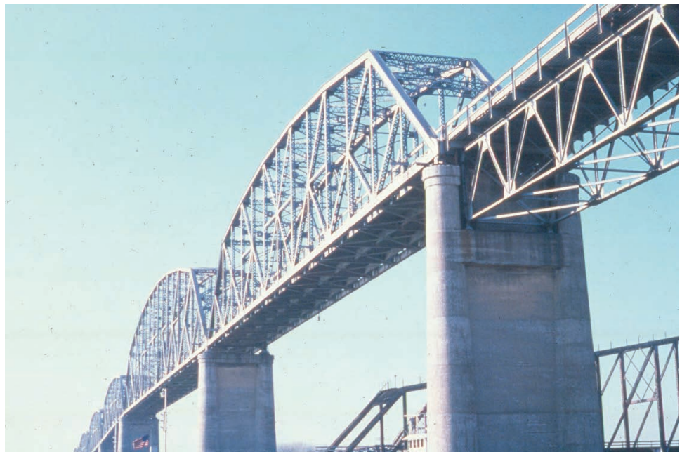
Figure 10.2.5 Column Pier with Web Wall
