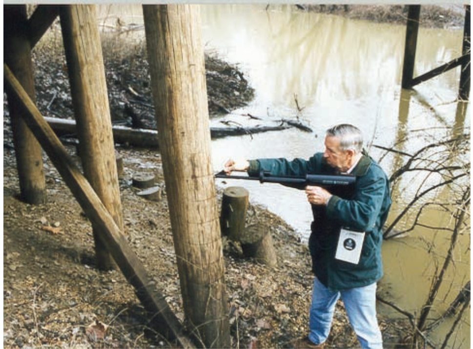
Figure 10.2.44 Drilling a Timber Bent Column for a Core Sample
