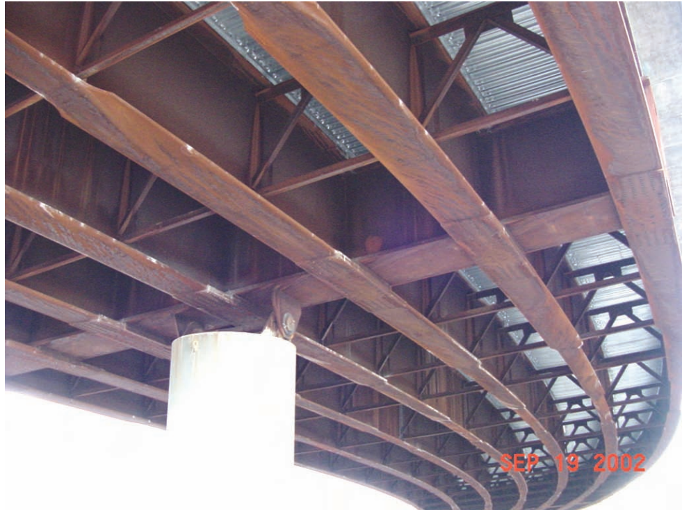
Figure 10.2.10 Integral Pier Cap
