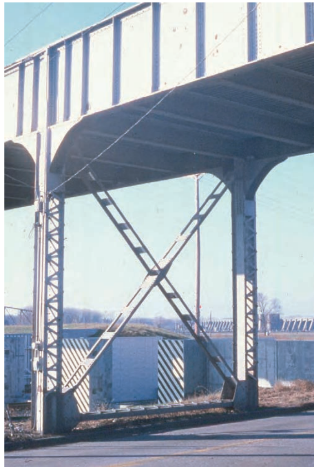
Figure 10.2.41 Corrosion and Debris at Steel Pile Bent
