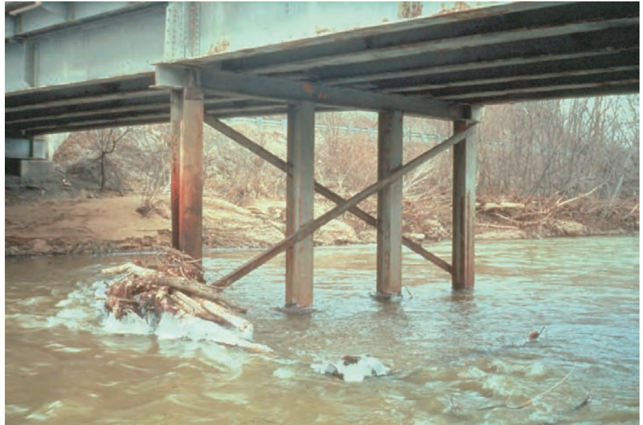
Figure 10.2.41 Corrosion and Debris at Steel Pile Bent
