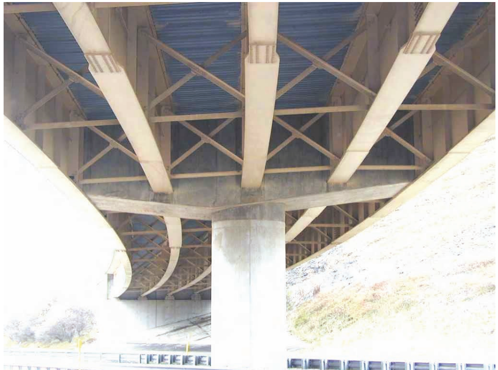
Figure 10.2.12 Integral Pier and Pier Cap
