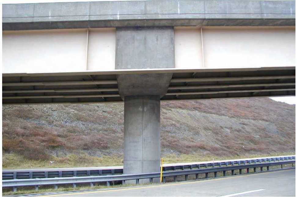
Figure 10.2.11 Integral Pier and Pier Cap
