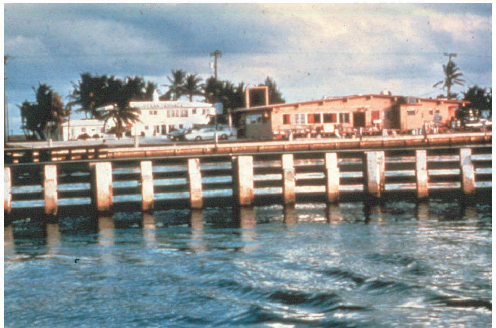
Figure 10.2.29 Fender System
