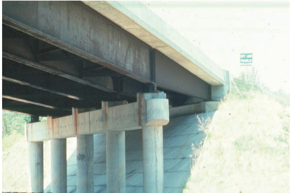
Figure 10.2.8 Column Bent or Open Bent
