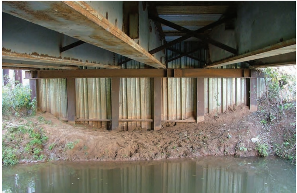
Figure 10.1.16 Steel Abutment
