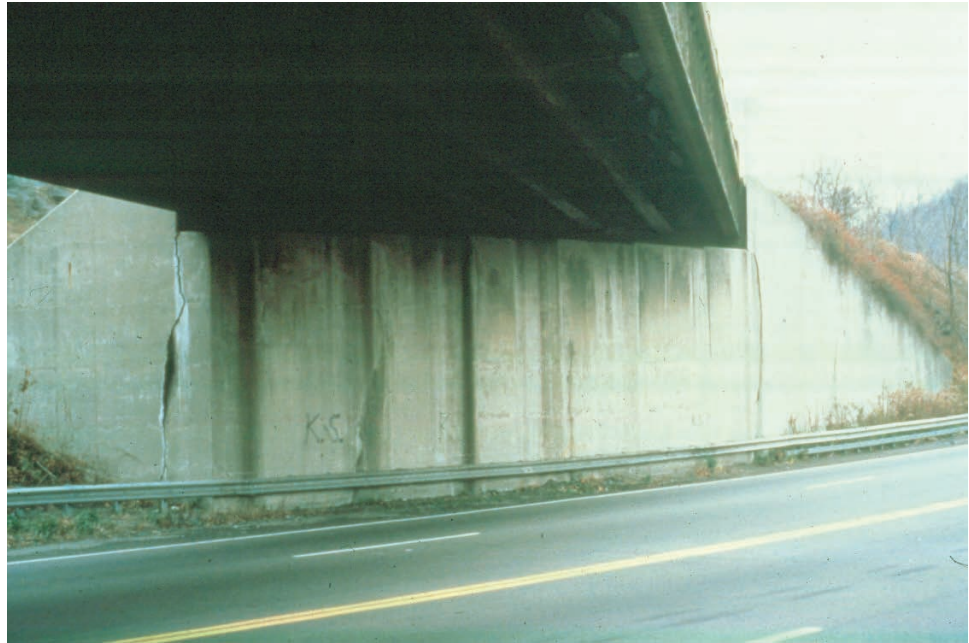
Figure 10.1.53 Settlement Cracks at Integral Concrete Wingwalls
