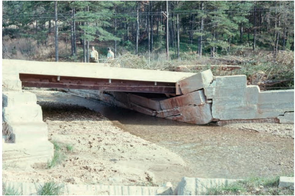
Figure 10.1.39 Abutment with Undermining due to Scour
