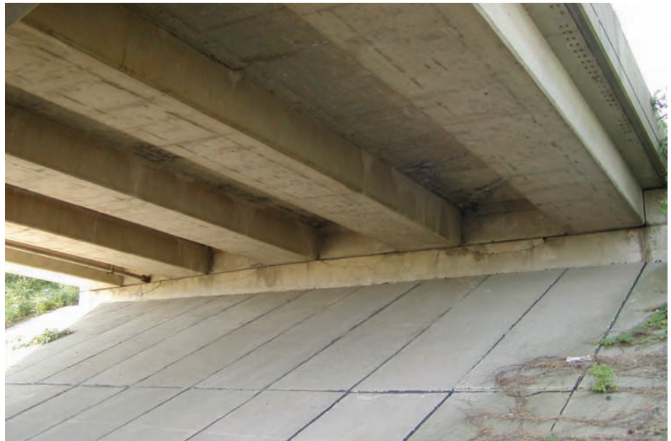
Figure 10.1.4 Stub Abutment
