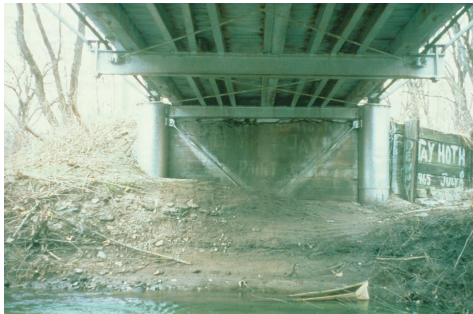
Figure 10.1.35 Steel Abutment
