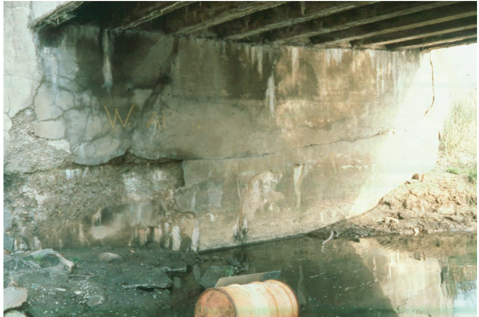
Figure 10.1.12 Plain Unreinforced Concrete Gravity Abutment
