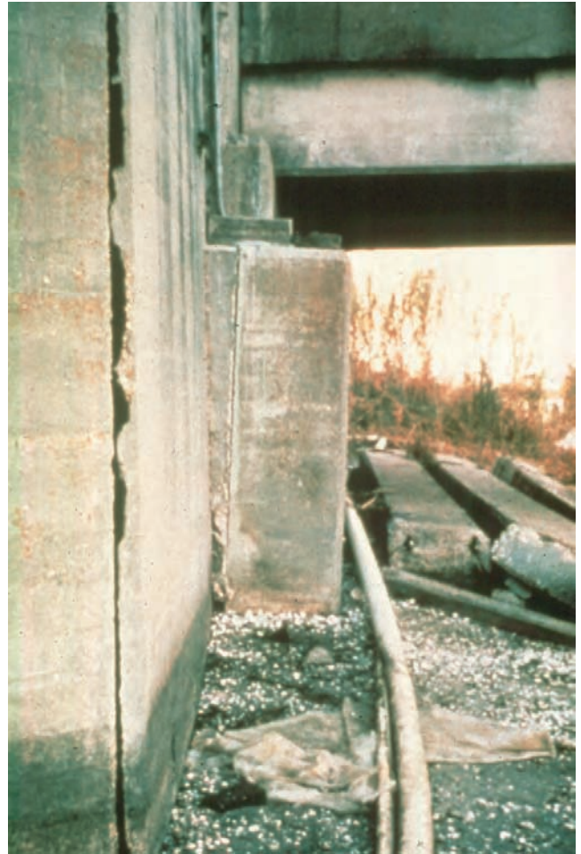
Figure 10.1.30 Rotational Movement at Abutment
