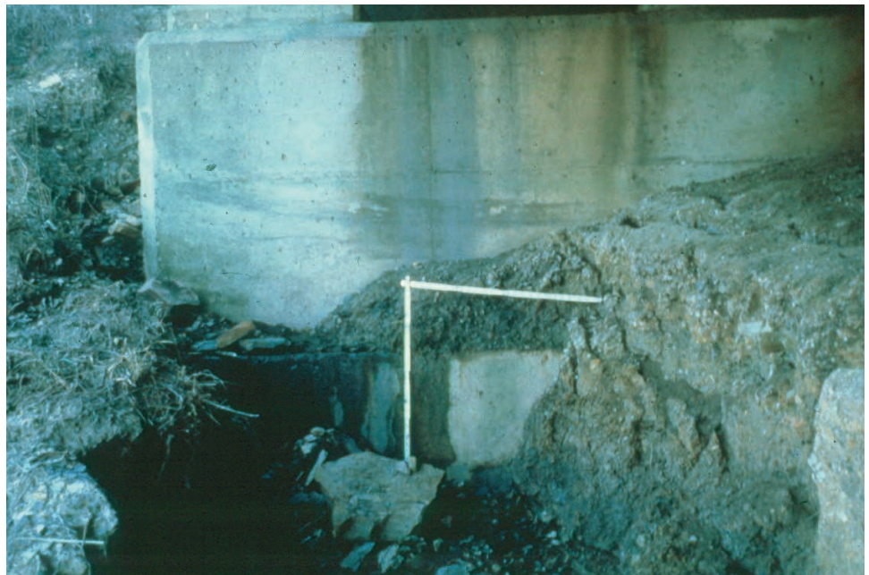
Figure 10.1.28 Erosion at Abutment Exposing Footing
