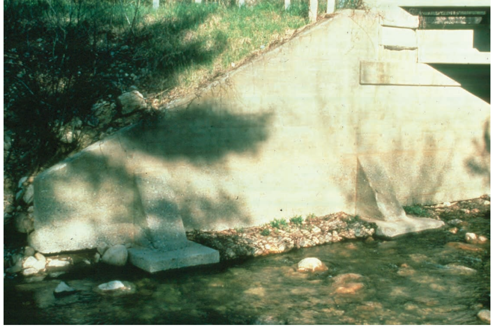
Figure 10.1.51 Scour and Possible Undermining of Concrete Wingwall
