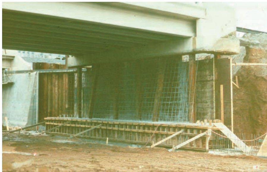
Figure 10.1.21 Stub Abutment on Piles with Piles Exposed
