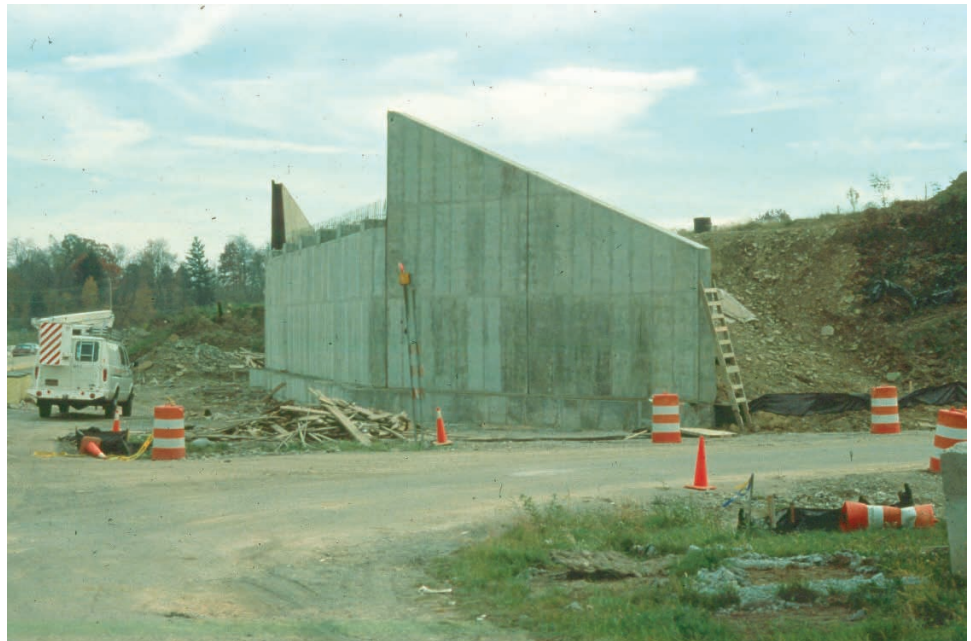
Figure 10.1.13 Reinforced Concrete Cantilever Abutment
