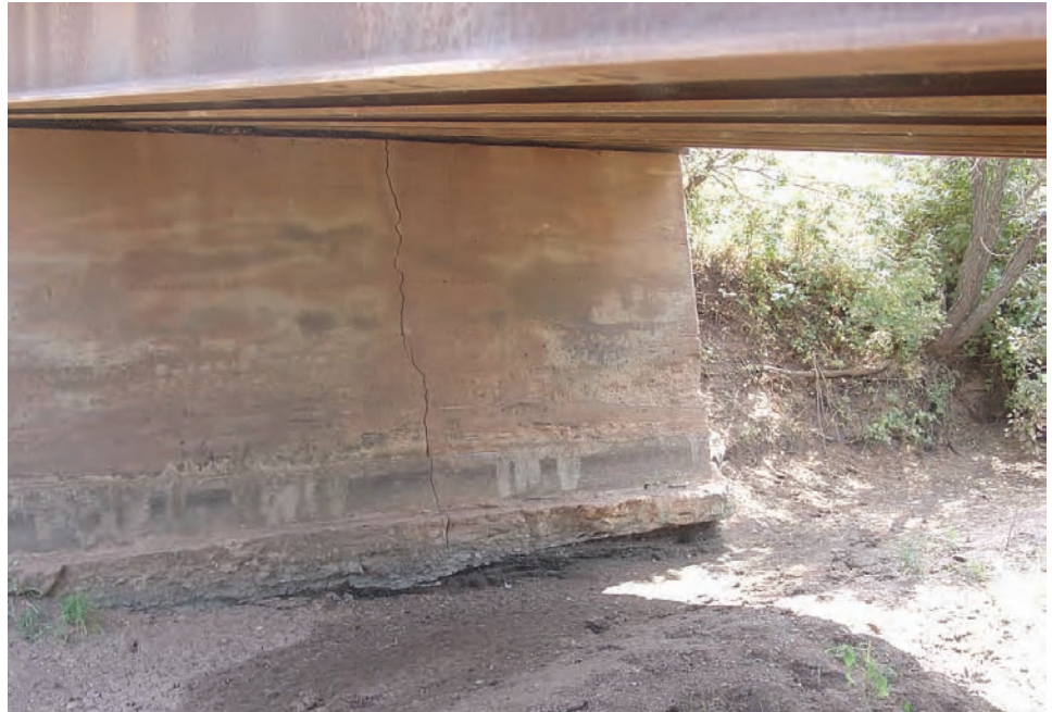
Figure 10.1.24 Crack in Abutment due to Settlement
