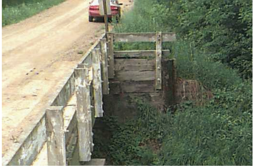
Figure 10.1.55 Timber Wingwall
