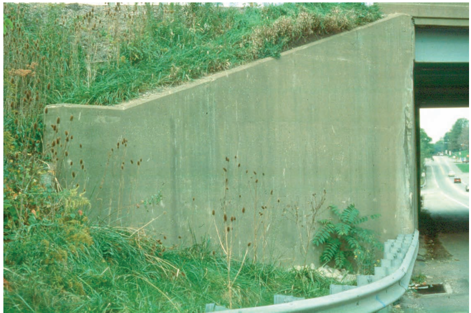
Figure 10.1.41 Typical Wingwall
