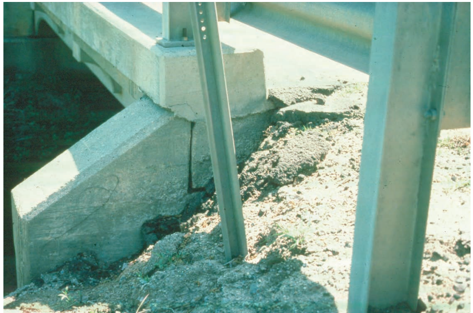
Figure 10.1.52 Roadway Shoulder Erosion Behind Wingwall
