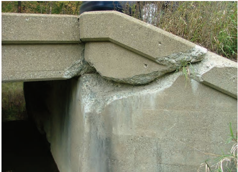
Figure 10.1.50 Deteriorated Concrete Wingwall
