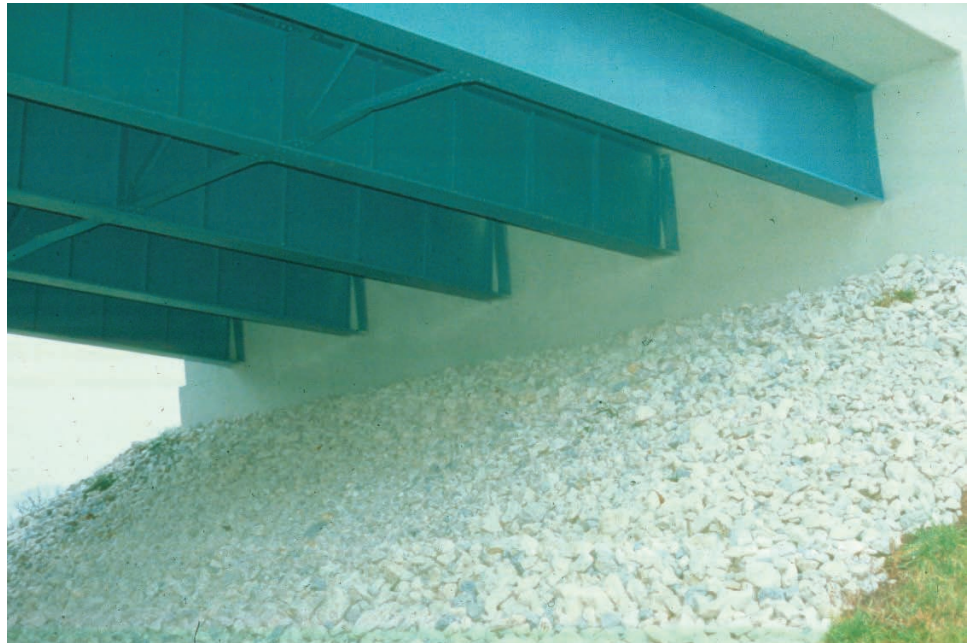
Figure 10.1.7 Integral Abutment
