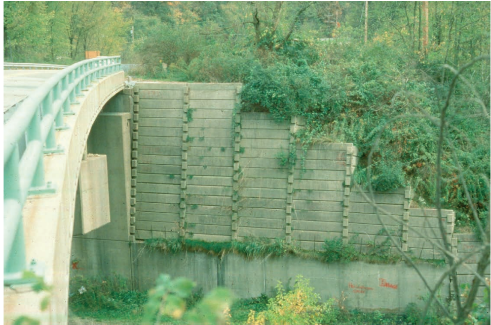
Figure 10.1.42 Straight Wingwall
