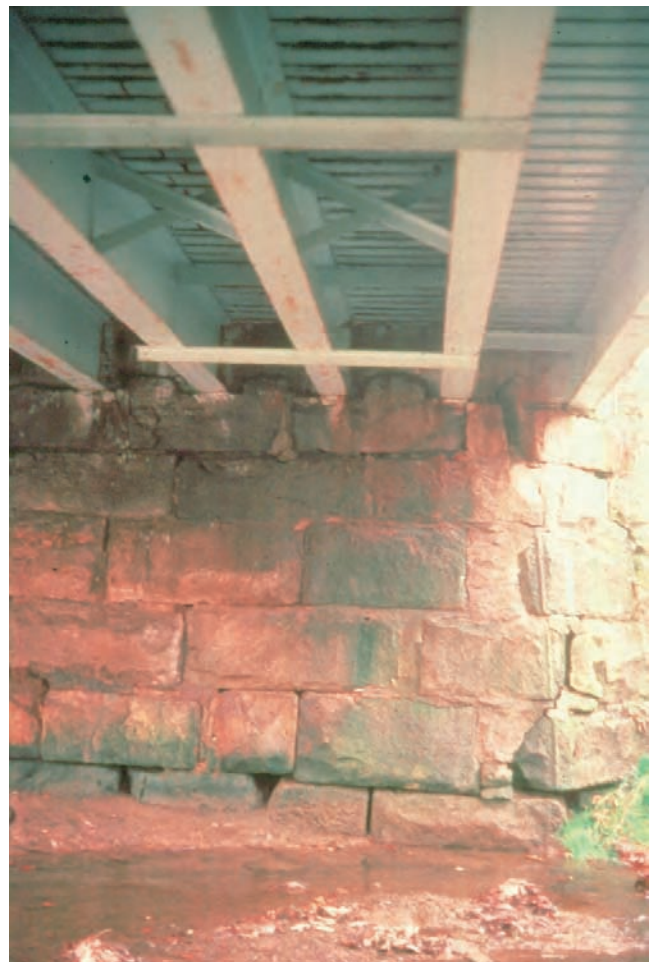
Figure 10.1.34 Deteriorated Stone Masonry Abutment
