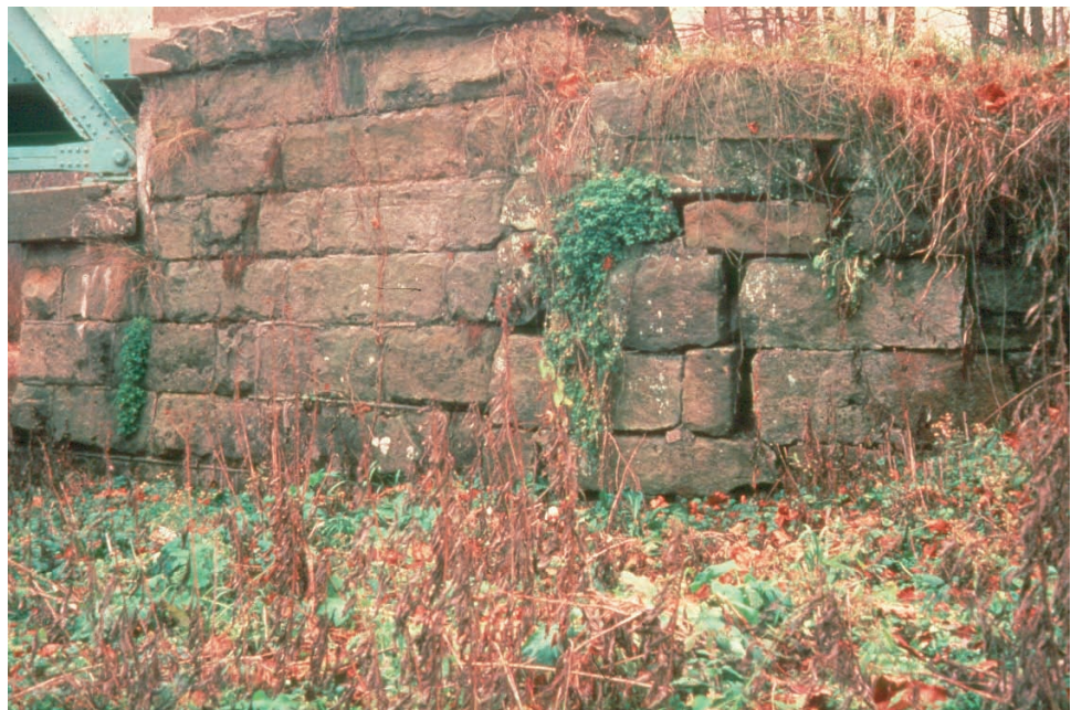
Figure 10.1.54 Deteriorating Stone Masonry Wingwall
