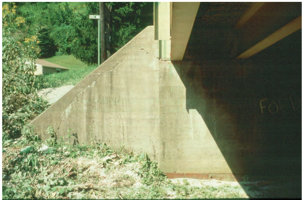
Figure 10.1.43 Flared Wingwall
