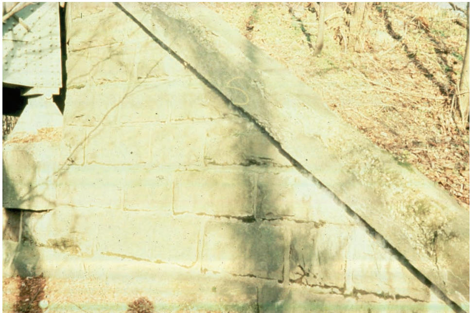
Figure 10.1.47 Masonry Wingwall
