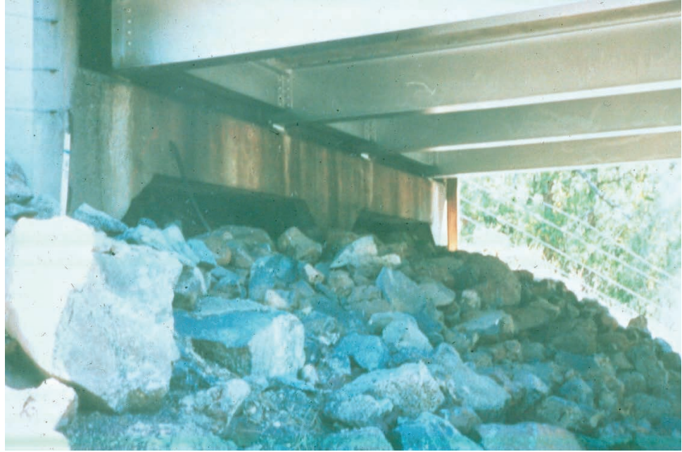
Figure 10.1.5 Open Abutment
