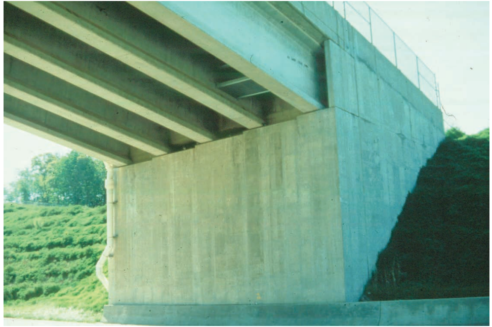
Figure 10.1.3 Full Height Abutment
