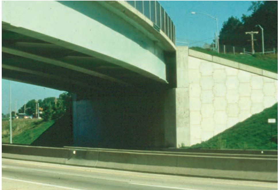
Figure 10.1.46 Independent MSE Wingwall
