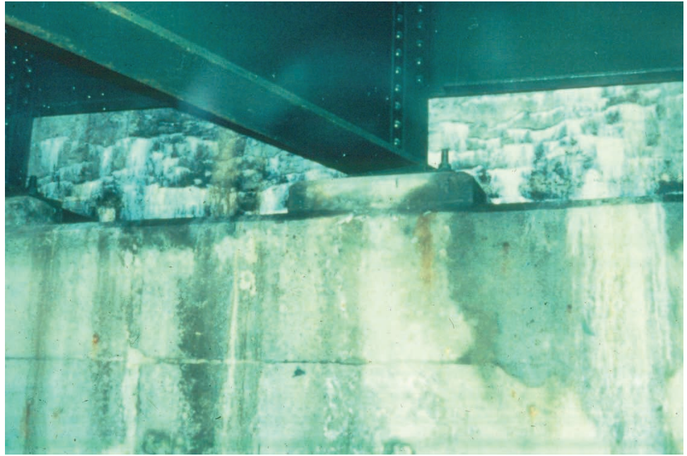
Figure 10.1.33 Deteriorated Concrete in Abutment Backwall
