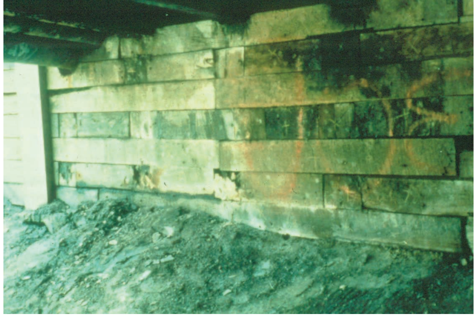
Figure 10.1.37 Decay in Lagging of Timber Crib Abutment
