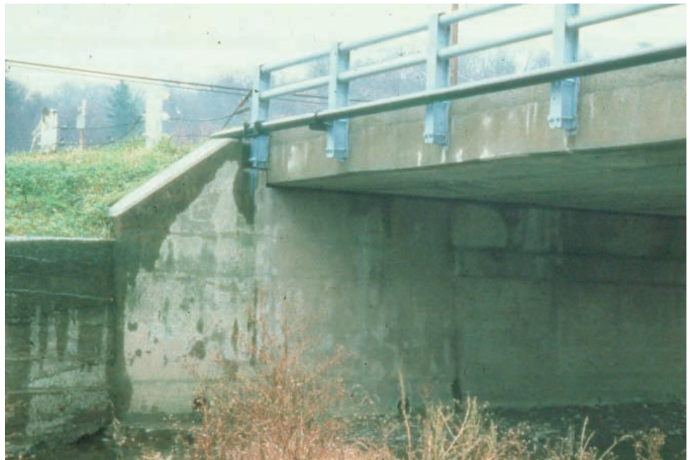
Figure 10.1.45 Integral Wingwall
