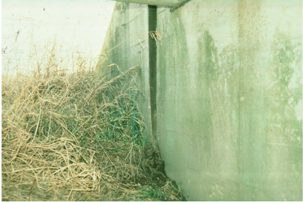
Figure 10.1.49 Rotational Movement at Concrete Wingwall
