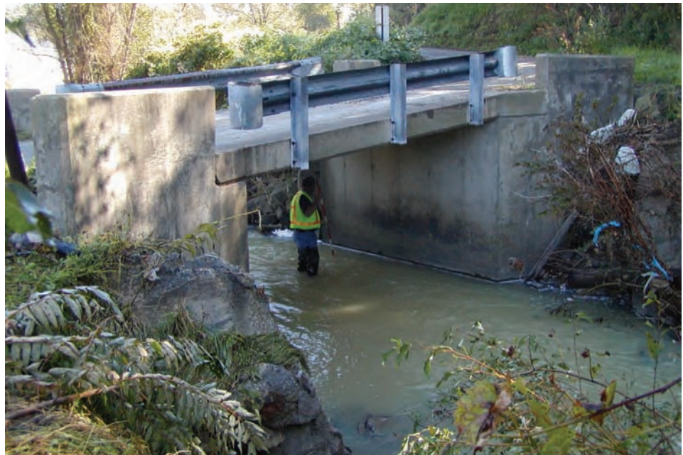
Figure 10.1.40 Inspector Checking for Scour
