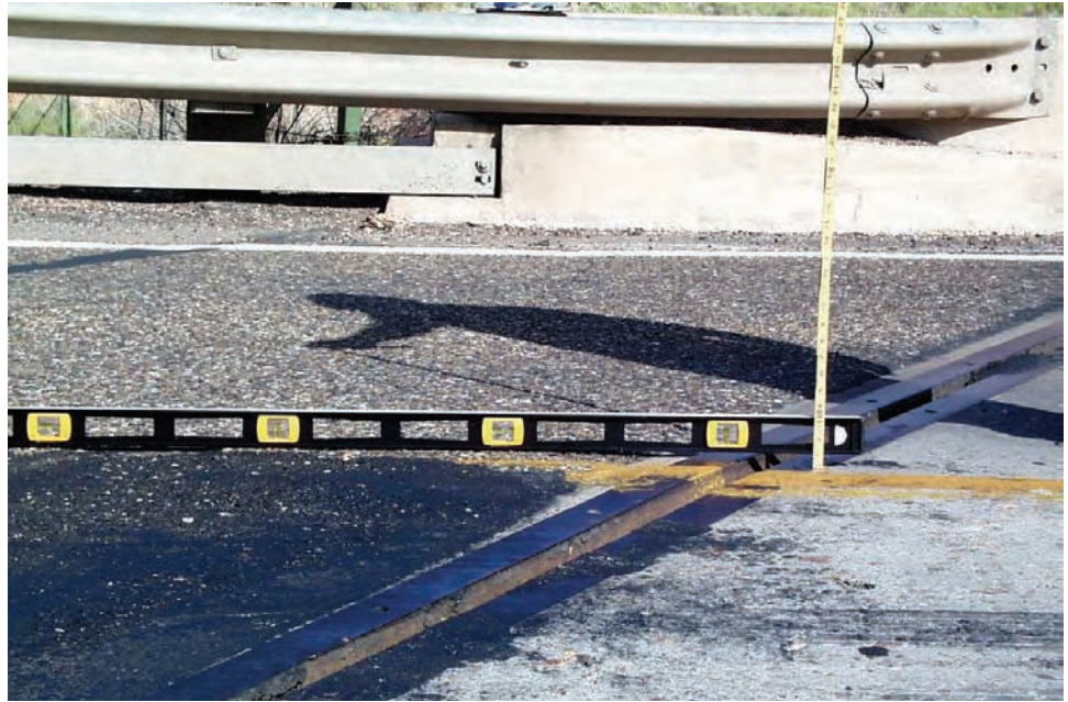
Figure 10.1.27 Depressed Approach Slab due to Rotating Abutment
