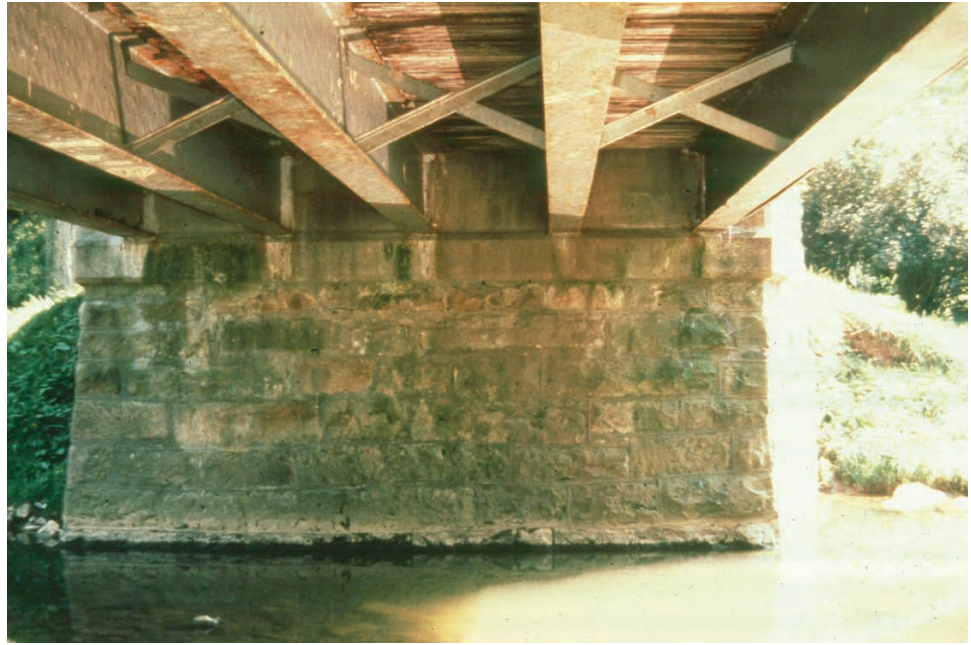
Figure 10.1.14 Stone Masonry Gravity Abutment
