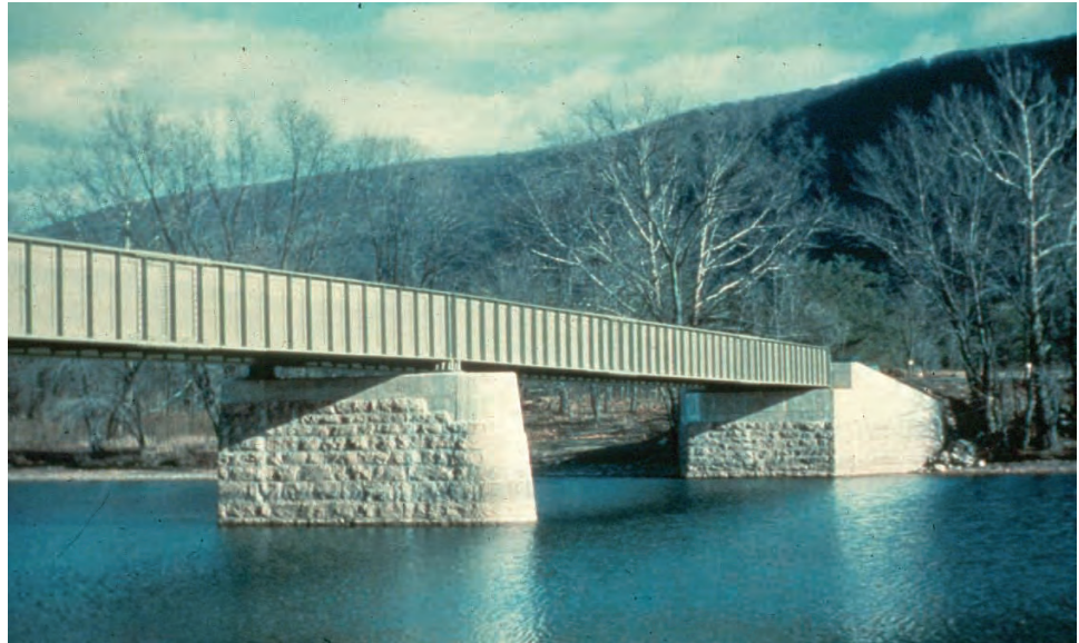
Figure 11.3.20 Solid Shaft Pier
