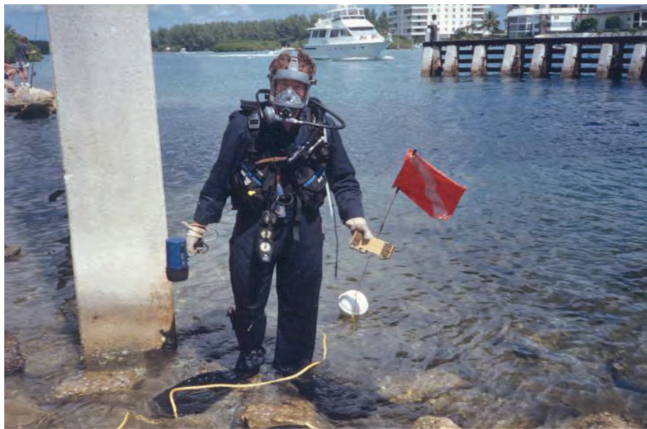
Figure 11.3.4 Self-Contained Inspection Diver
