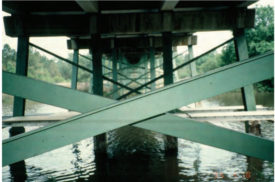
Figure 11.3.16 Steel Pile Bent
