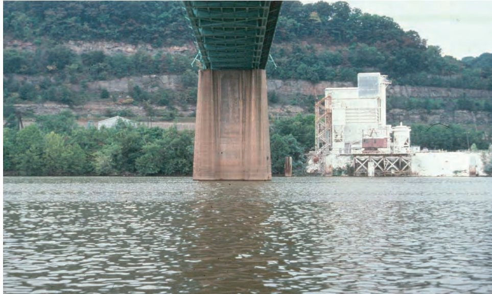
Figure 11.3.18 Column Pier with Solid Web Wall
