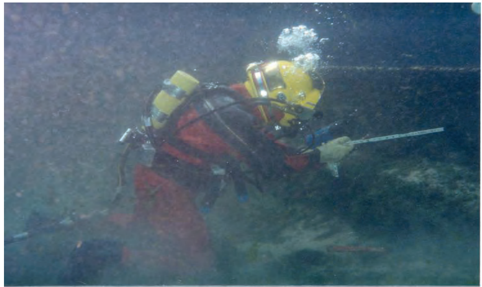
Figure 11.3.5 Surface-Supplied Diving Inspection
