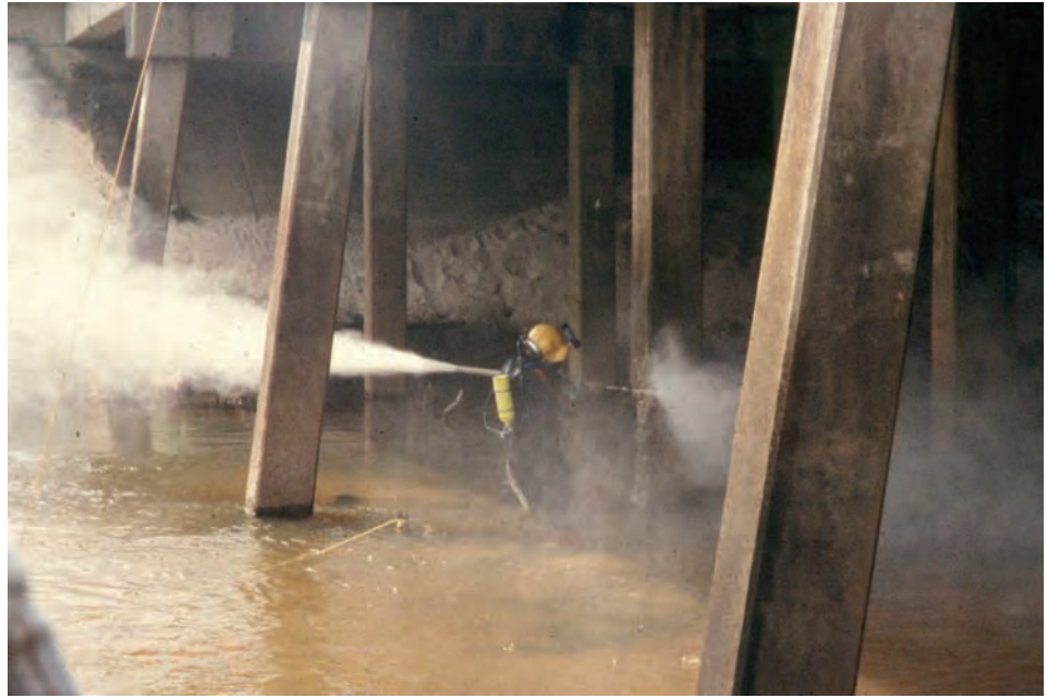
Figure 11.3.41 Cleaning with a Water Blaster
