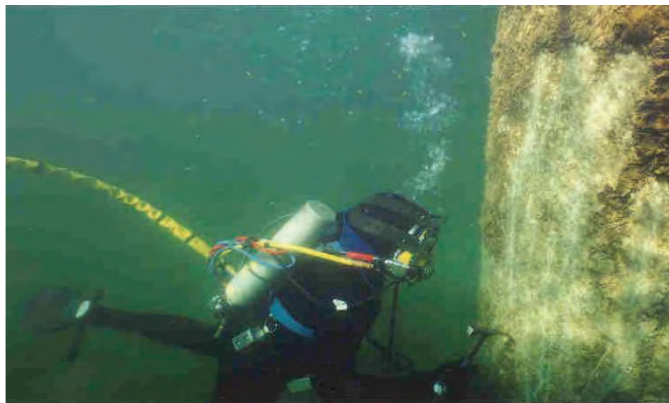
Figure 11.3.6 Diver Cleaning Pier Face For Inspection
