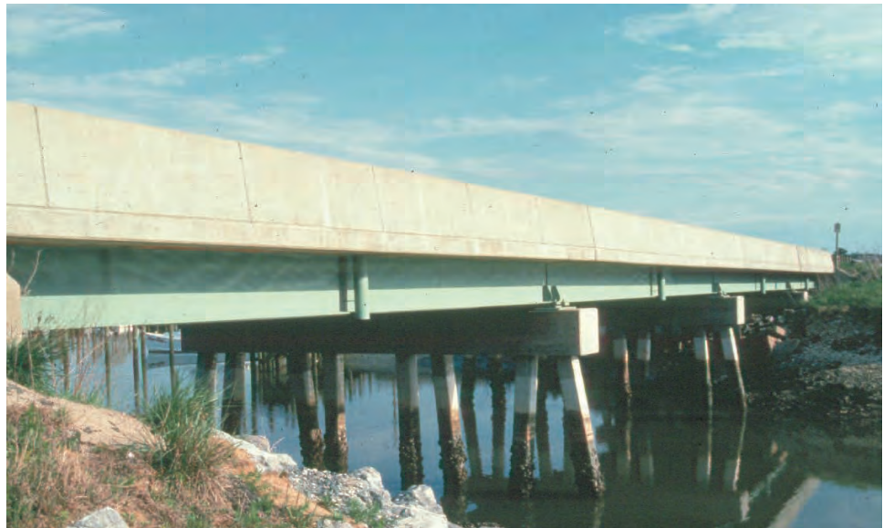
Figure 11.3.17 Concrete Pile Bent
