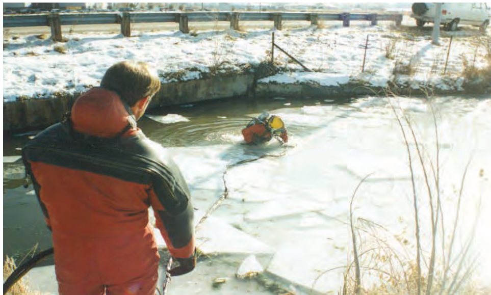
Figure 11.3.22 Inspection of Culvert With Limited Freeboard and Ice Cover
