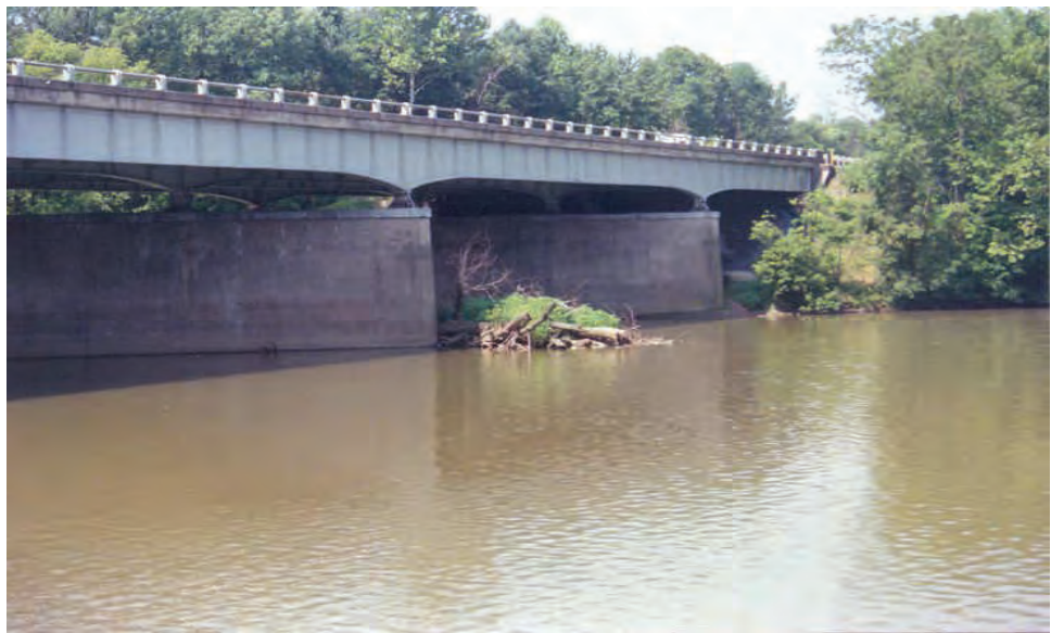
Figure 11.3.13 Buildup of Debris At Pier
