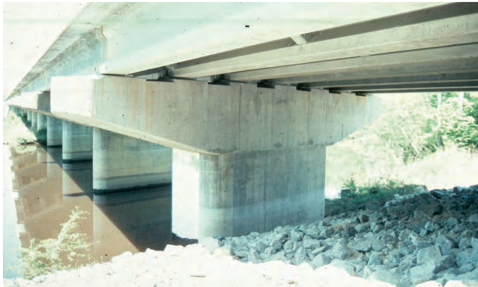
Figure 11.3.19 Cantilever or Hammerhead Pier
