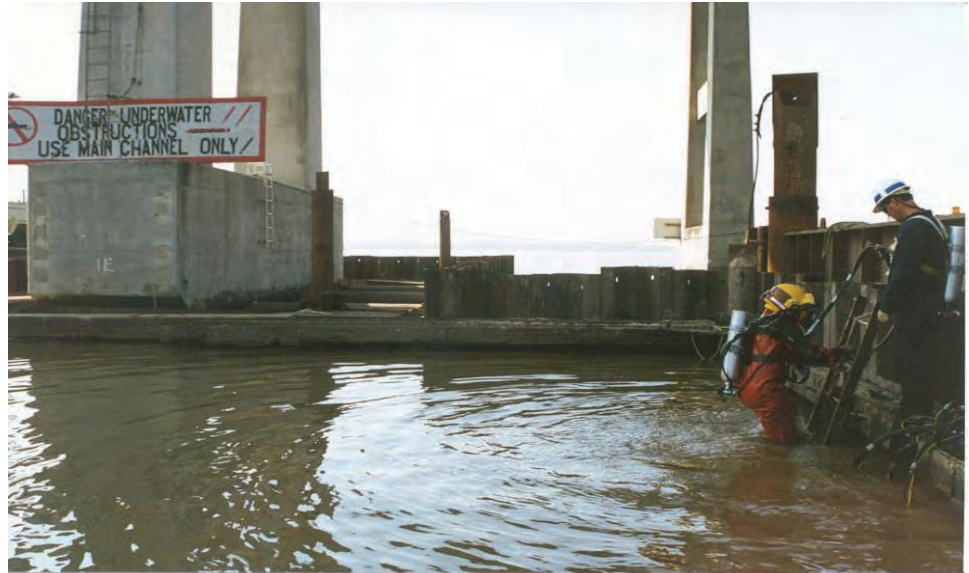
Figure 11.3.50 Diving Inside a Cofferdam
