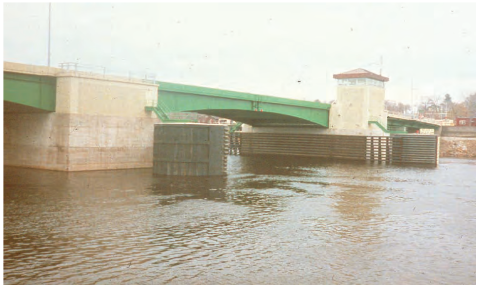
Figure 11.3.7 Bascule Bridge on the Saint Croix River
