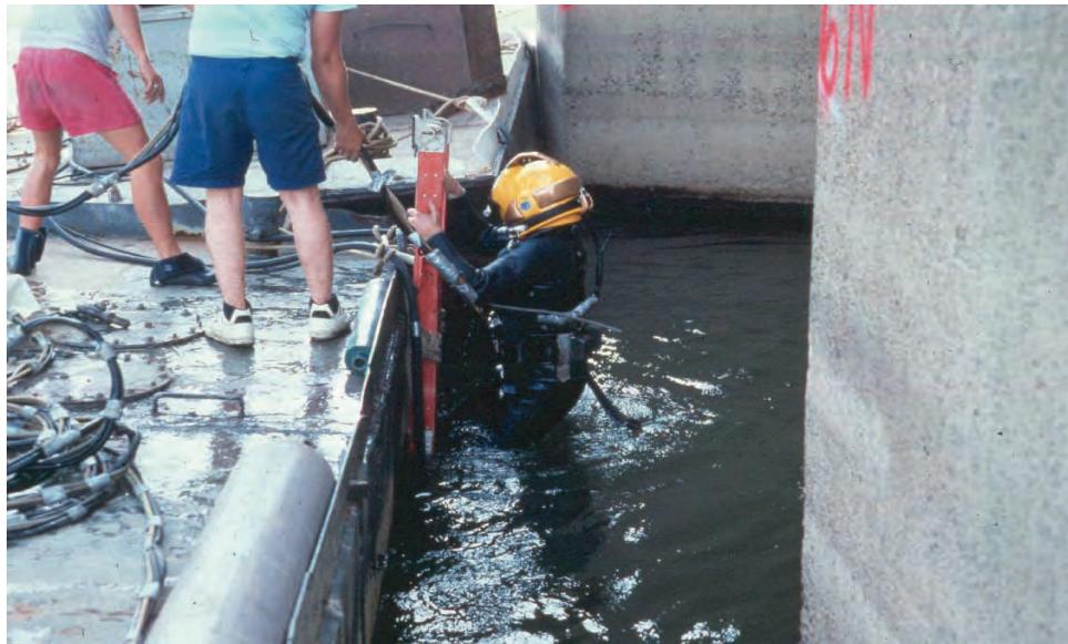
Figure 11.3.38 Access Barge and Exit Ladder
