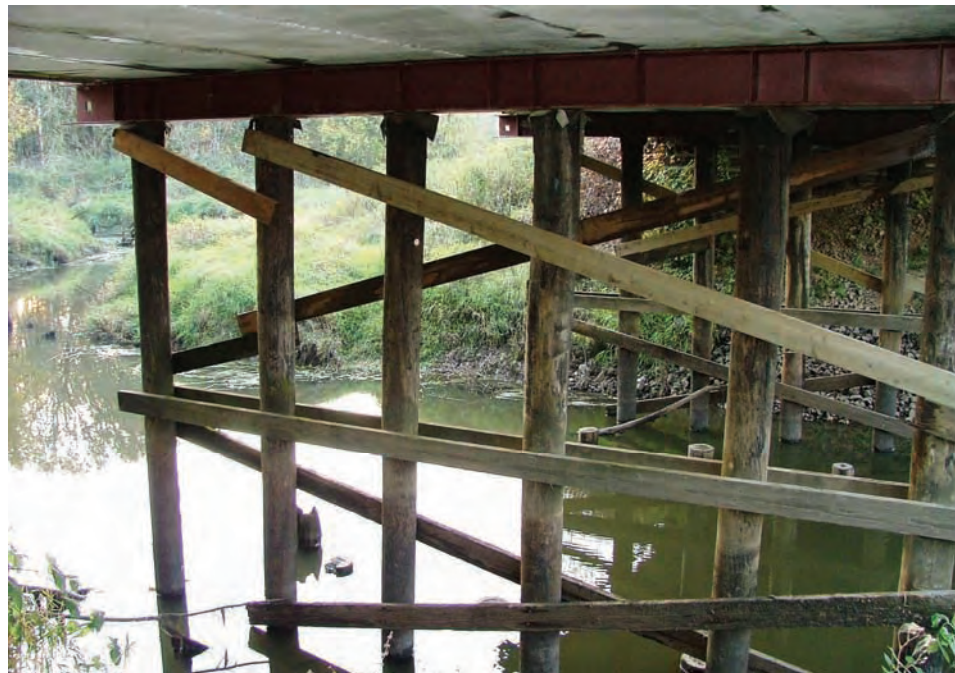
Figure 11.3.15 Timber Pile Bent
