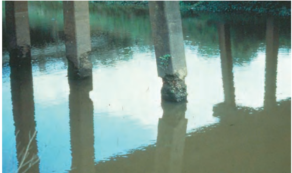
Figure 11.3.26 Concrete Deterioration
