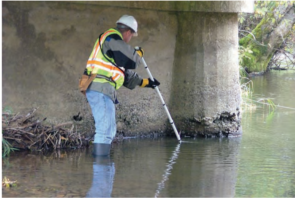
Figure 11.3.3 Wading Inspection
