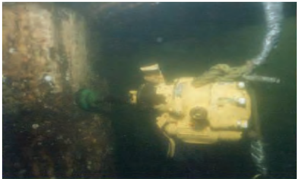
Figure 11.3.44 Concrete Coring Taking Place
