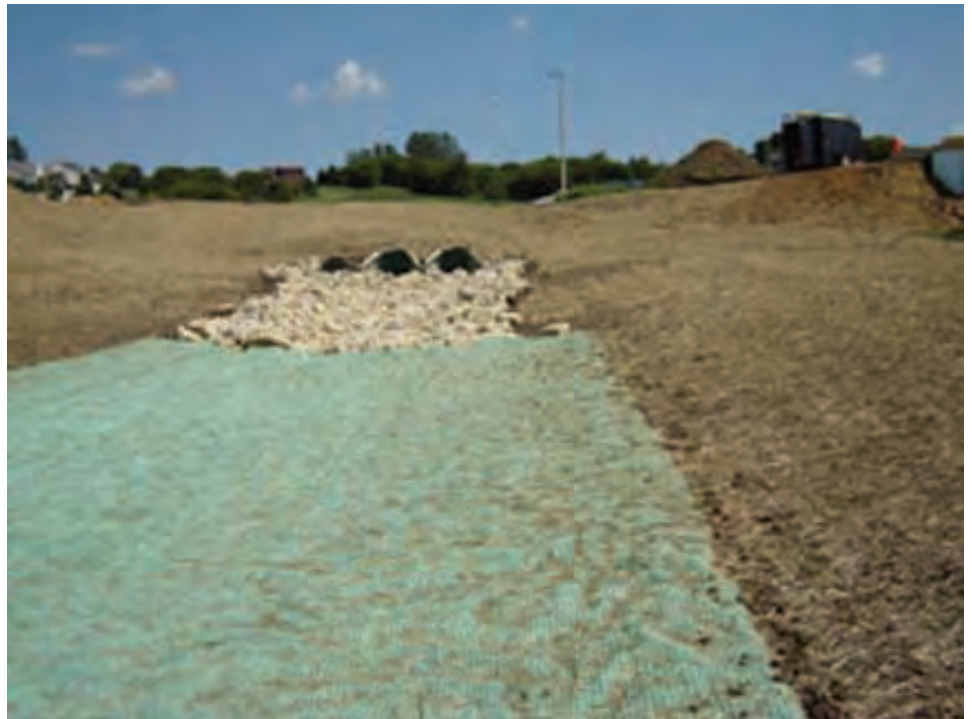
Figure 11.1.11 Wire Mesh and Grass Slope Stabilization
