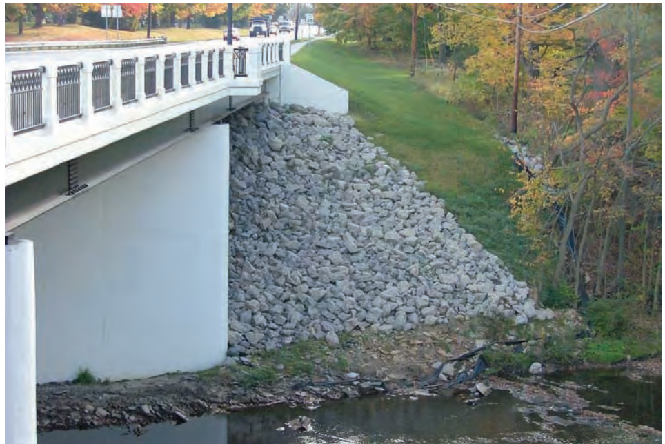
Figure 11.1.7 Crushed Stone Riprap
