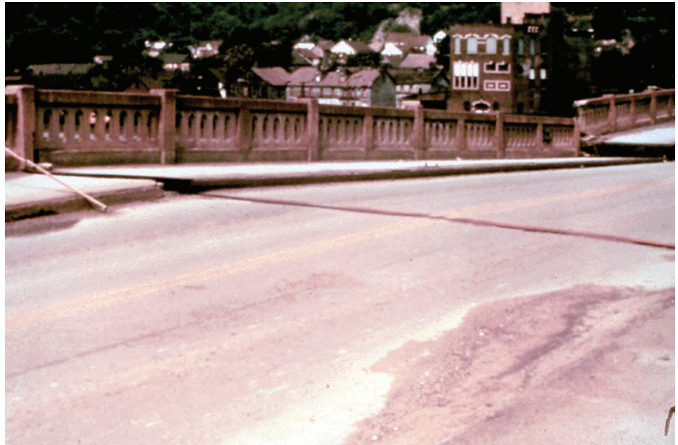
Figure 11.2.30 Superstructure Misalignment
