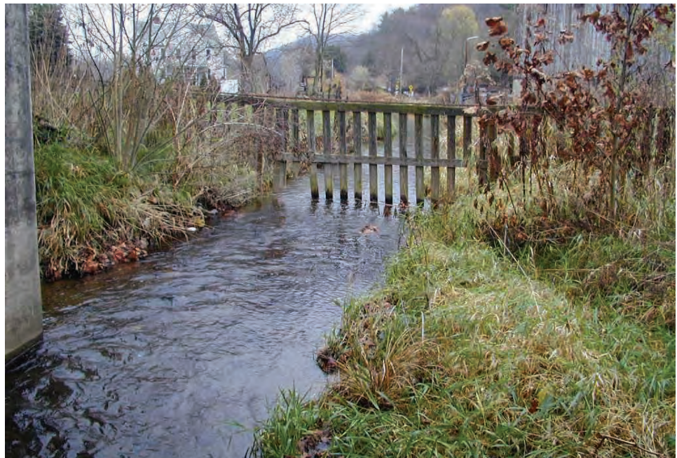
Figure 11.2.39 Fence in Stream at Bridge
