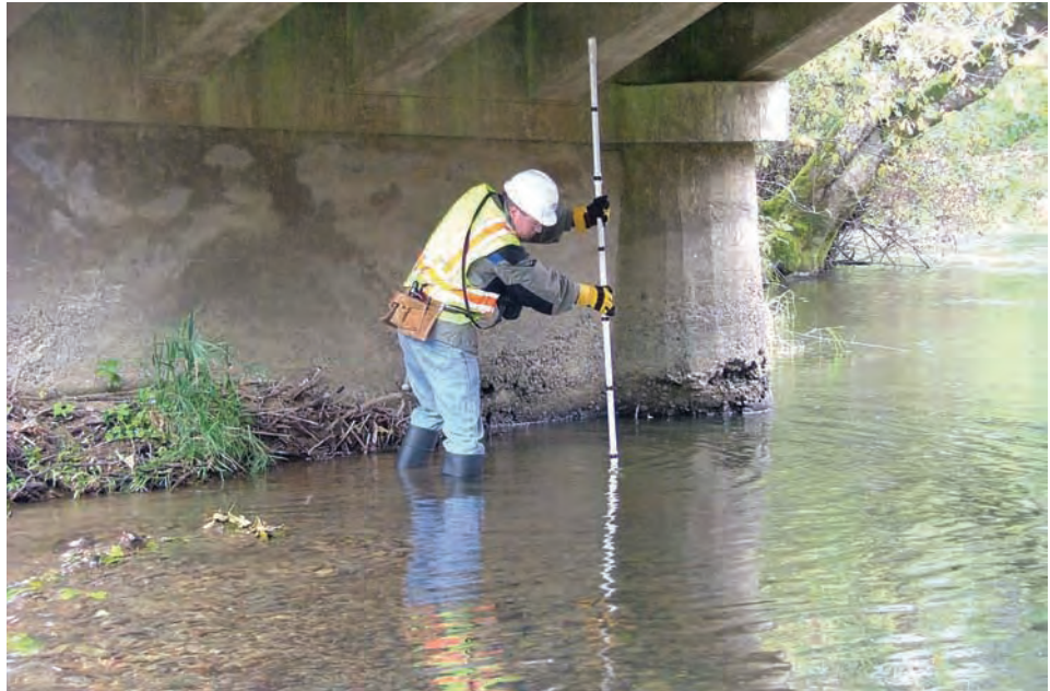
Figure 11.2.22 Probing Rod and Waders
