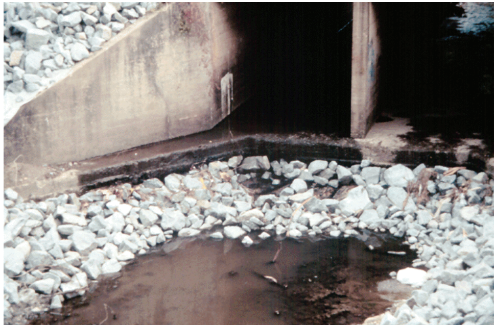
Figure 11.2.33 Failed Riprap
