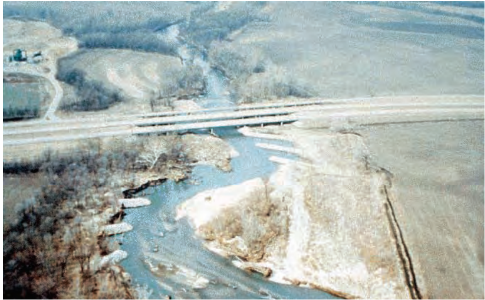
Figure 11.1.8 Spurs Constructed on Mackinaw River (Illinois Route 121)
