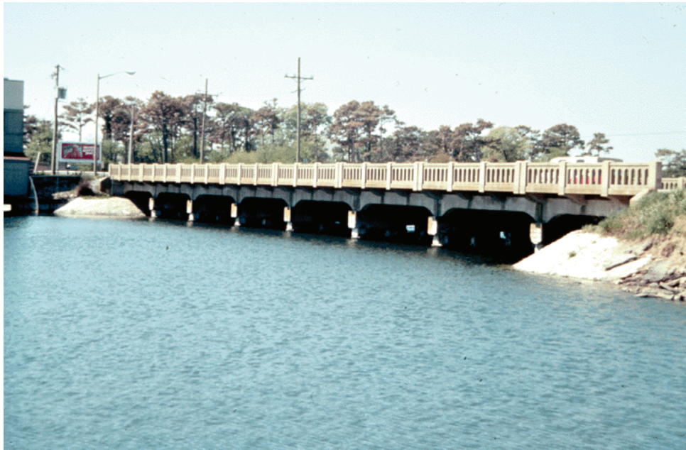
Figure 11.2.32 Typical Simple Multi-Span Bridge
