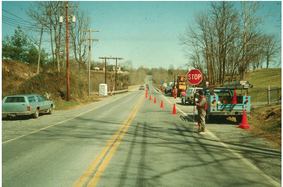
Figure 3.1.4 Traffic Control Operation
