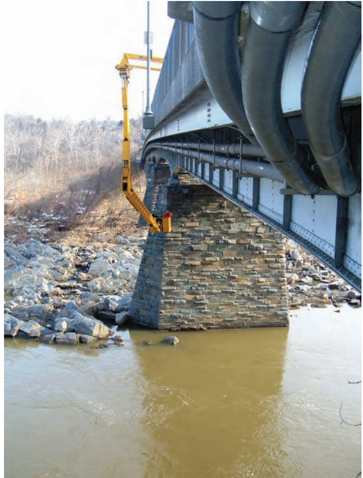
Figure 3.5.16 Underbridge Inspection Vehicle
