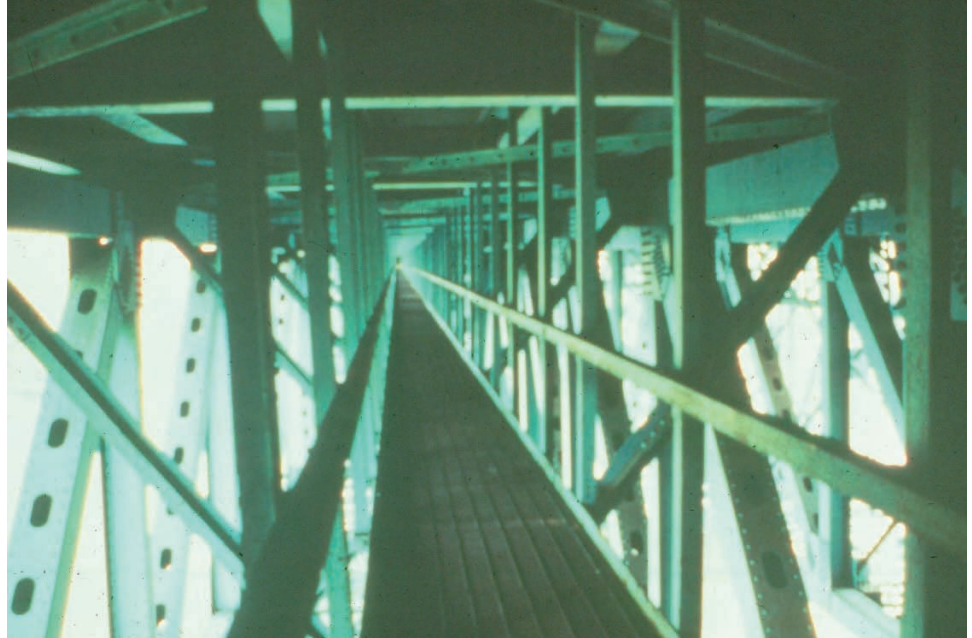
Figure 3.2.11 Inspection Catwalk
