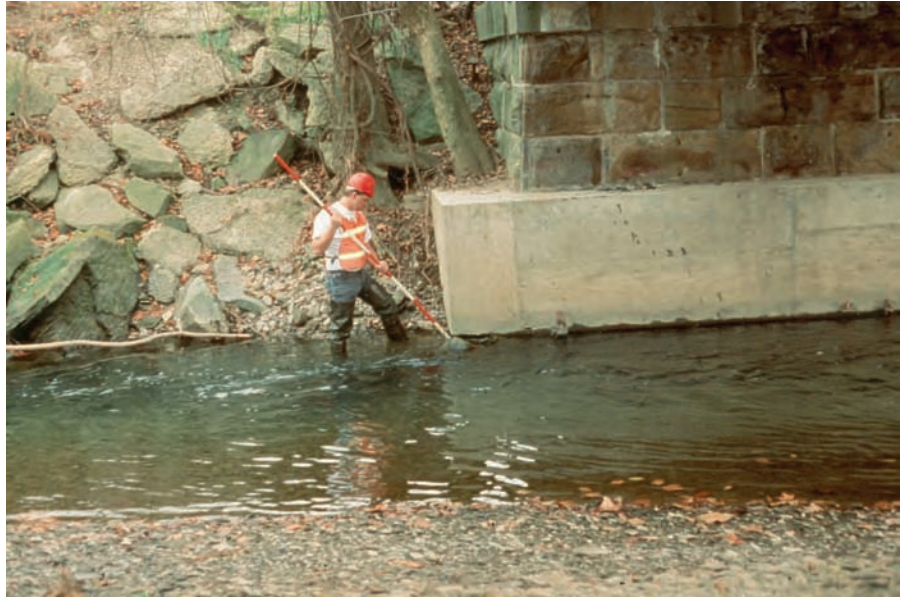
Figure 3.1.5 Inspection for Scour and Undermining
