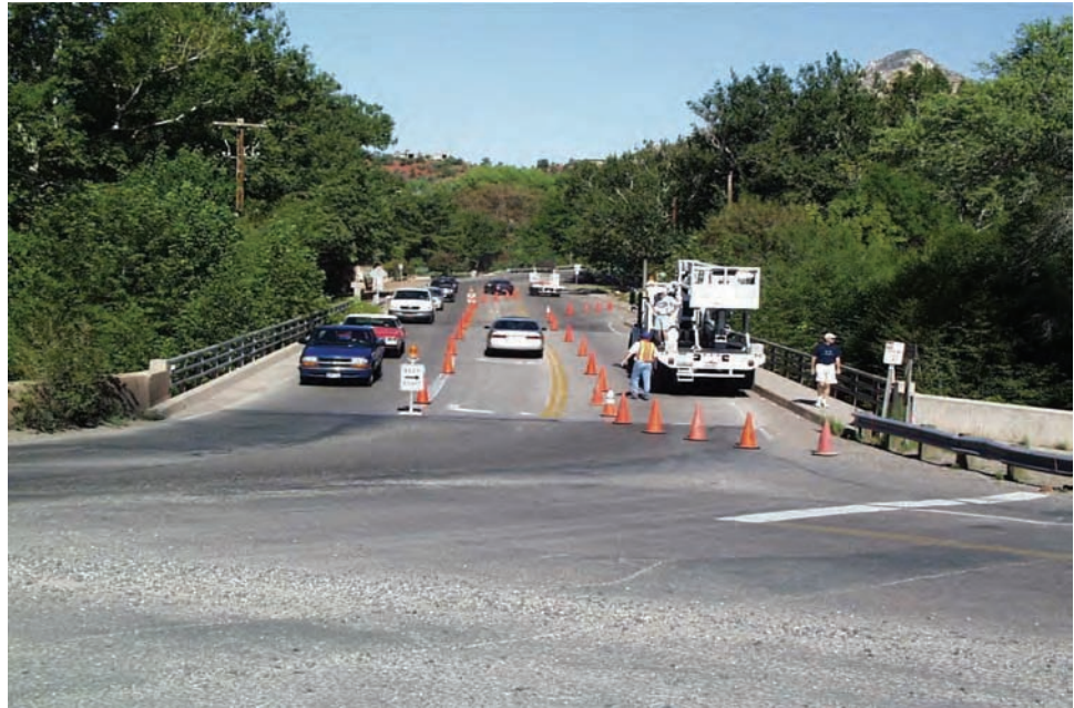
Figure 3.3.1 Traffic Control Operation
