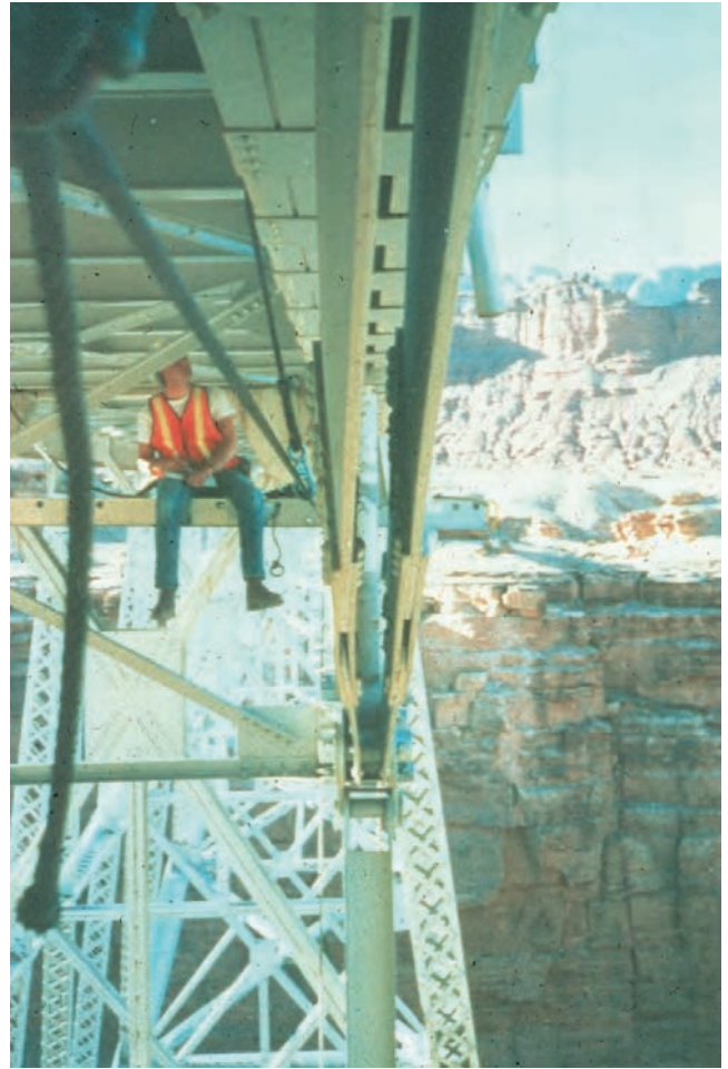
Figure 3.5.4 Rigging for Superstructure Inspection
