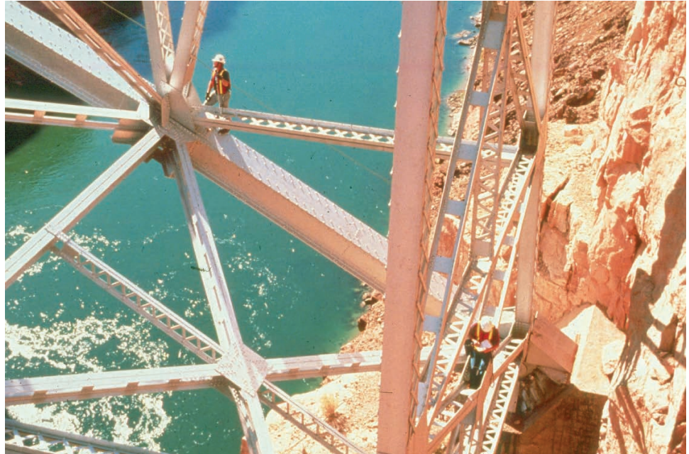
Figure 3.2.7 Inspection Involving Extensive Climbing
