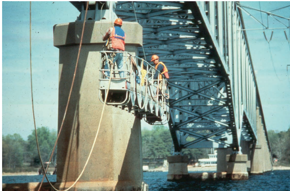
Figure 3.5.3 Rigging for Substructure Inspection
