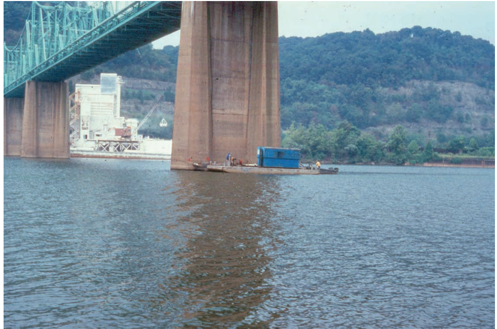
Figure 3.5.6 Inspection Operations from a Barge
