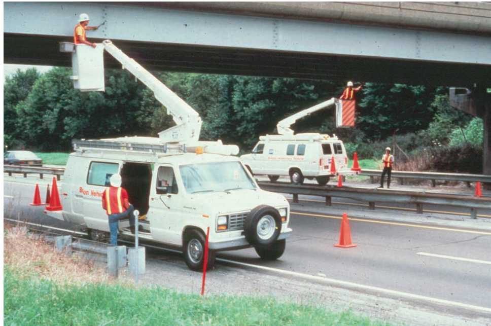
Figure 3.3.3 Inspection Vehicles with Flashing Light
