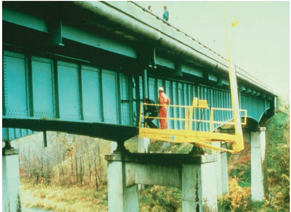
Figure 3.5.17 Underbridge Inspection Vehicle (Snooper) with Platform
