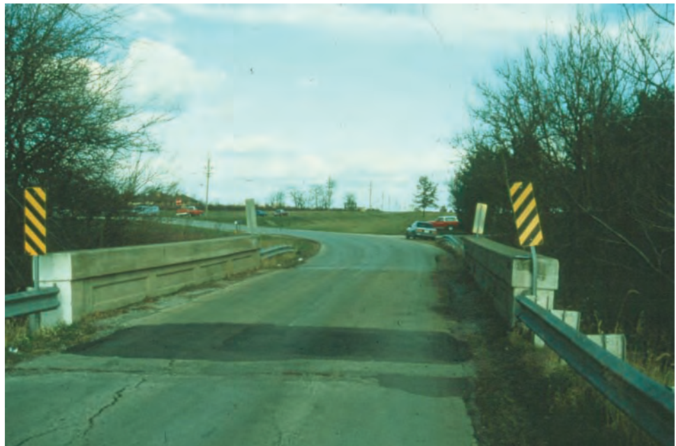
Figure 7.3.2 Concrete Through Girder Bridge
