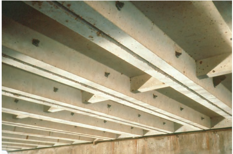
Figure 7.4.1 Underside View of Precast Channel Beam Bridge
