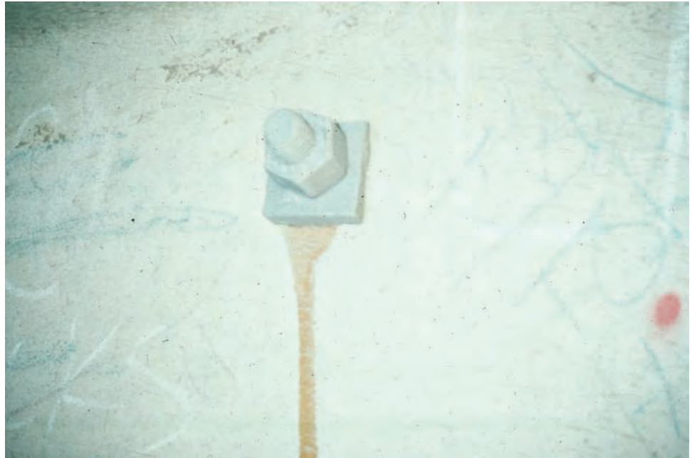
Figure 7.4.9 Close-up of Stem Tie-bolt (Epoxy Resin)
