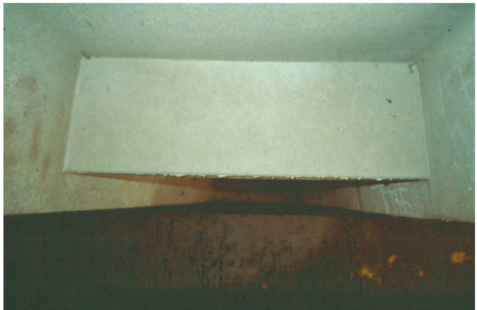
Figure 7.4.10 Close-up of Diaphragm
