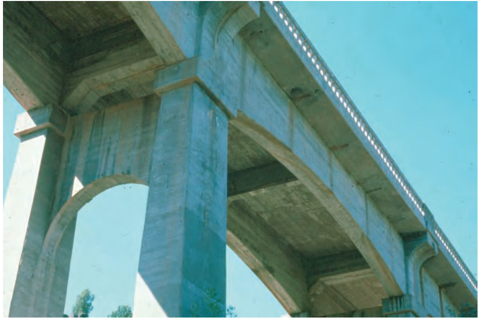
Figure 7.3.3 Concrete Deck Girder, Underside View
