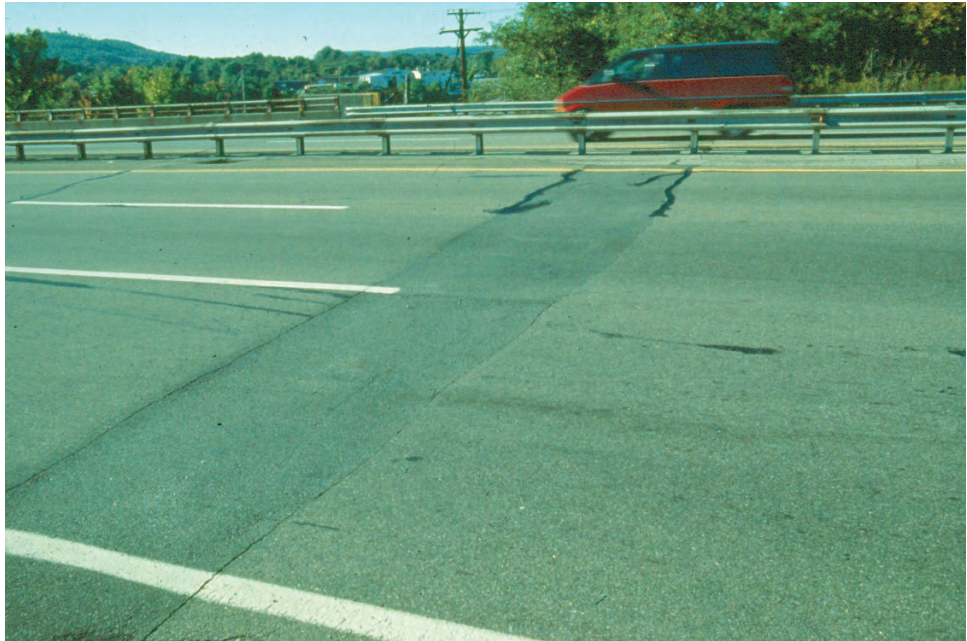
Figure 7.6.14 Roadway of a Rigid Frame Bridge with Asphalt Wearing Surface
