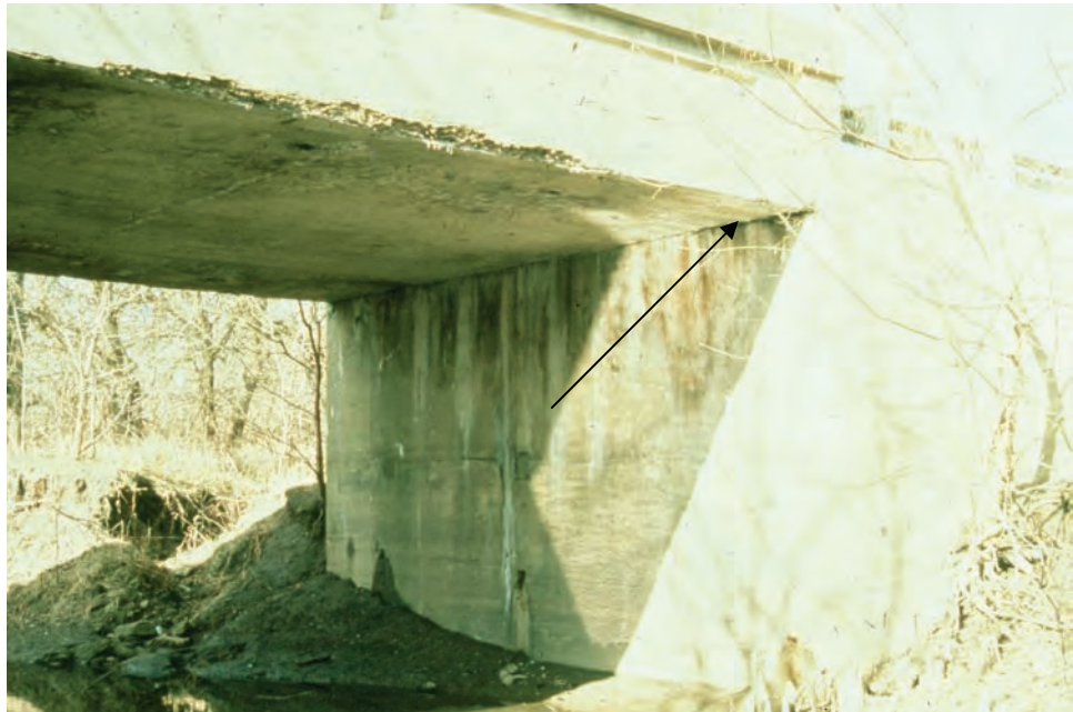
Figure 7.3.6 Bearing Area of a Through Girder Bridge
