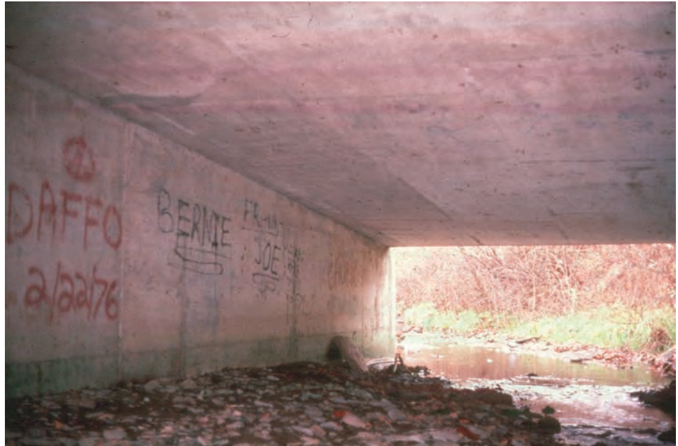
Figure 7.1.4 Bearing Area: Cast-in-Place Slab
