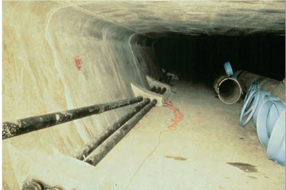
Figure 7.11.44 Inside View of Externally Post-tensioned Box Girder
