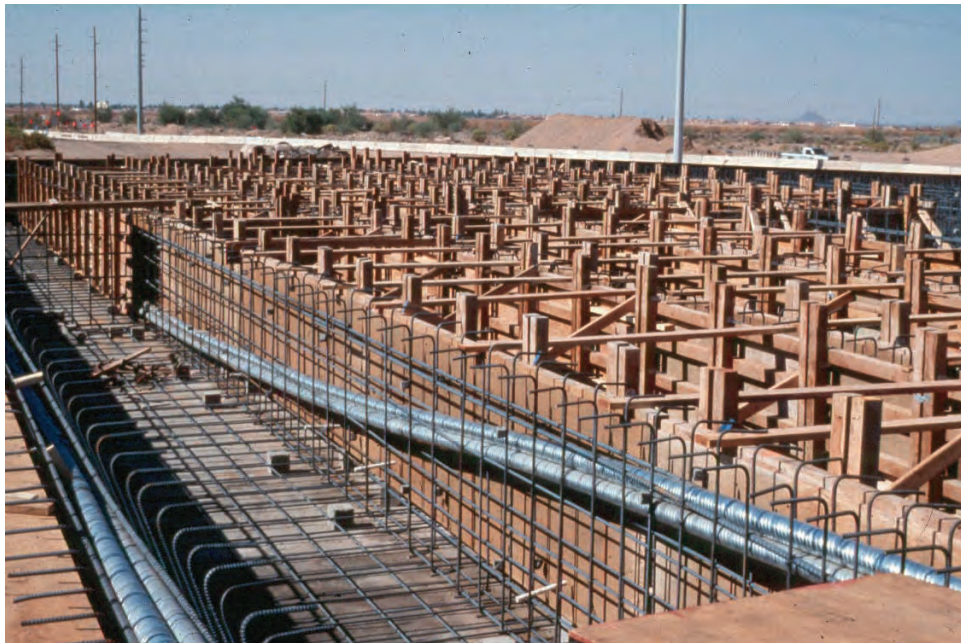
Figure 7.11.36 Post-tensioning Tendon Duct
