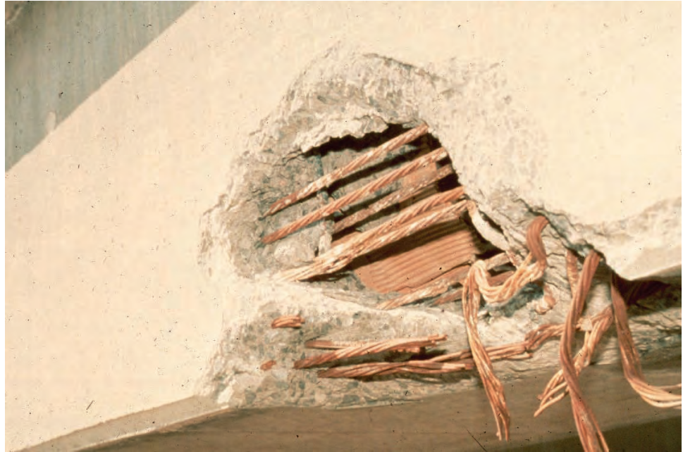
Figure 7.10.17 Close-up of Collision Damage
