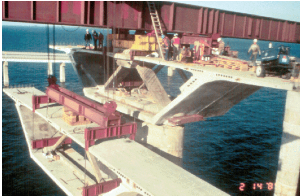
Figure 7.11.18 Balanced Cantilever Construction
