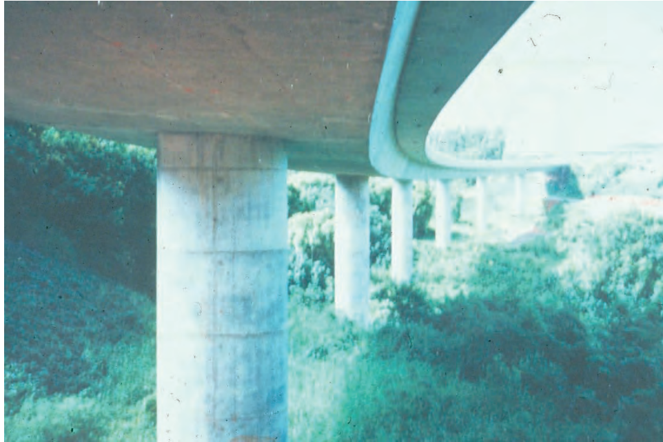
Figure 7.11.2 Cast-in-place Concrete Box Girder Bridge
