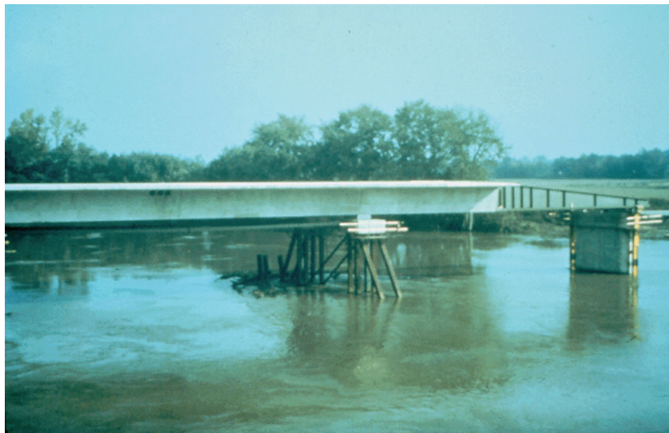
Figure 7.11.25 Incremental Launching Overview (Note Temporary Pile Bent)
