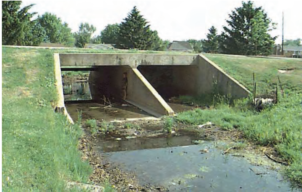
Figure 7.12.2 Multi-cell Concrete Box Culvert
