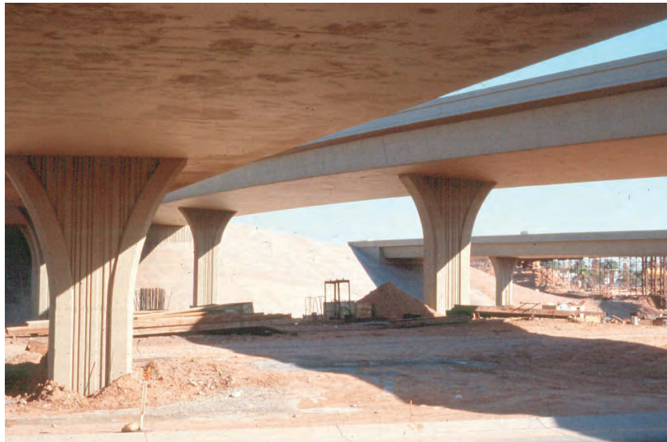
Figure 7.11.7 Box Girder Bridge Construction
