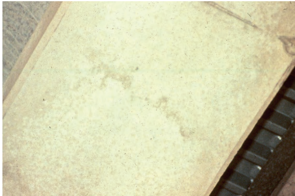
Figure 7.9.11 Flexure Crack
