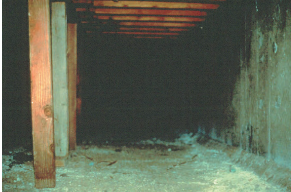
Figure 7.11.37 Interior Formwork Left in Place
