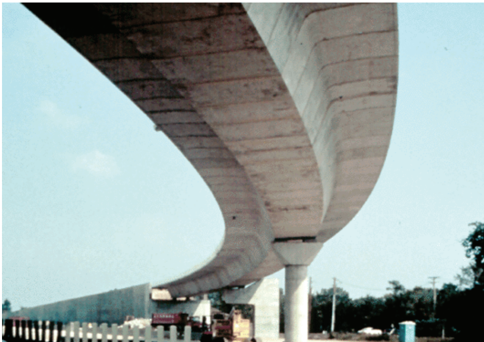
Figure 7.11.13 Segmental Concrete Bridge
