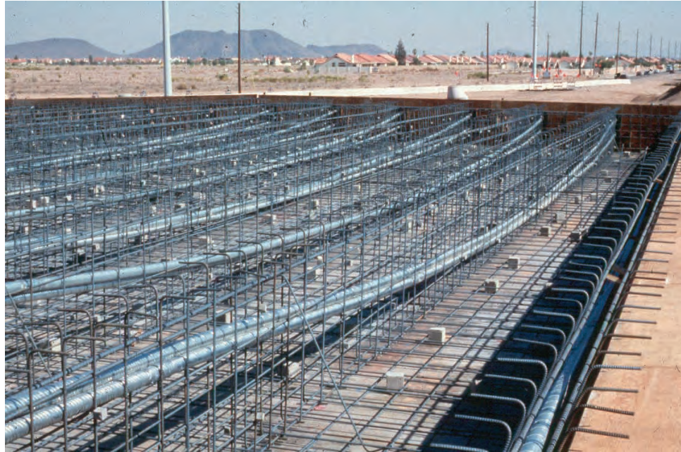
Figure 7.11.6 At-grade Formwork with Post-tensioning Ducts
