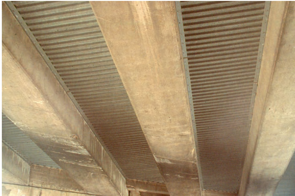
Figure 7.10.7 Underside of a Typical Spread Box Beam
