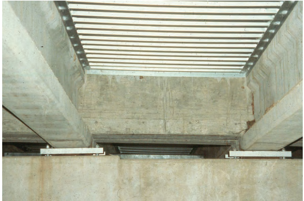
Figure 7.9.12 Typical Concrete Diaphragm
