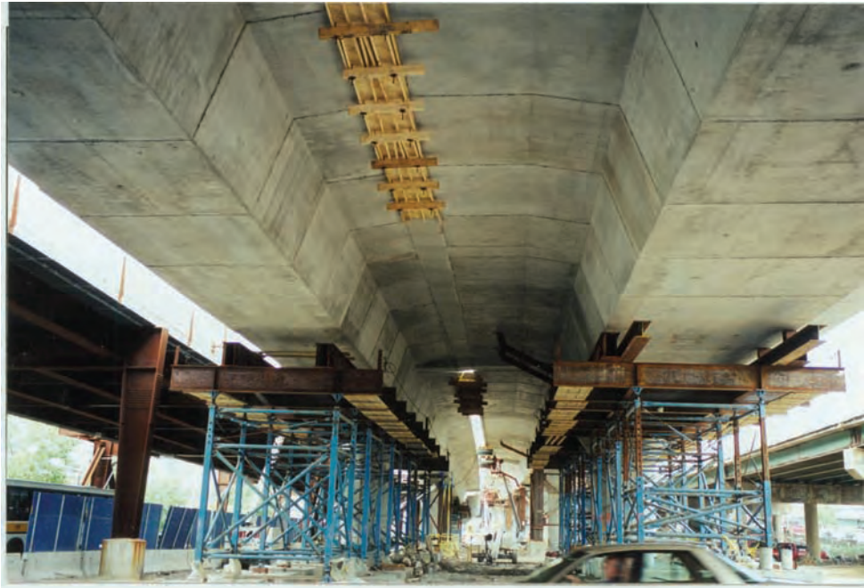
Figure 7.11.12 Adjacent Single Cell Boxes with Closure Pour
