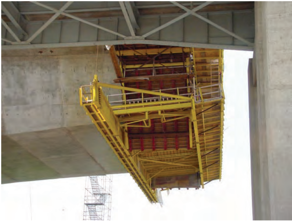
Figure 7.11.15 Cast-in-place Box Girder Segment
