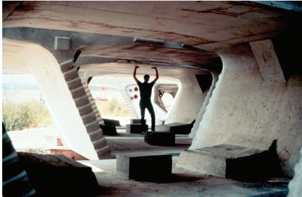
Figure 7.11.16 Box Girder Segment
