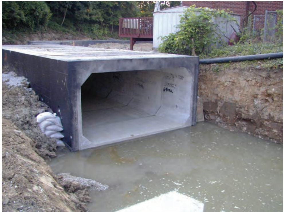
Figure 7.12.4 Precast Concrete Box Culvert
