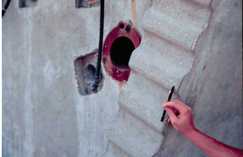
Figure 7.11.41 Close-up View of Box Girder Shear Keys
