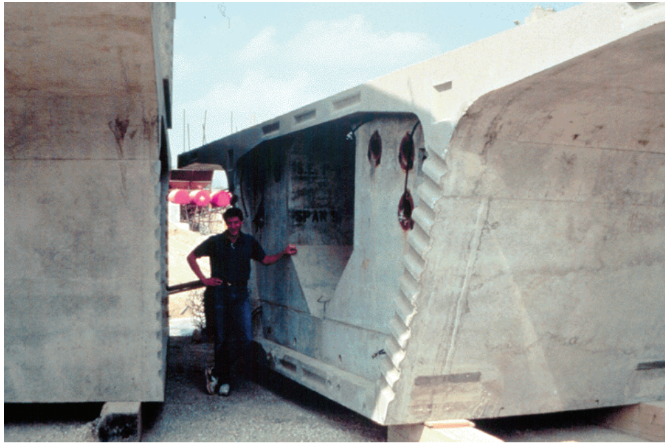
Figure 7.11.43 Box Girder Interior (End) Diaphragm
