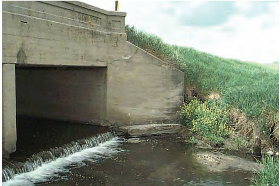
Figure 7.12.9 Cast in Place Concrete Box Culvert Outlet
