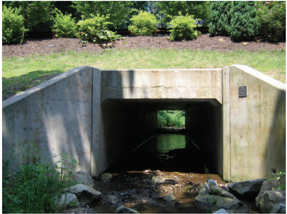
Figure 7.12.1 Concrete Box Culvert
