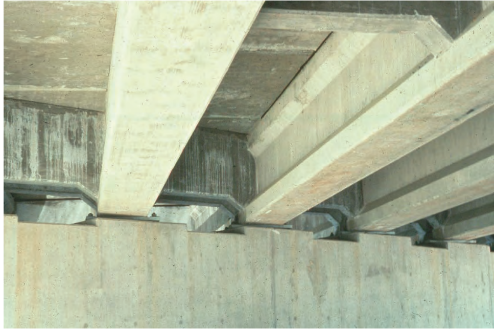
Figure 7.9.7 Concrete End Diaphragm
