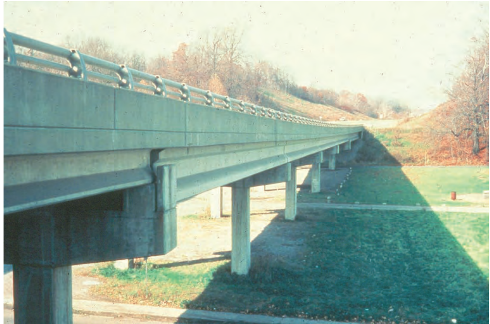
Figure 7.9.1 Prestressed I-beam Superstructure
