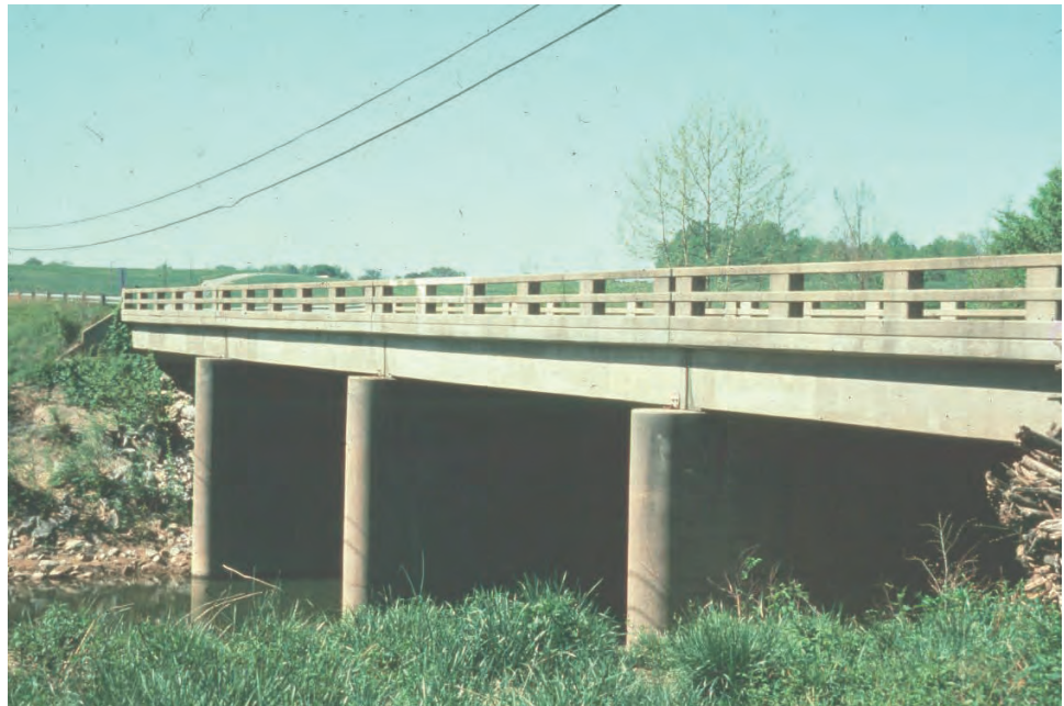
Figure 7.10.1 Typical Box Beam Bridge
