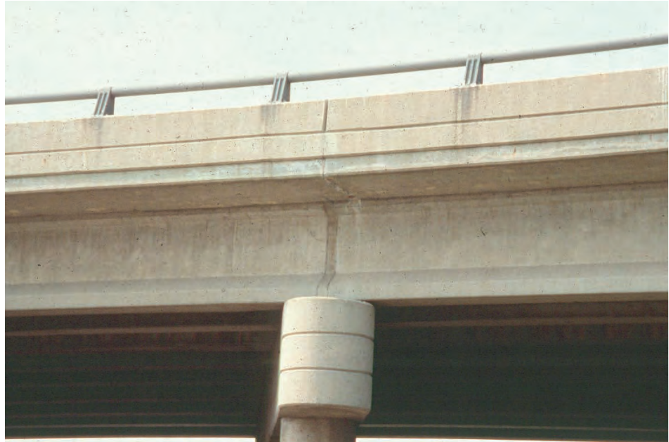
Figure 7.9.5 Continuous Prestressed I-Beam Bridge
