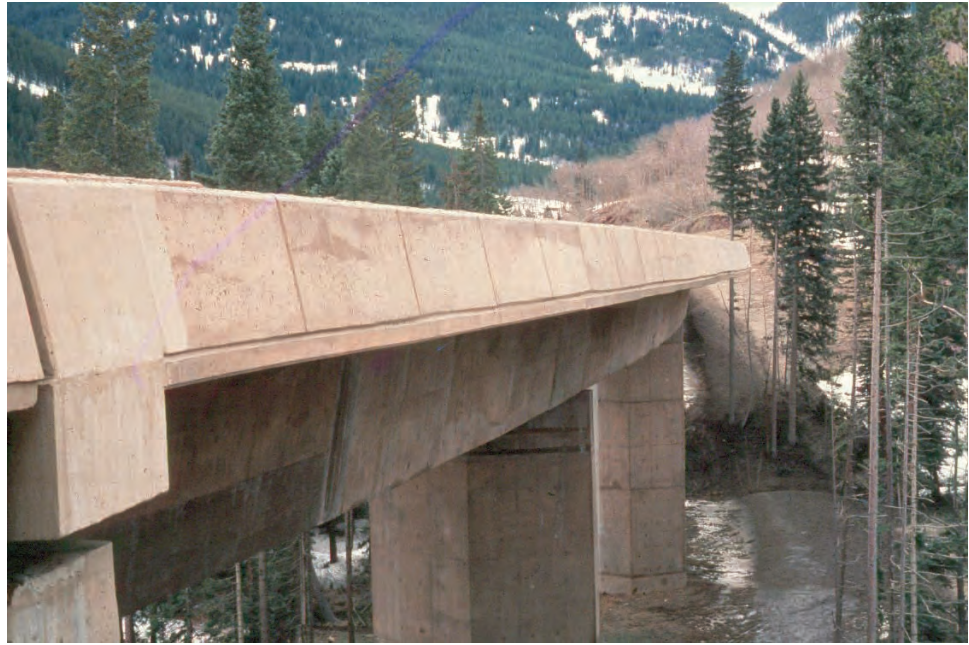
Figure 7.11.4 Cast-in-place Concrete Box Girder Bridge
