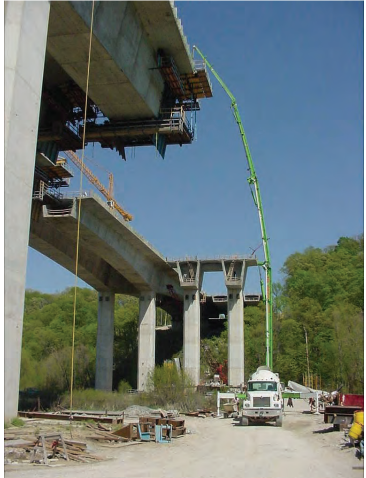
Figure 7.11.23 Progressive Placement Construction
