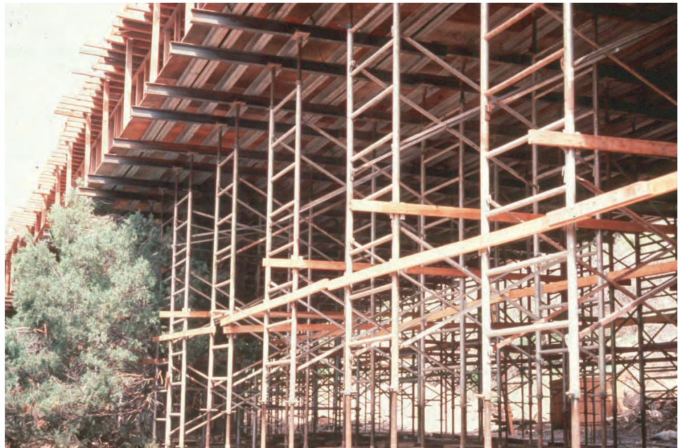
Figure 7.11.5 High Level Casting Formwork on Falsework
