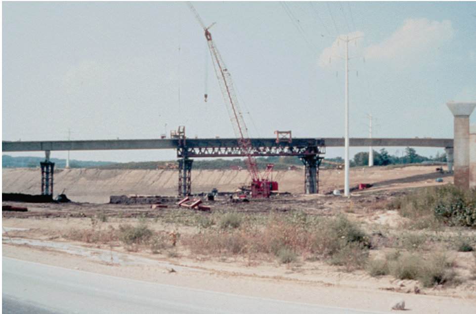
Figure 7.11.20 Span-by-Span Construction (with Erection Truss)
