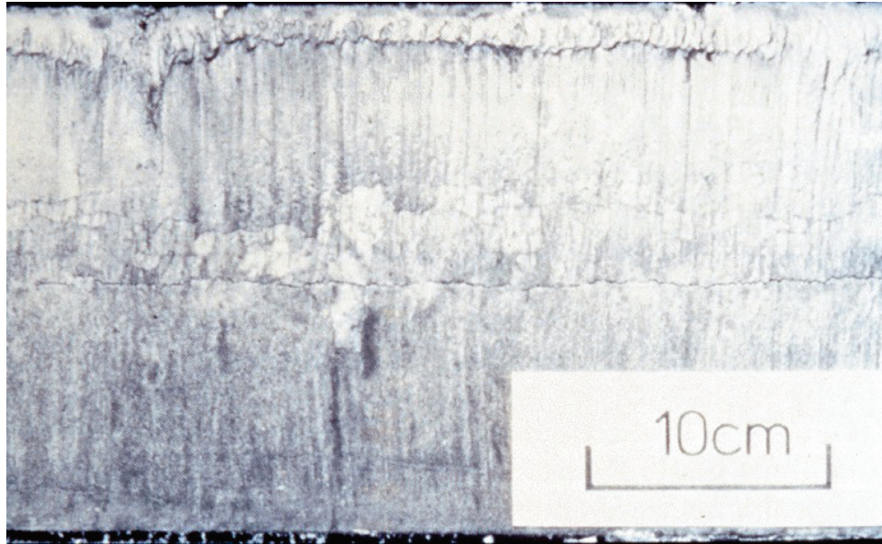
Figure 8.1.17 Centerline Crack in Steel Slab
