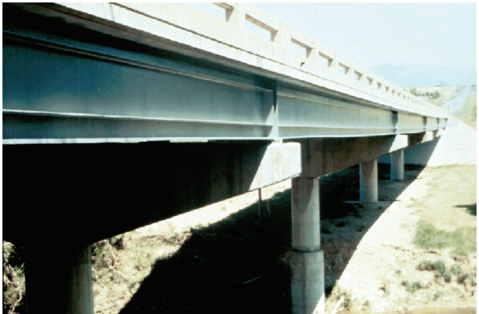
Figure 8.1.4 Structurally Redundant Continuous Span Bridge
