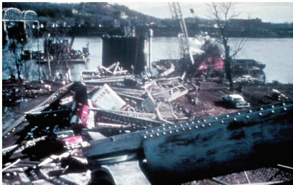
Figure 8.1.1 Silver Bridge Collapse
