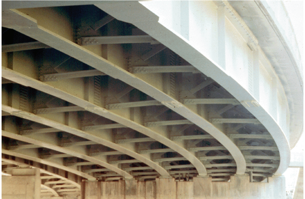
Figure 8.1.3 Load Path Redundant Multi-Girder Bridge
