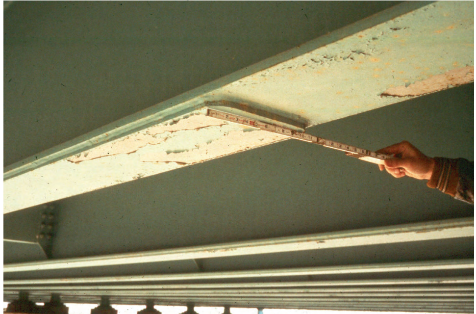
Figure 8.2.3 Rolled Multi-beam Bridge with a Cover Plate
