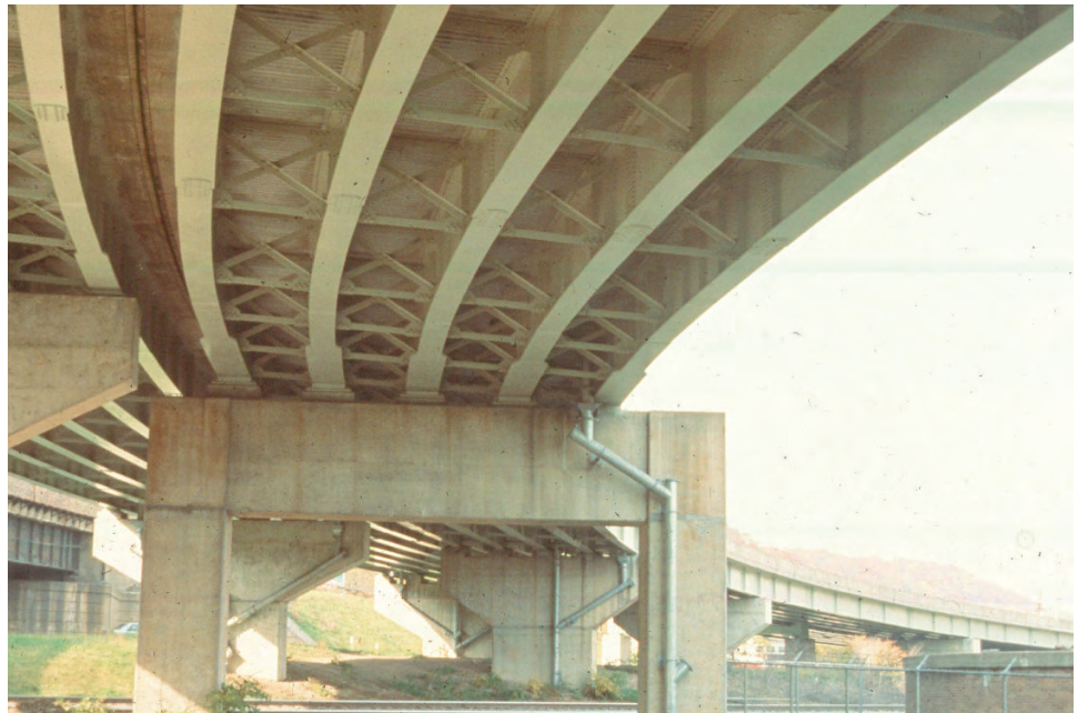
Figure 8.2.8 Curved Fabricated Multi-girder Bridge
