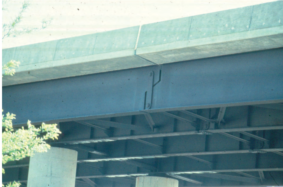
Figure 8.2.9 Fabricated Multi-girder Bridge with Pin & Hanger Connection
