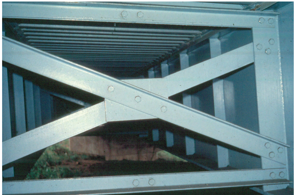
Figure 8.2.22 Intermediate Diaphragm
