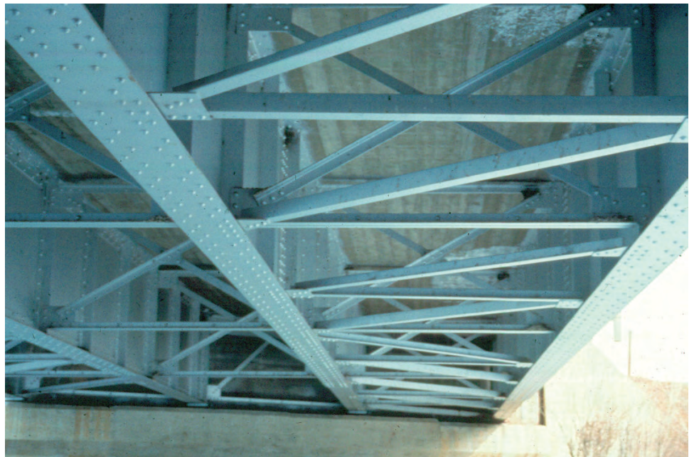
Figure 8.2.15 Straight Multi-girder Bridge
