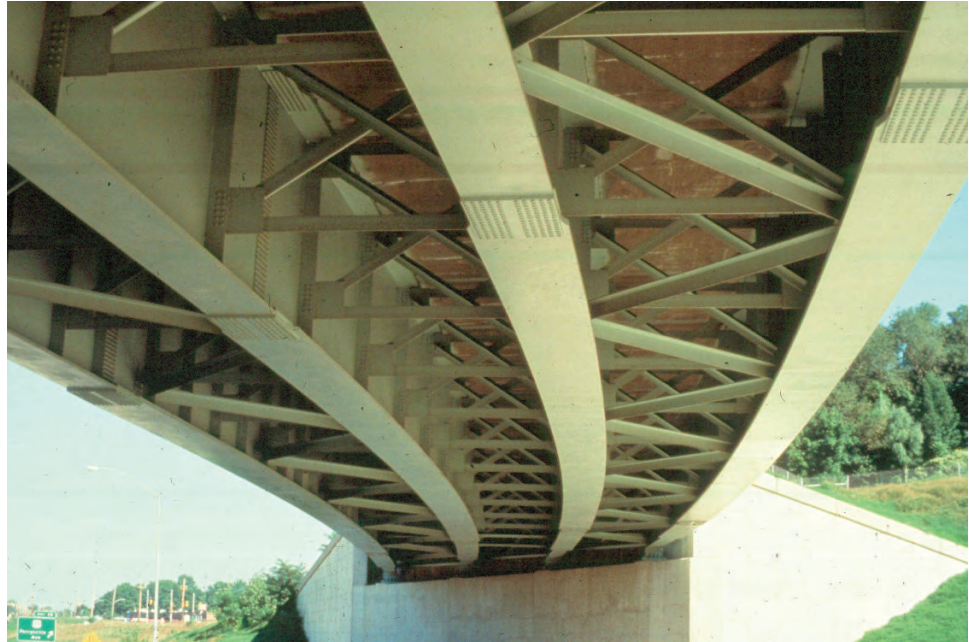
Figure 8.2.14 Curved Multi-girder Bridge
