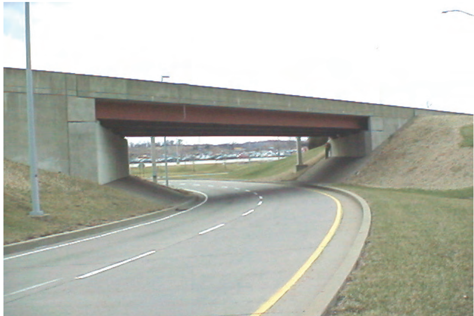
Figure 8.2.6 Single Span Fabricated Multi-girder Bridge
