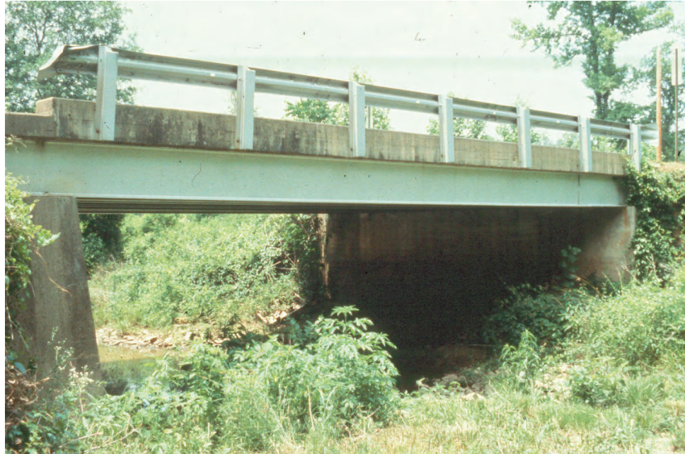
Figure 8.2.1 Simple Span Rolled Multi-beam Bridge
