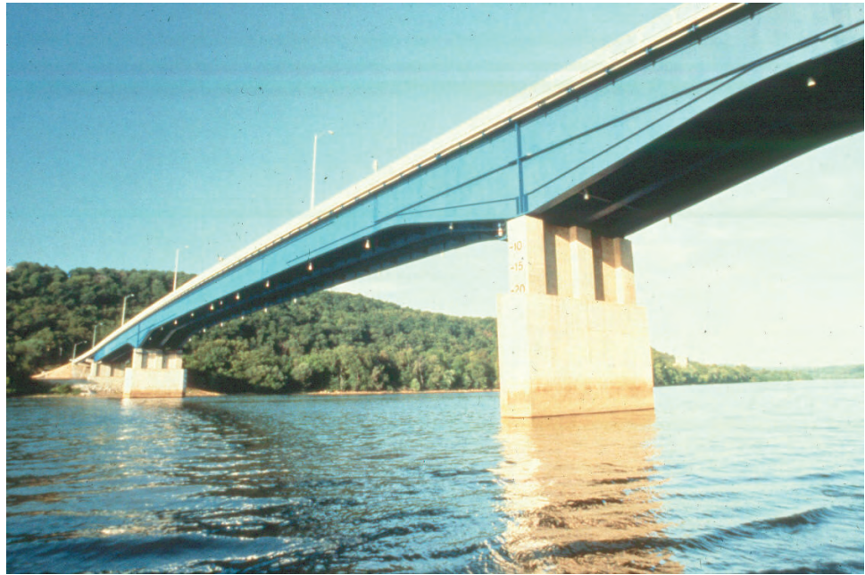
Figure 8.2.12 Fabricated Variable Depth Girder Bridge
