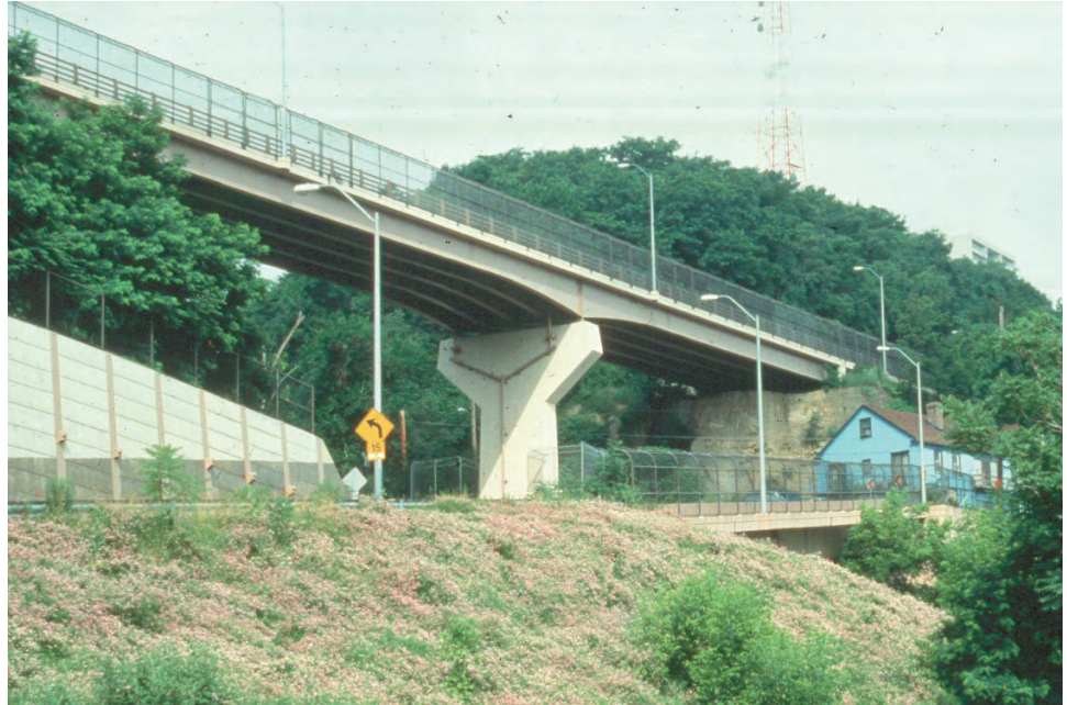
Figure 8.2.7 Continuous Span Fabricated Multi-girder Bridge
