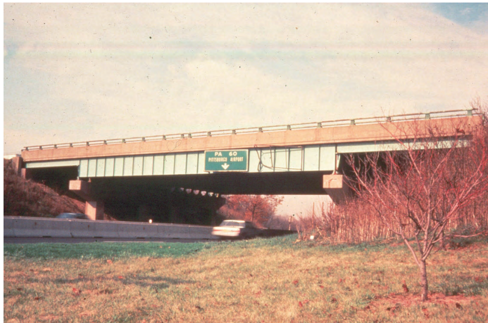
Figure 8.2.10 Combination Rolled Beams and Fabricated Girders
