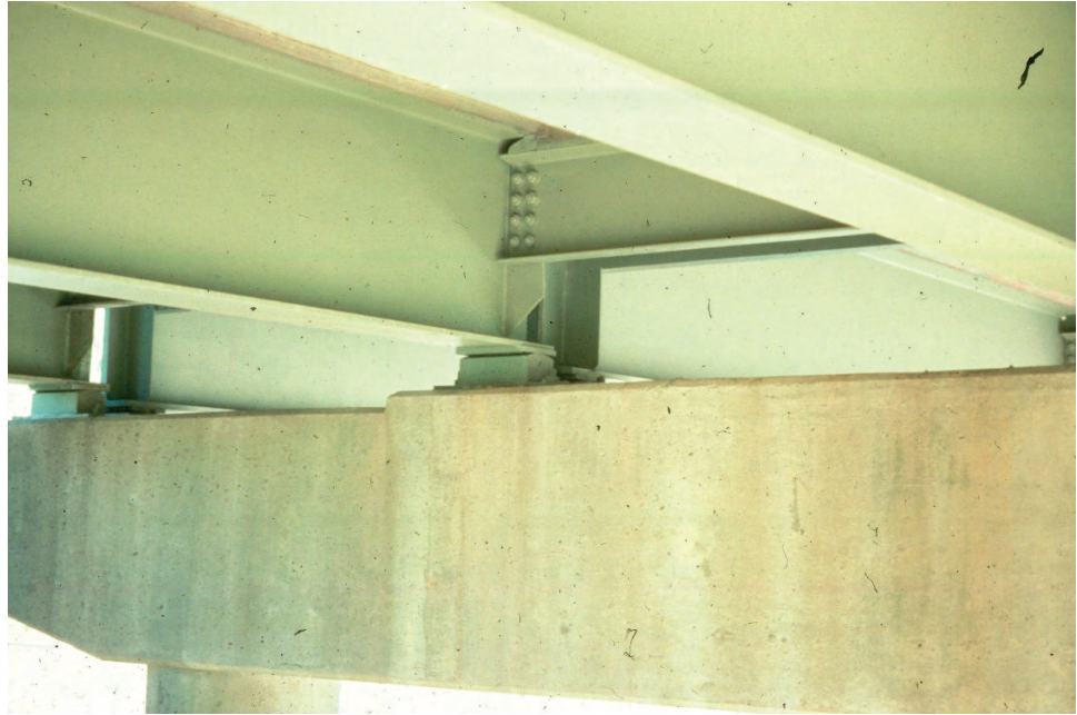
Figure 8.2.21 End Diaphragm
