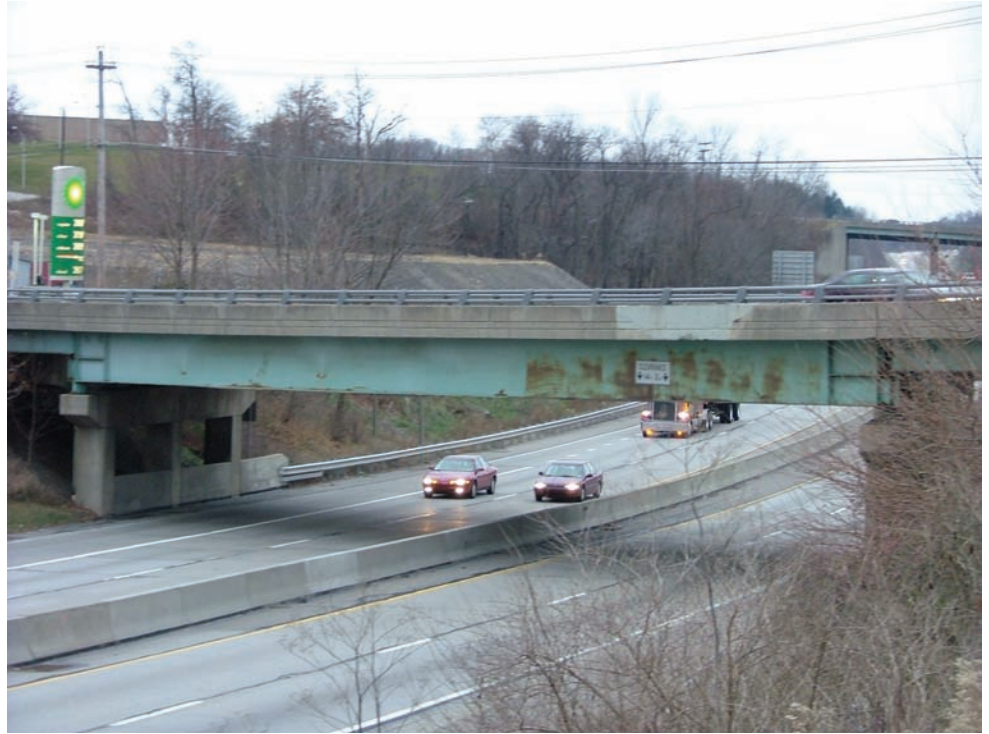
Figure 2.3.21 Roadway Spray Zone Damage
