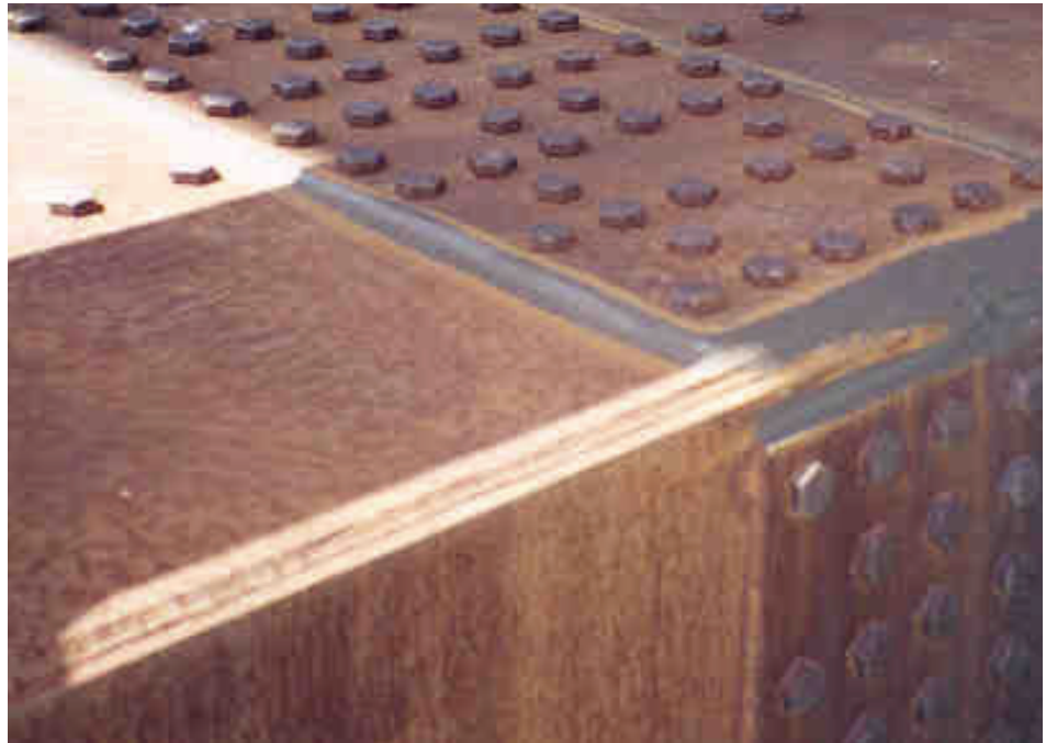
Figure 2.3.24 Light Brown – Early Stage of Exposure
