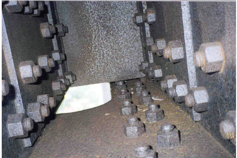
Figure 2.3.26 Black – Non-protective Oxide
