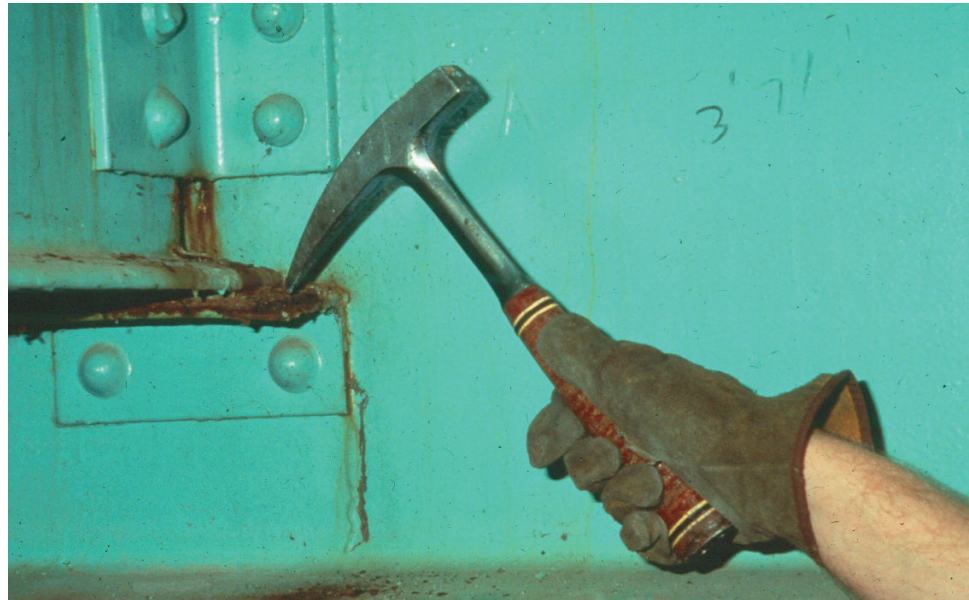
Figure 2.3.16 Corrosion of Steel
