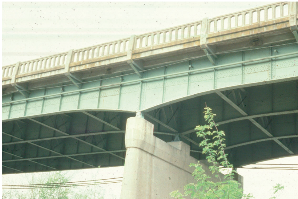
Figure 2.3.5 Built-up Shapes
