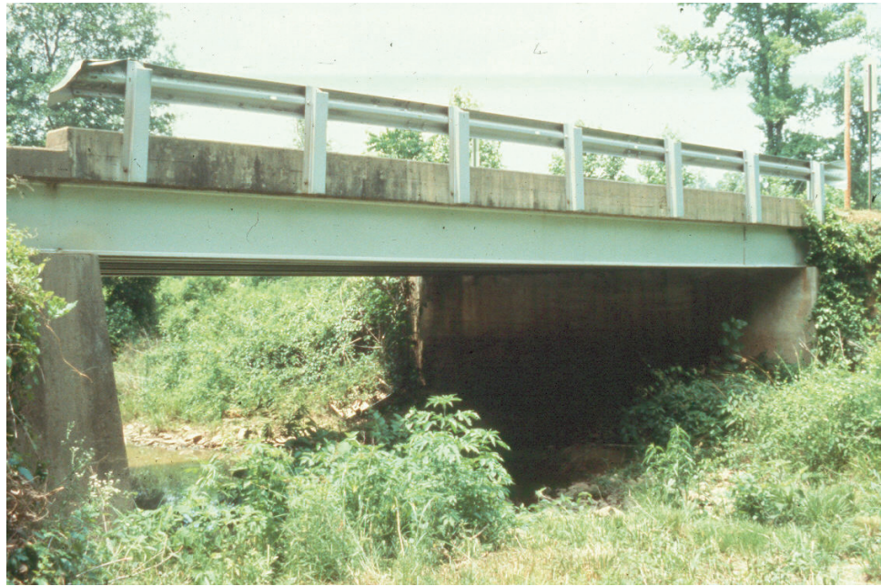
Figure 2.3.4 Rolled Shapes
