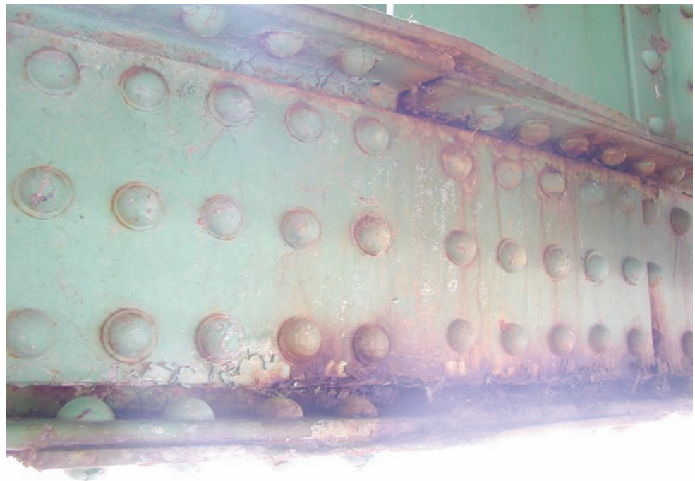
Figure 2.3.20 Corroding Rivet Head
