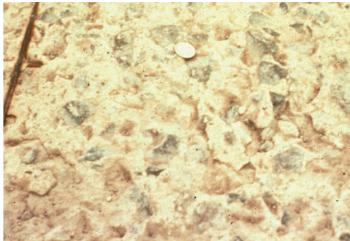
Figure 2.2.19 Severe Scaling
