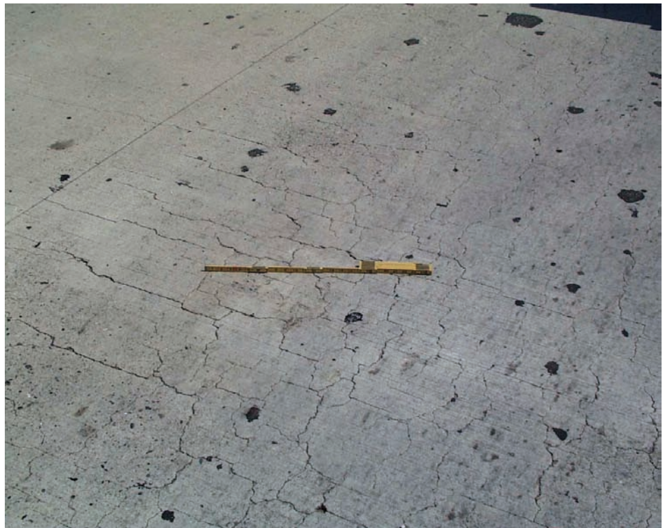
Figure 2.2.12 Shrinkage Cracks
