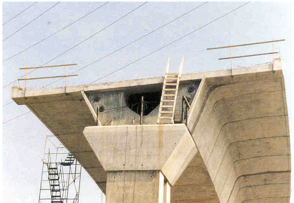
Figure 2.2.5 Post-tensioned Concrete Box Girder
