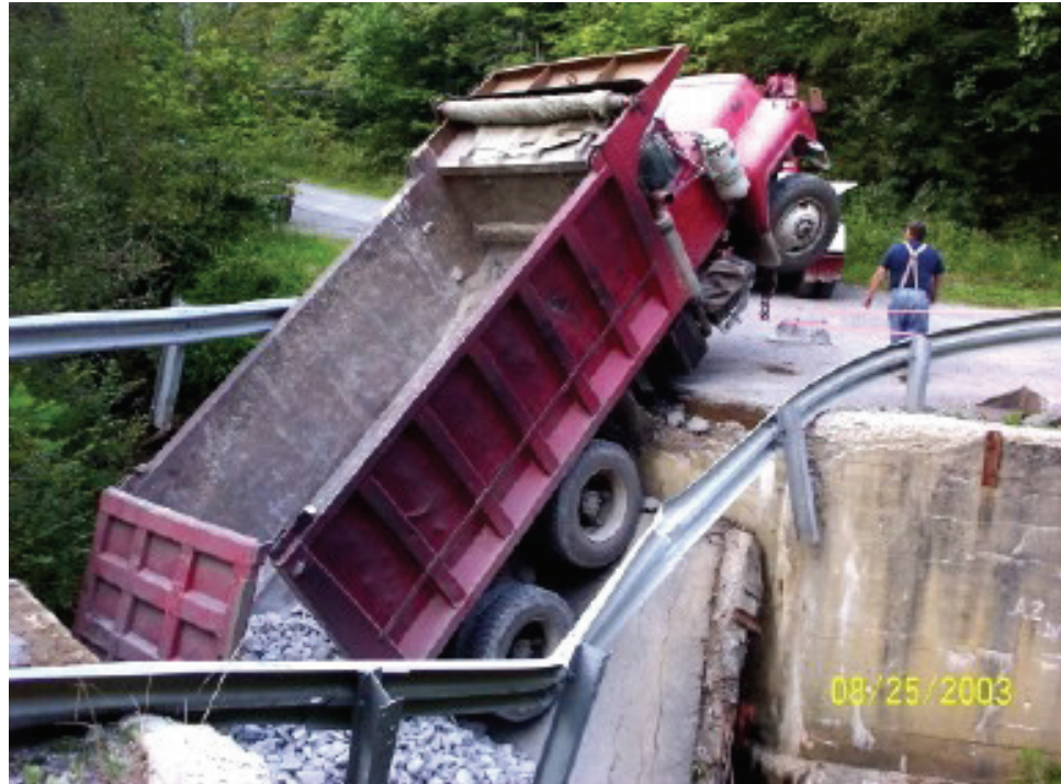
Figure 2.2.25 Overload Damage
