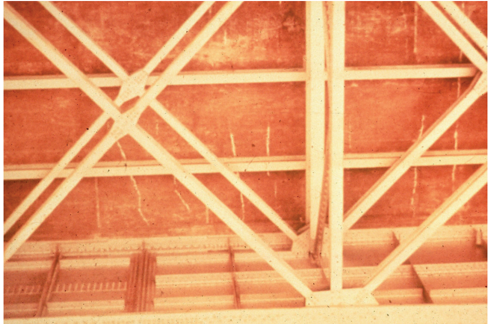
Figure 2.2.13 Transverse Cracks
