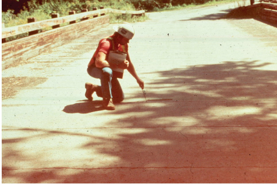
Figure 2.1.27 Inspector Performing a Pick Test
