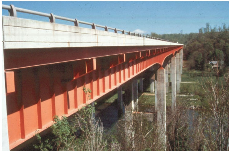
Figure 8.3.13 Flexural Zone on a Two Girder Bridge
