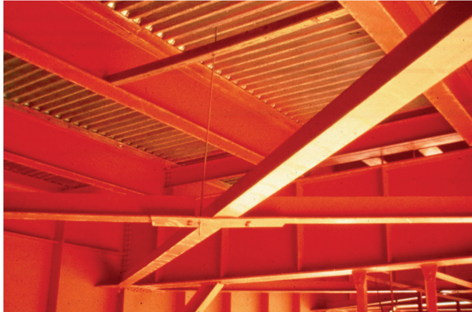
Figure 8.3.8 Underside View of Deck Girder Bridge with Lateral Bracing System
