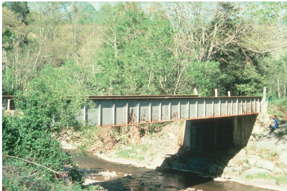
Figure 8.3.15 Flexural Zone on a Through Girder Bridge
