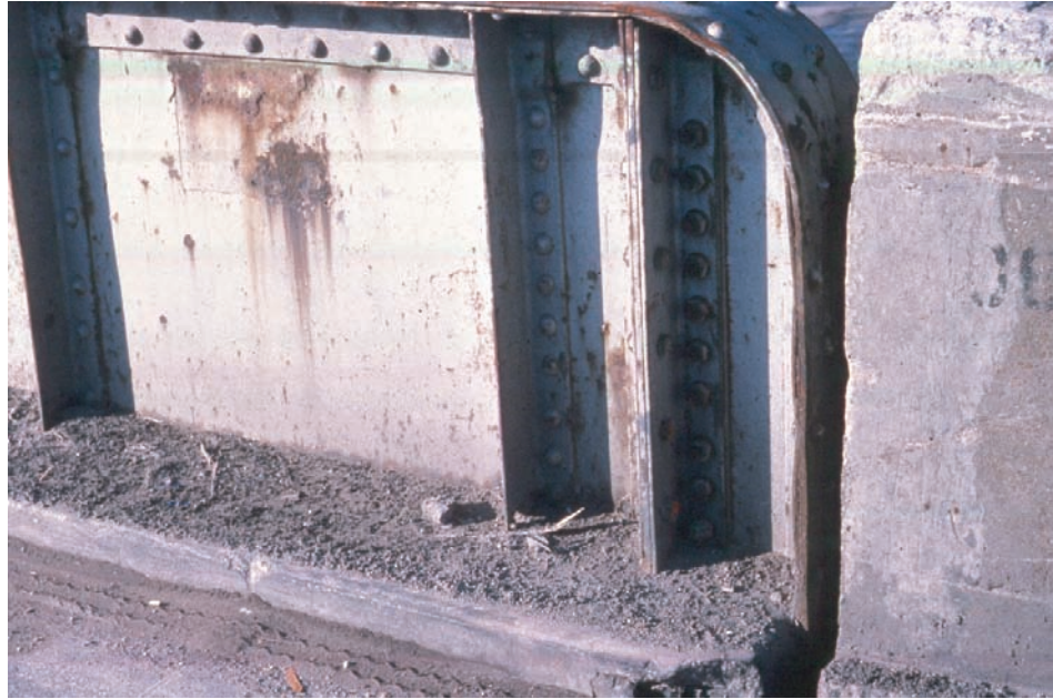
Figure 8.3.12 Web Area Near Support on a Through Girder Bridge
