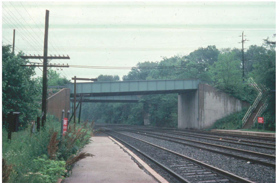
Figure 8.3.3 Through Girder Bridge with Limited Underclearance
