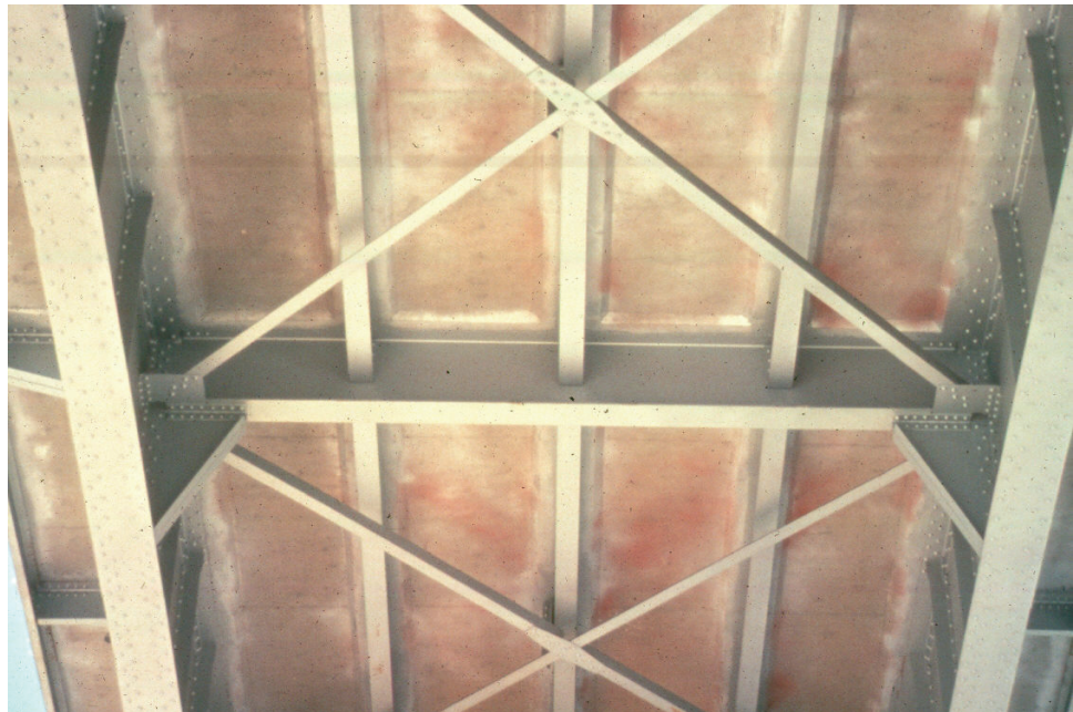
Figure 8.3.6 Two Girder Bridge with Girder-Floorbeam-Stringer System
