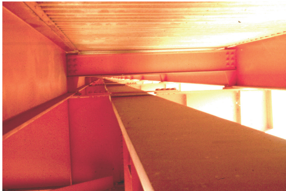
Figure 8.3.29 Tie Plate for Cantilever Floorbeam
