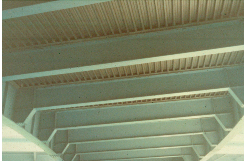
Figure 8.3.5 Two Girder Bridge with Girder-Floorbeam System
