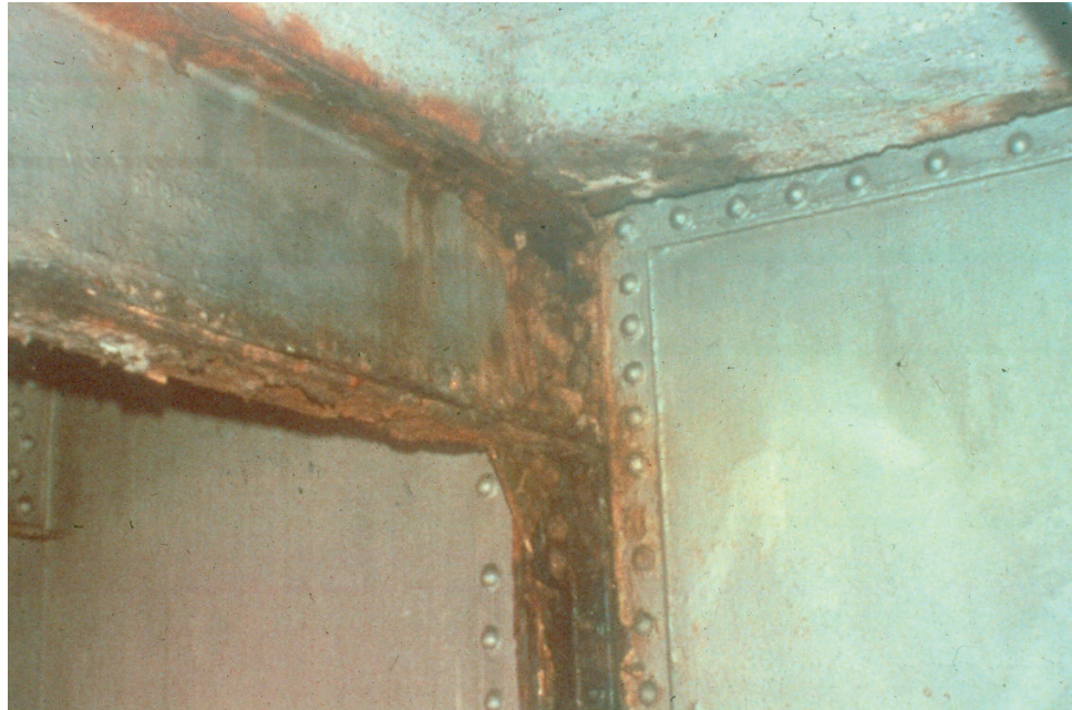
Figure 8.3.11 Shear Zone on a Deck Girder Bridge
