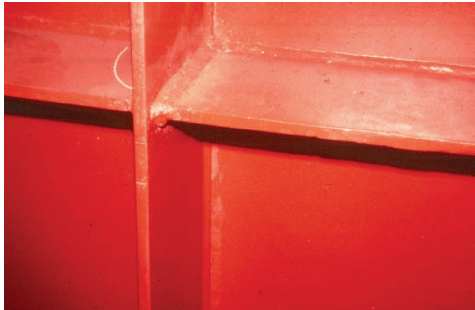
Figure 8.3.21 Intersecting Welds
