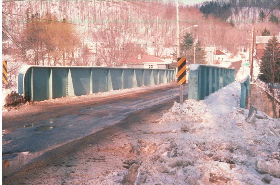
Figure 8.3.2 Through Girder Bridge
