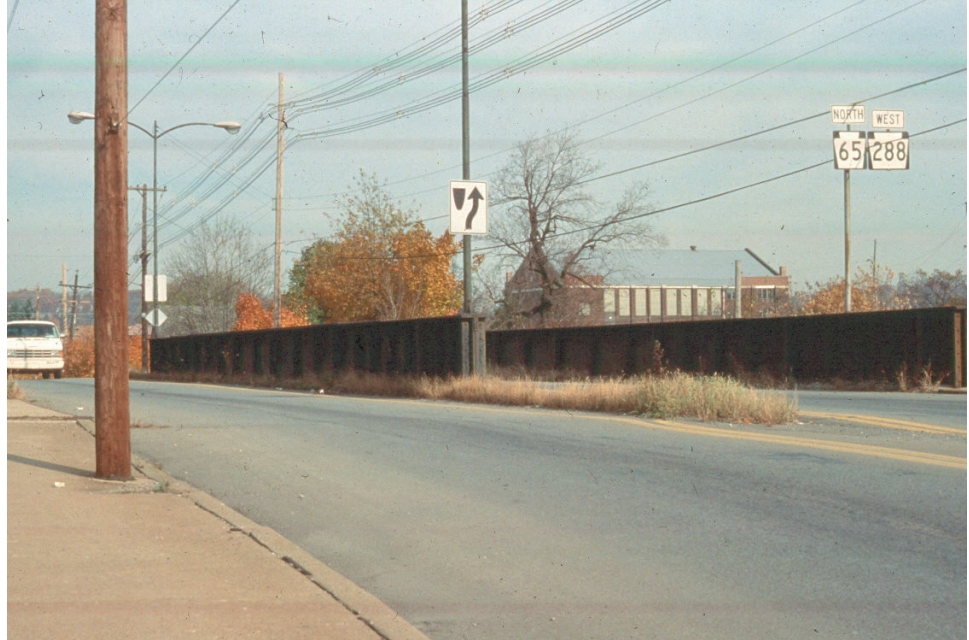
Figure 8.3.4 Through Girder Bridge with Three Girders
