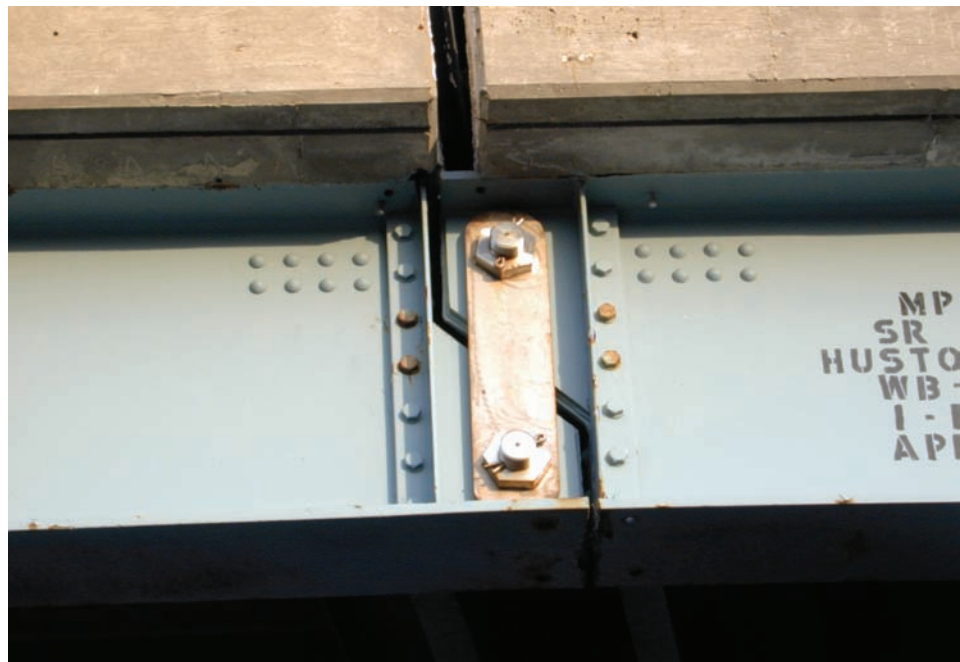
Figure 8.4.25 Stainless Steel Pin and Hanger Assembly
