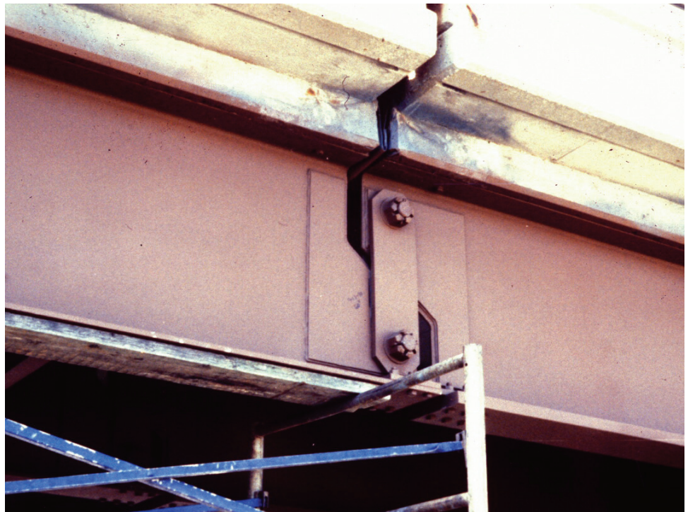
Figure 8.4.1 Typical Pin and Hanger Assembly
