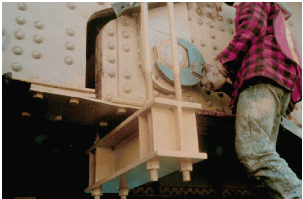
Figure 8.4.9 Retaining Nut
