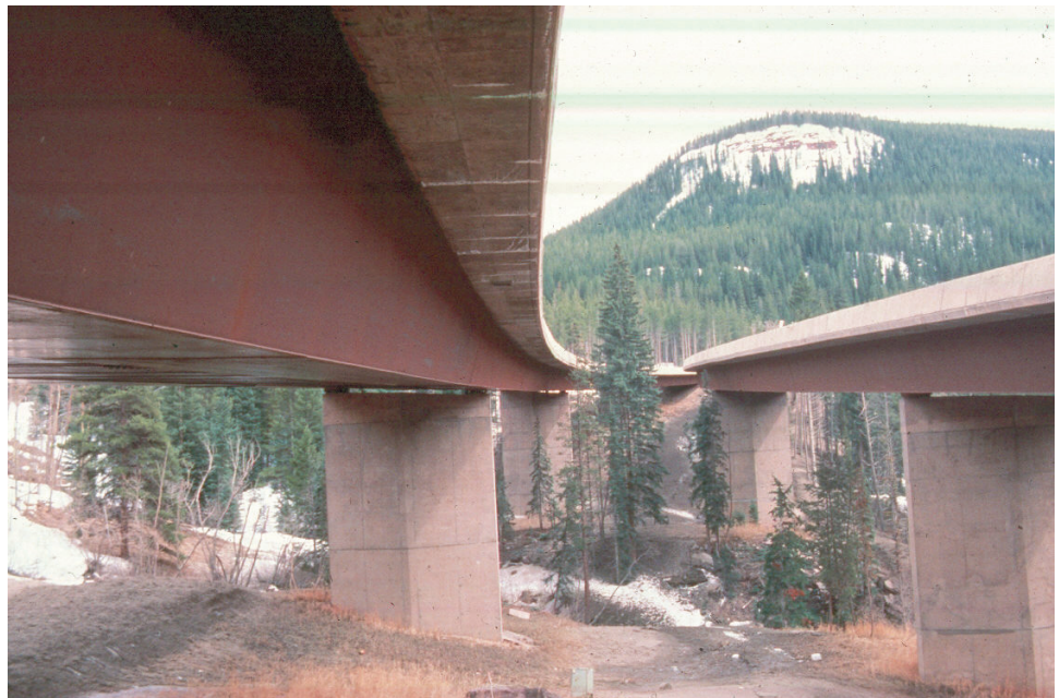
Figure 8.5.2 Curved Box Girder Bridge
