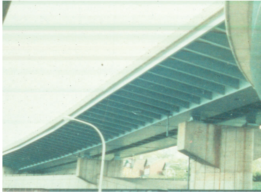
Figure 8.5.14 Non-redundant Box Girder Bridge
