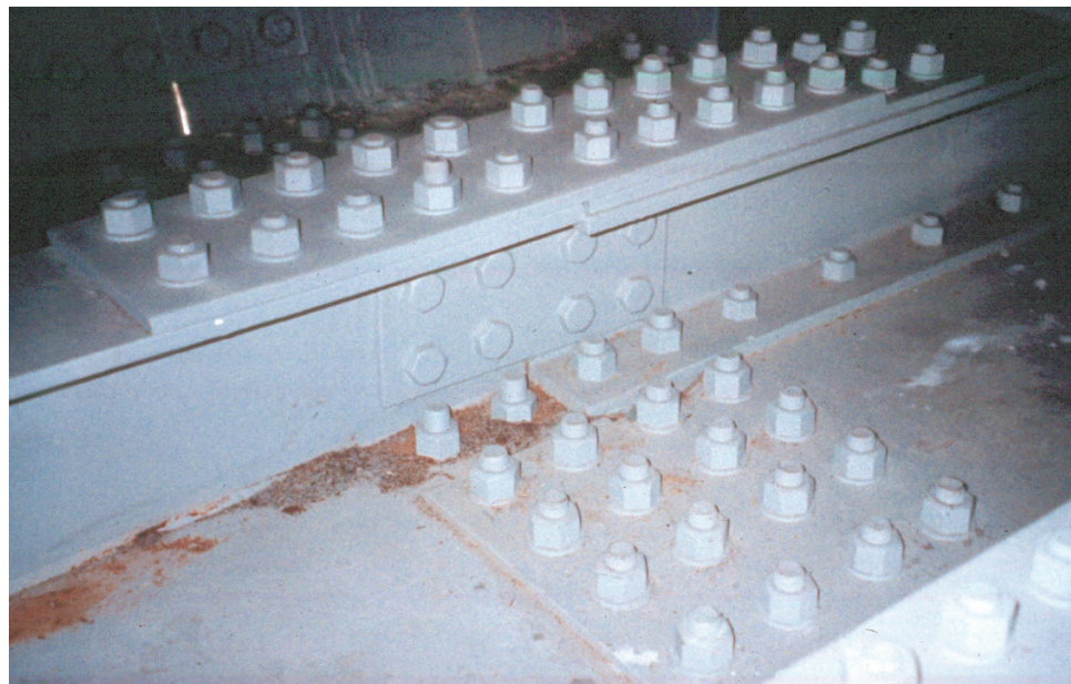
Figure 8.5.12 Field Splice
