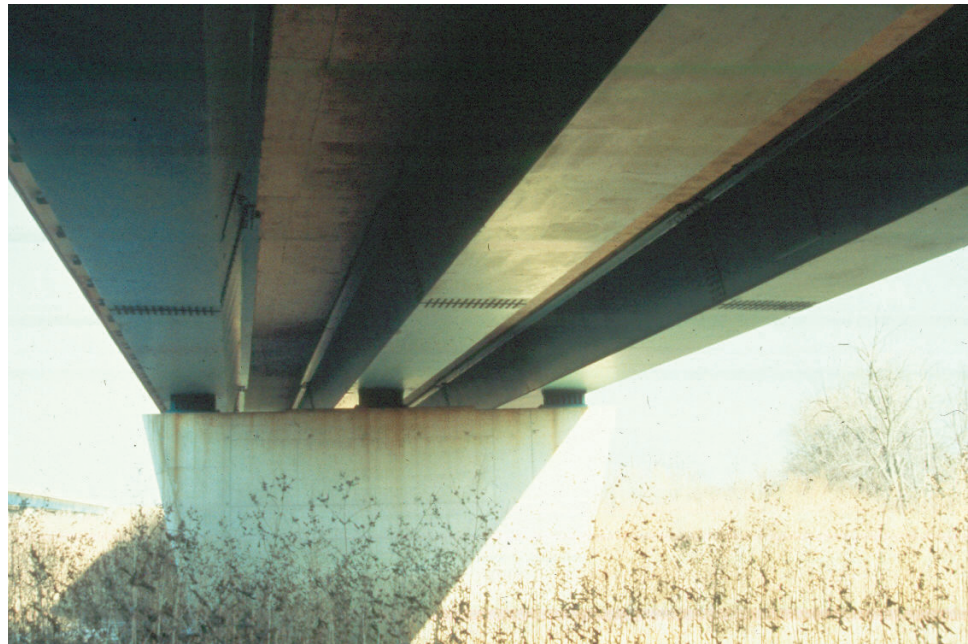
Figure 8.5.15 Redundant Box Girder Bridge
