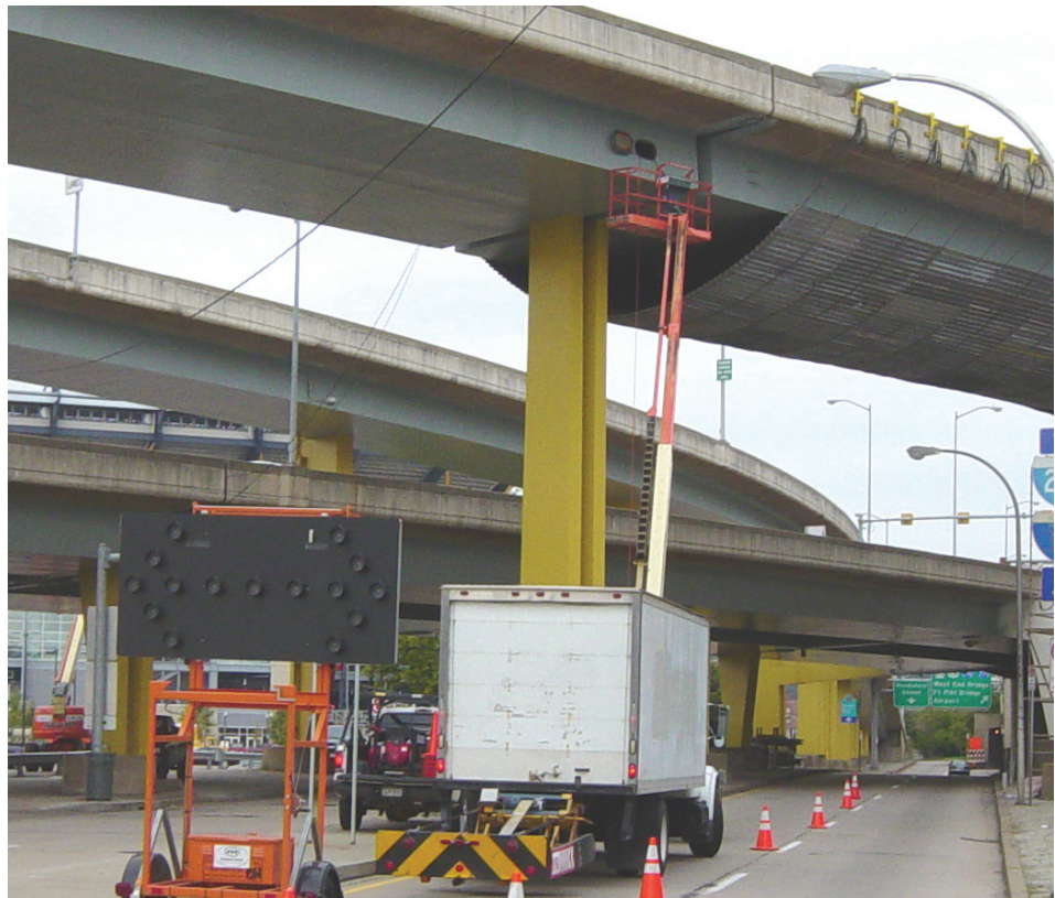
Figure 8.5.7 Box Girder Access Door
