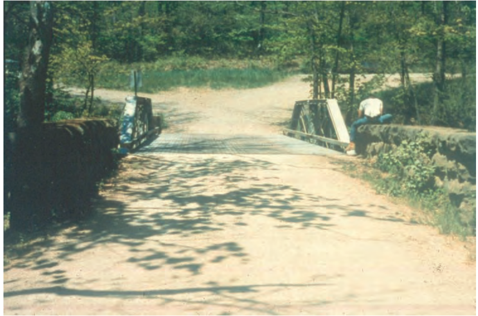
Figure 8.6.4 Pony Truss
