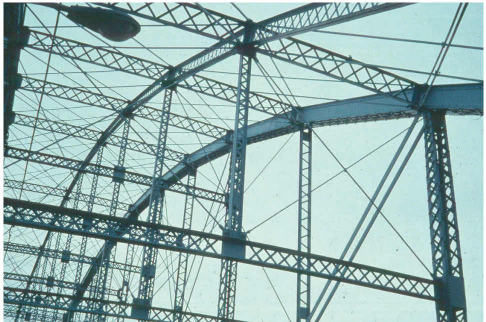
Figure 8.6.39 Sway Bracing
