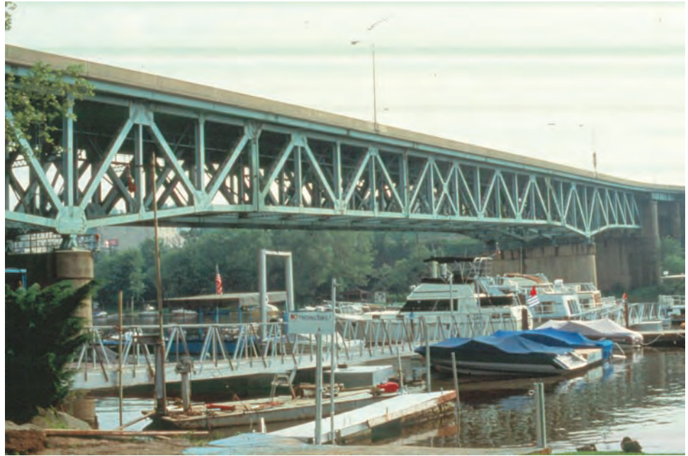
Figure 8.6.16 Cantilever Deck Truss
