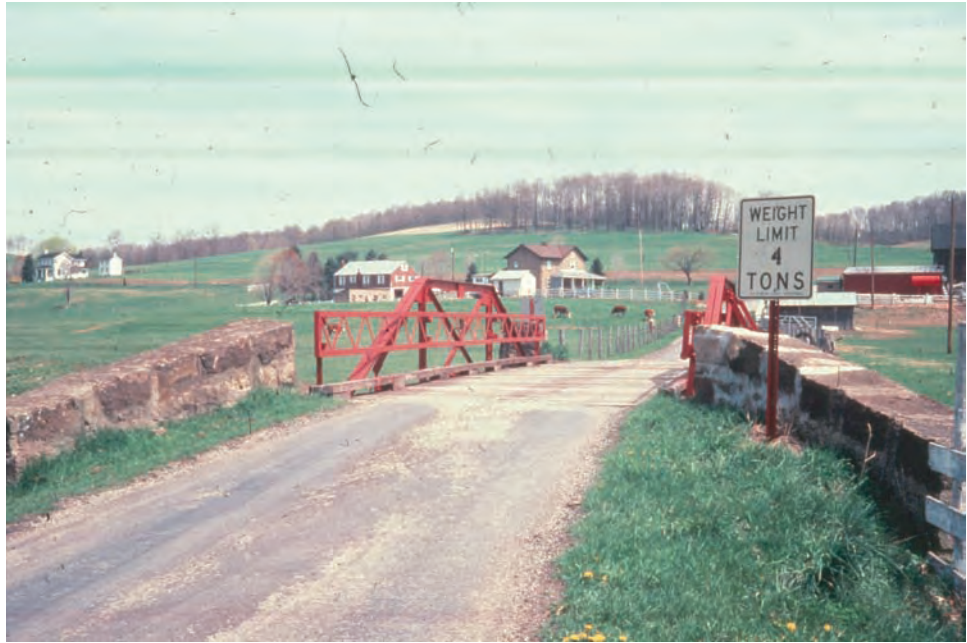
Figure 8.6.10 Single Span Pony Truss
