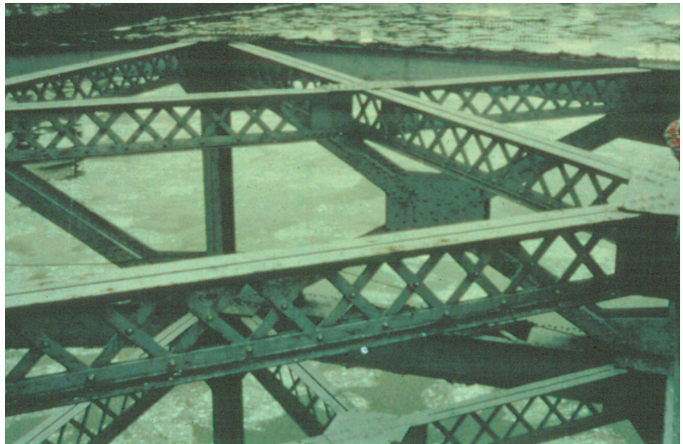
Figure 8.6.35 Upper Lateral Bracing
