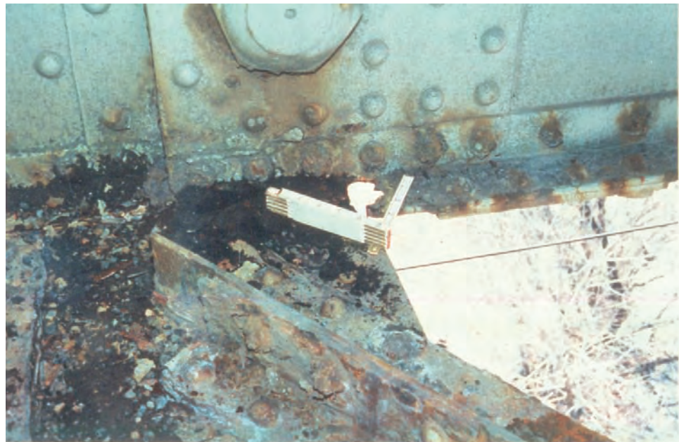
Figure 8.6.37 Lateral Bracing Gusset Plate and Lateral Bracing
