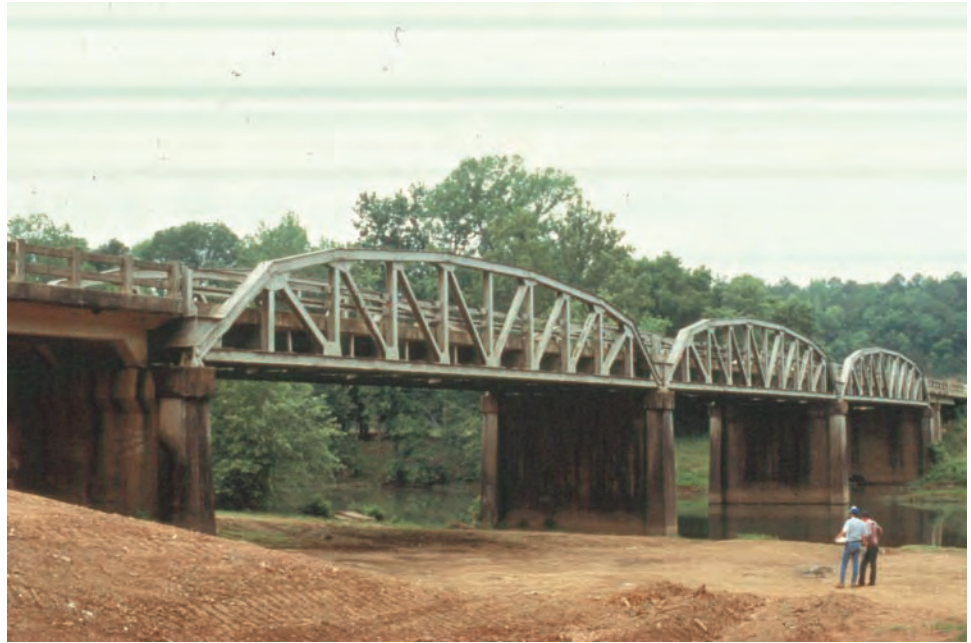
Figure 8.6.12 Multiple Span Pony Truss
