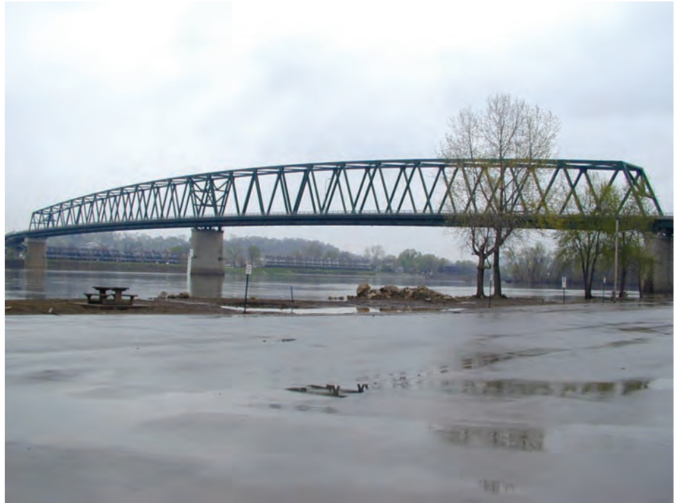
Figure 8.6.23 Continuous Through Truss
