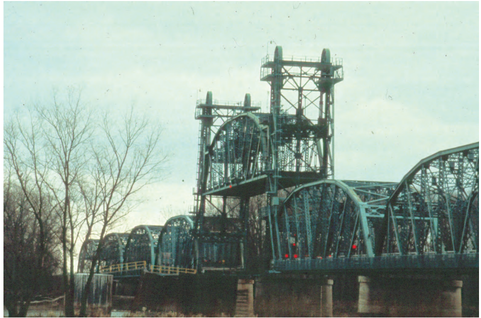
Figure 8.6.8 Vertical Lift Bridge
