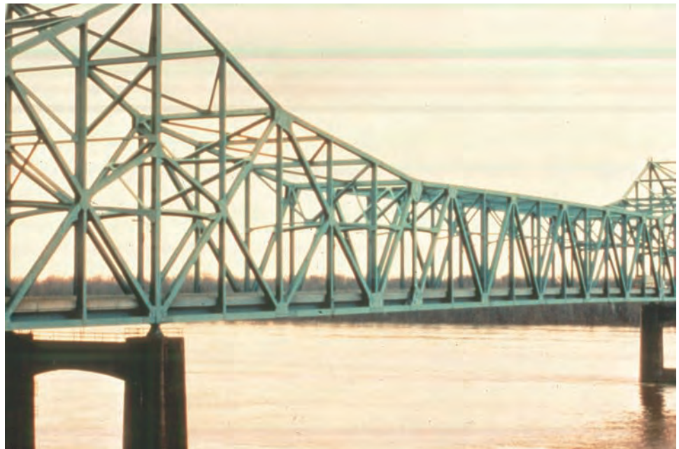
Figure 8.6.17 Cantilever Through Truss
