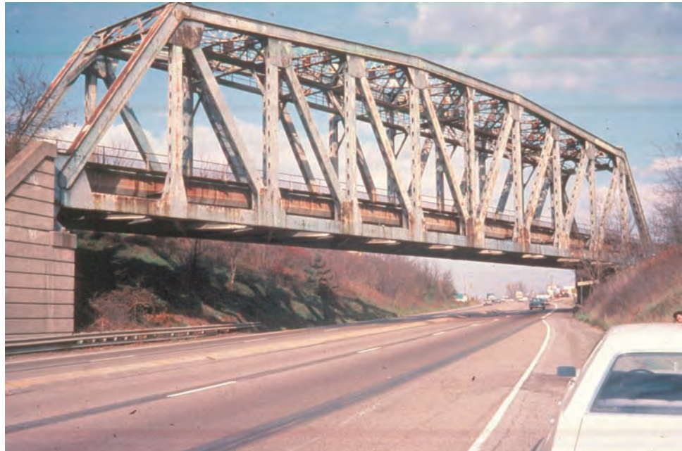
Figure 8.6.22 Single Span Through Truss – General Elevation View
