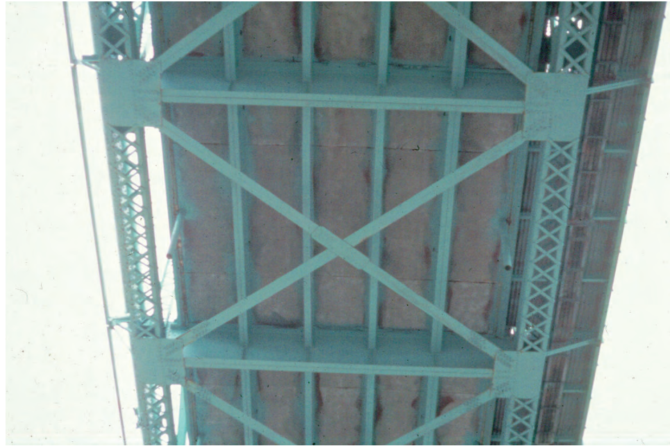
Figure 8.6.36 Lower Lateral Bracing
