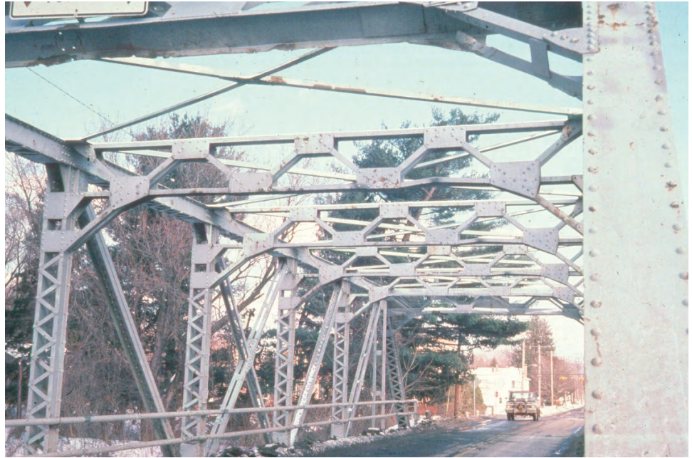
Figure 8.6.38 Sway Bracing
