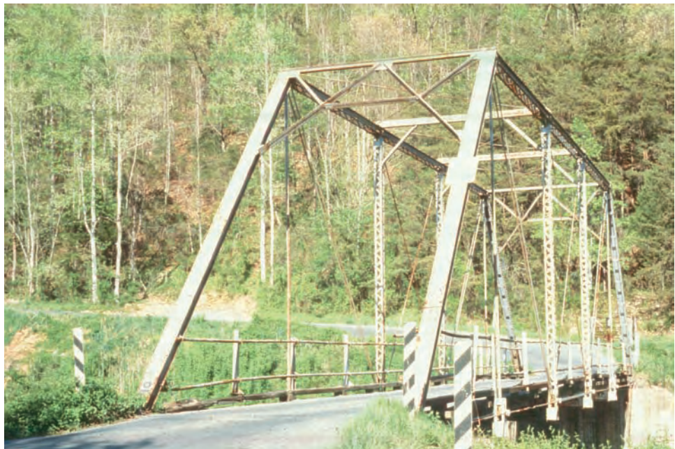
Figure 8.6.11 Single Span Through Truss
