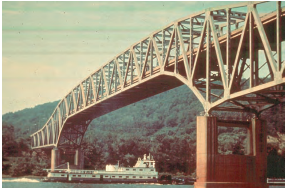
Figure 8.6.3 Through Truss
