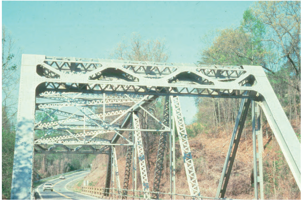
Figure 8.6.40 Portal Bracing
