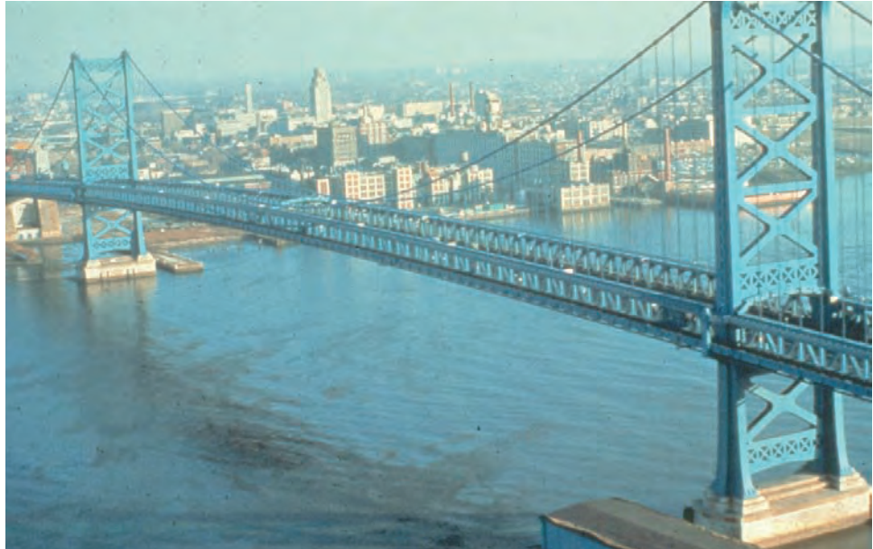
Figure 8.6.6 Suspension Bridge with Stiffening Truss
