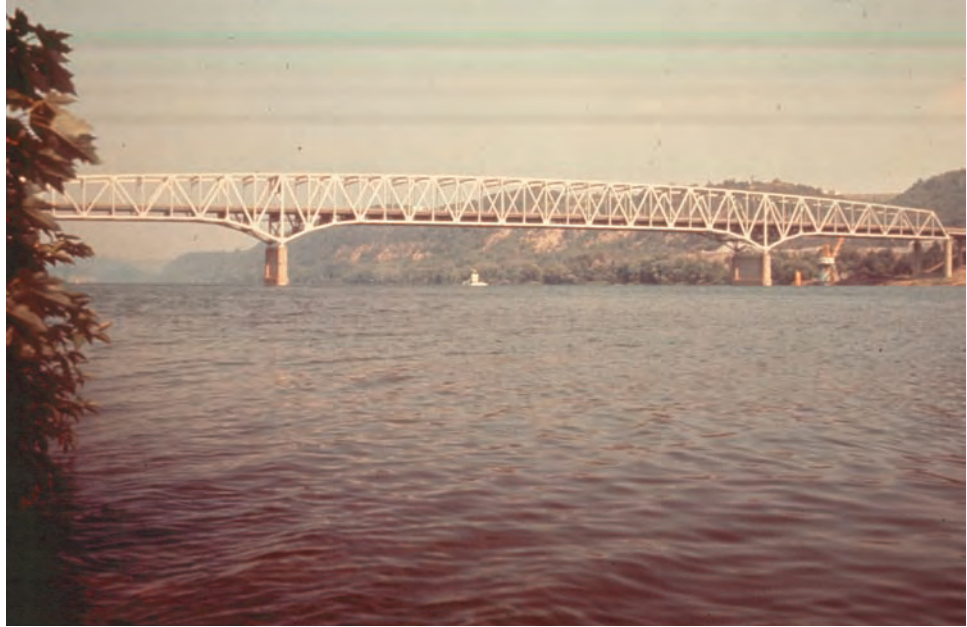
Figure 8.6.14 Continuous Through Truss
