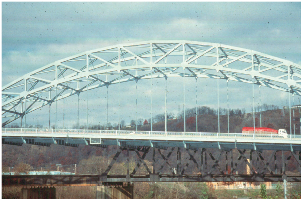
Figure 8.6.7 Arch Bridge with Stiffening Truss
