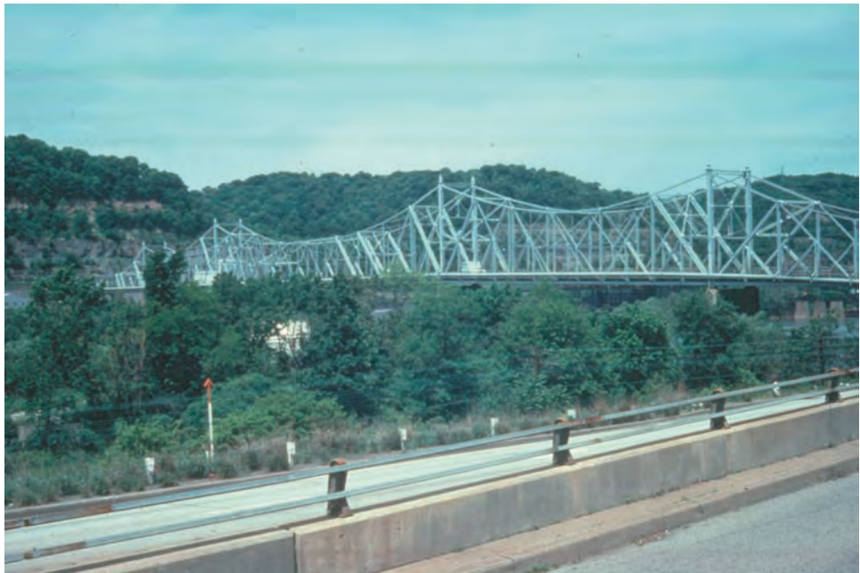
Figure 8.6.15 Cantilever Through Truss
