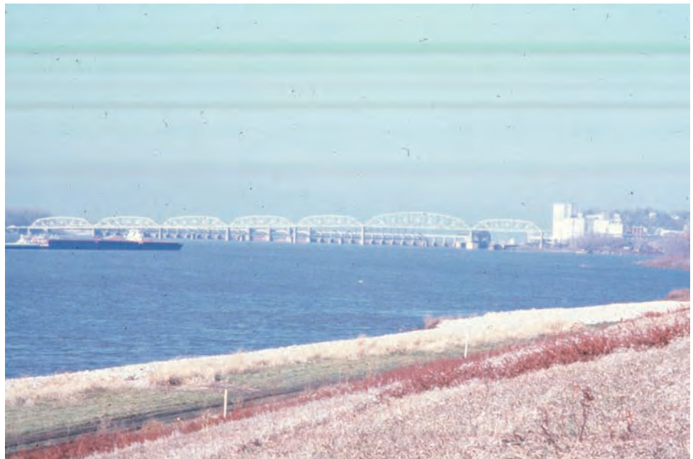
Figure 8.6.13 Multiple Span Through Truss
