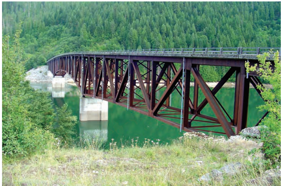
Figure 8.6.5 Deck Truss
