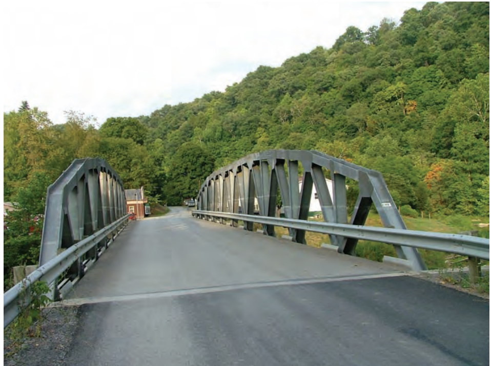
Figure 8.6.1 Single Span Truss
