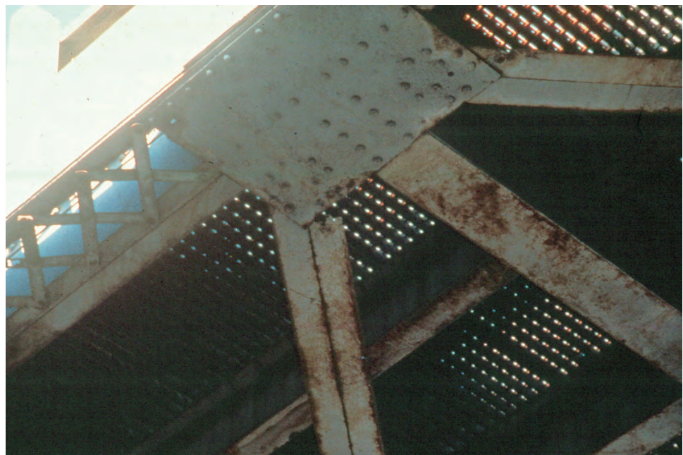
Figure 8.6.65 Lateral Bracing
