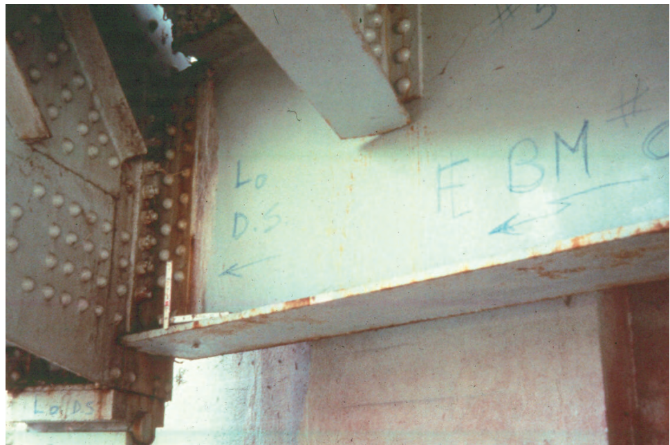
Figure 8.6.59 Clip Angles at Floorbeam and Stringer Connections
