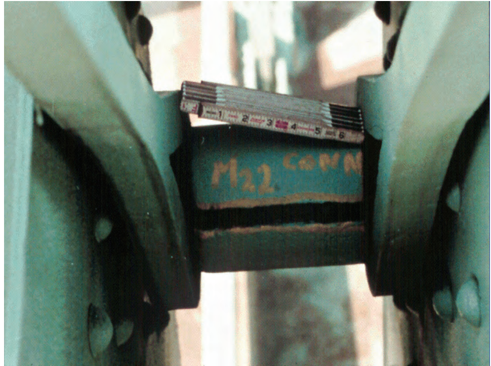
Figure 8.7.17 Steel Pin Spacer or Filling Ring
