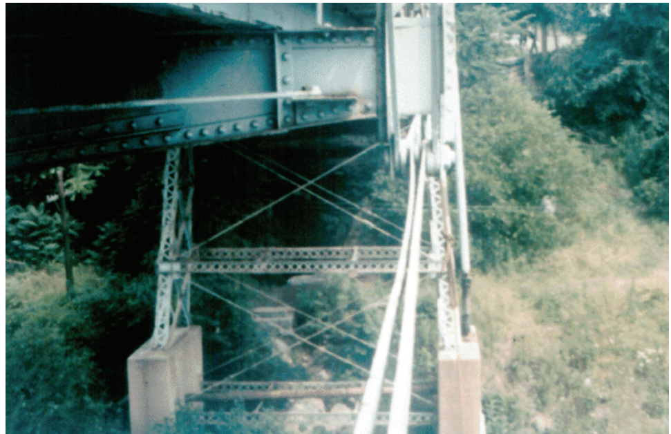
Figure 8.7.22 Non-parallel Eyebar Member
