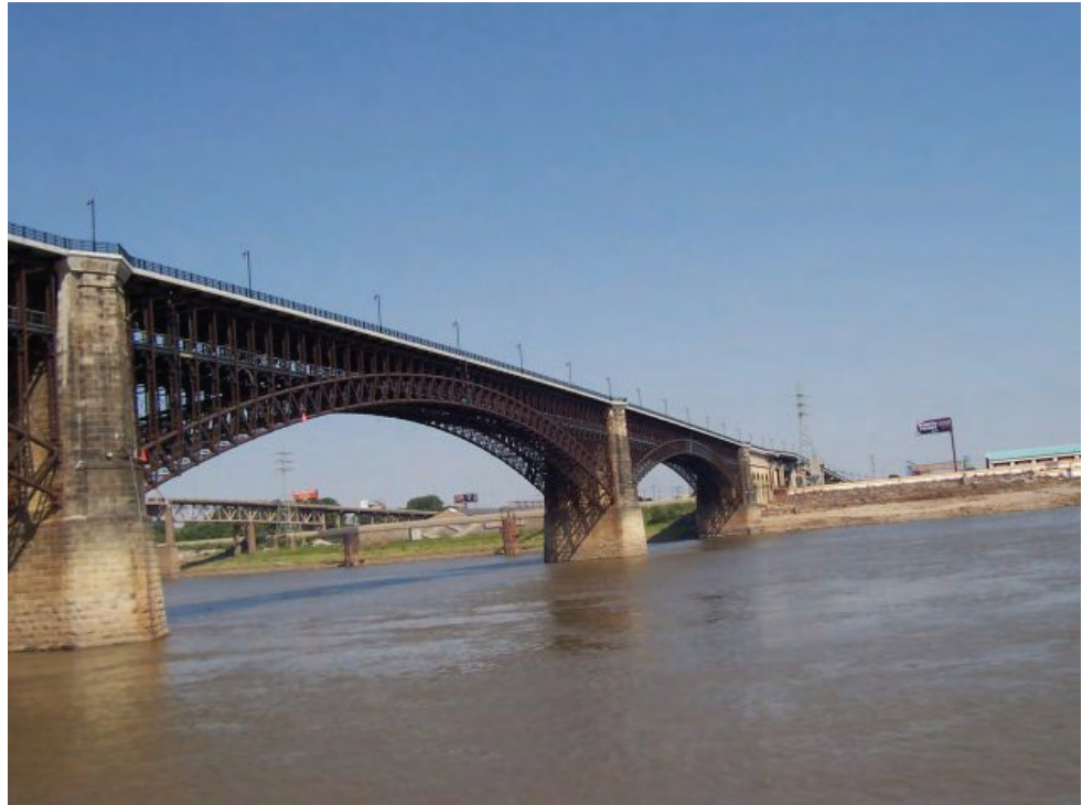
Figure 8.7.9 Eads Bridge, St. Louis
