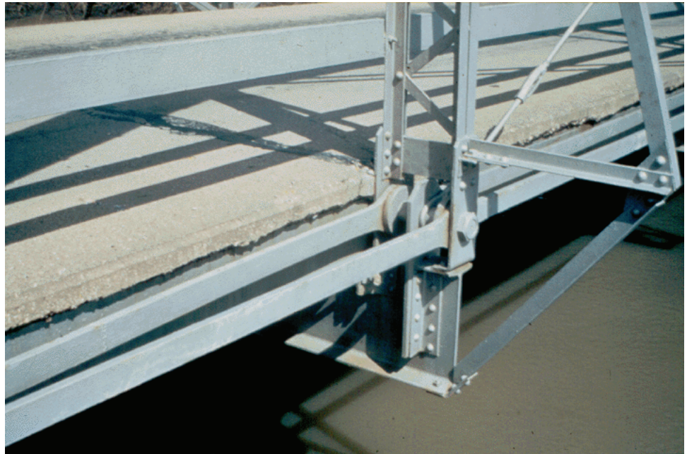
Figure 8.7.1 Typical Eyebar Tension Member on a Truss
