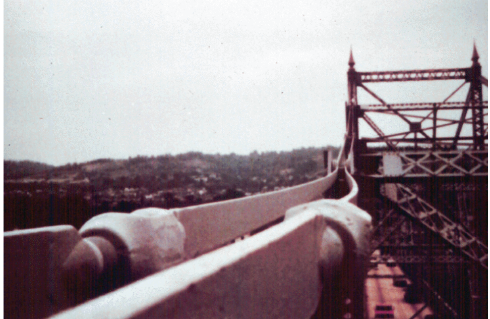
Figure 8.7.20 Bowed Eyebar Member
