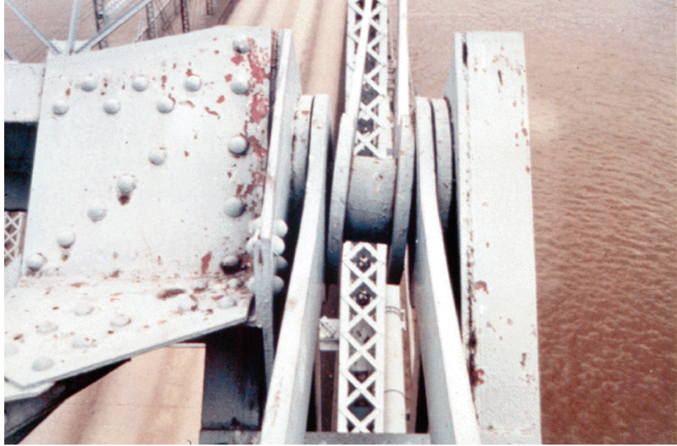
Figure 8.7.24 Symmetry at an Eyebars Connection
