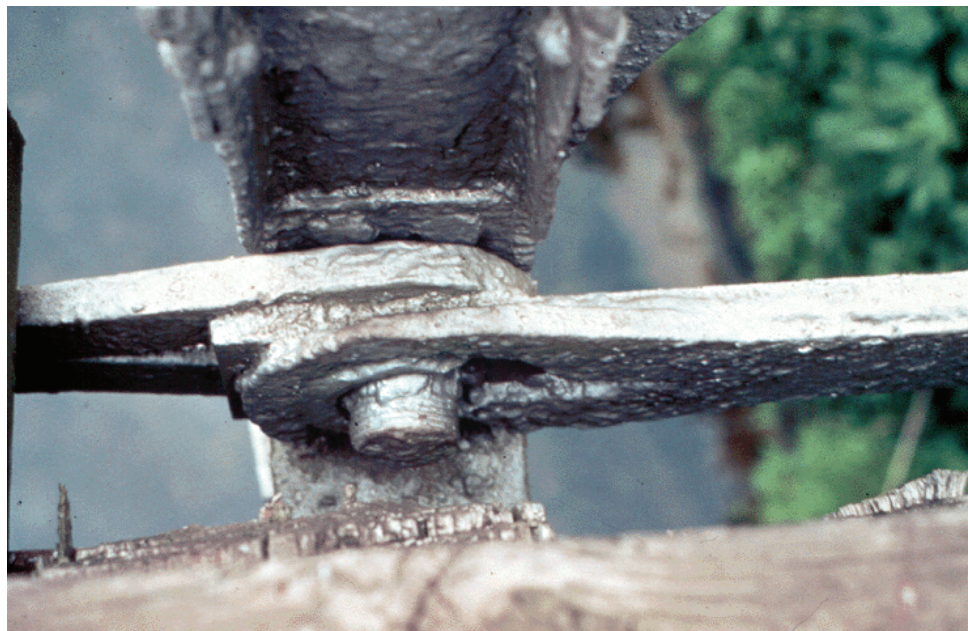
Figure 8.7.27 Welded Repair to Loop Rods
