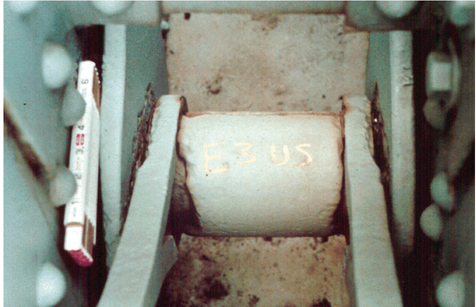
Figure 8.7.23 Corroded Spacer
