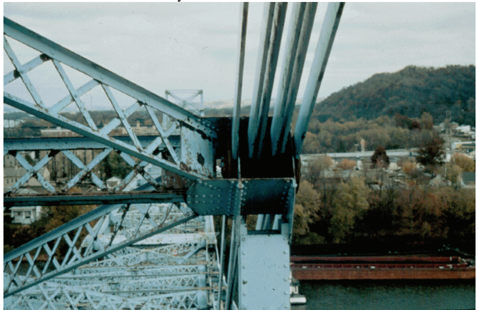
Figure 8.7.32 Fracture Critical Top Chord Truss Member: Internally Redundant Eyebar
