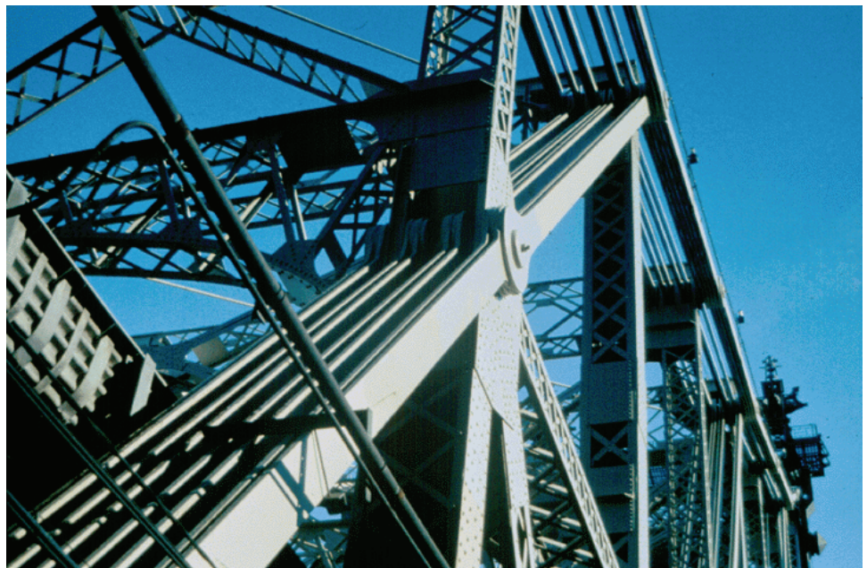
Figure 8.7.2 Eyebar Cantilevered Truss Bridge (Queensboro Bridge, NYC)
