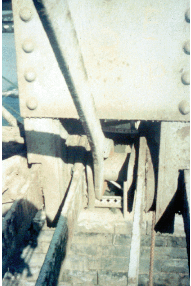
Figure 8.7.18 Nonredundant Eyebar Member
