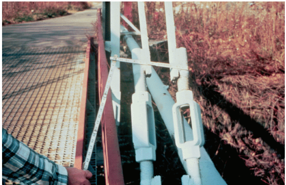
Figure 8.7.29 Welded Repair to Turnbuckles
