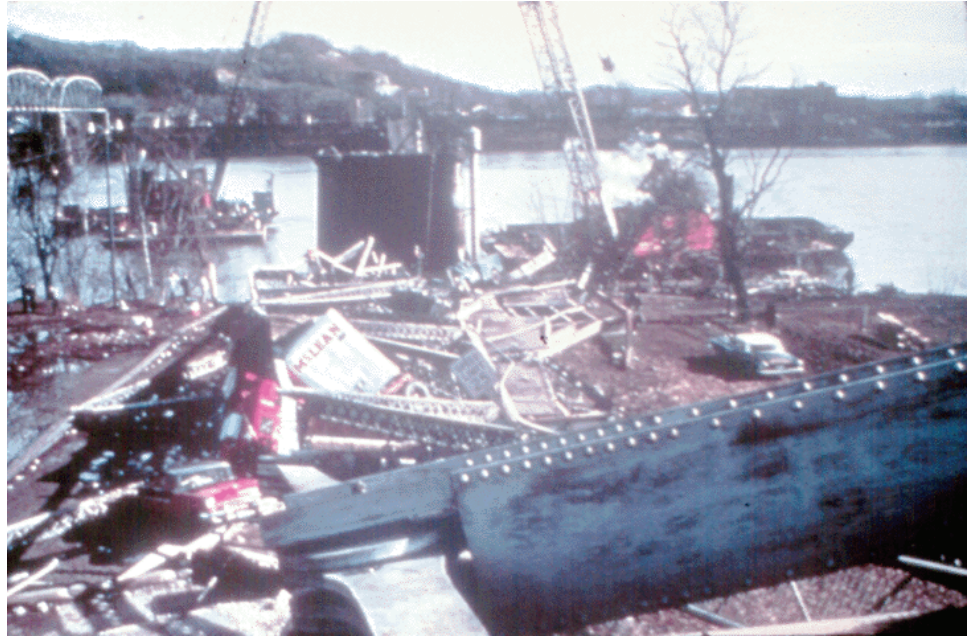
Figure 8.7.5 Collapsed Silver Bridge
