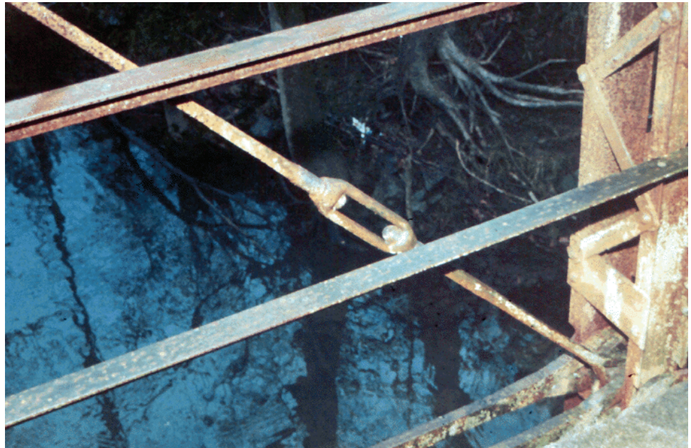
Figure 8.7.28 Turnbuckle on a Truss Diagonal
