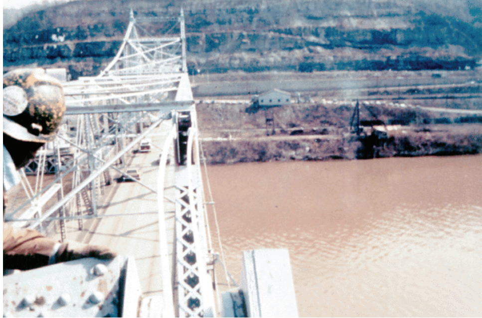
Figure 8.7.6 Inspection of Eyebars
