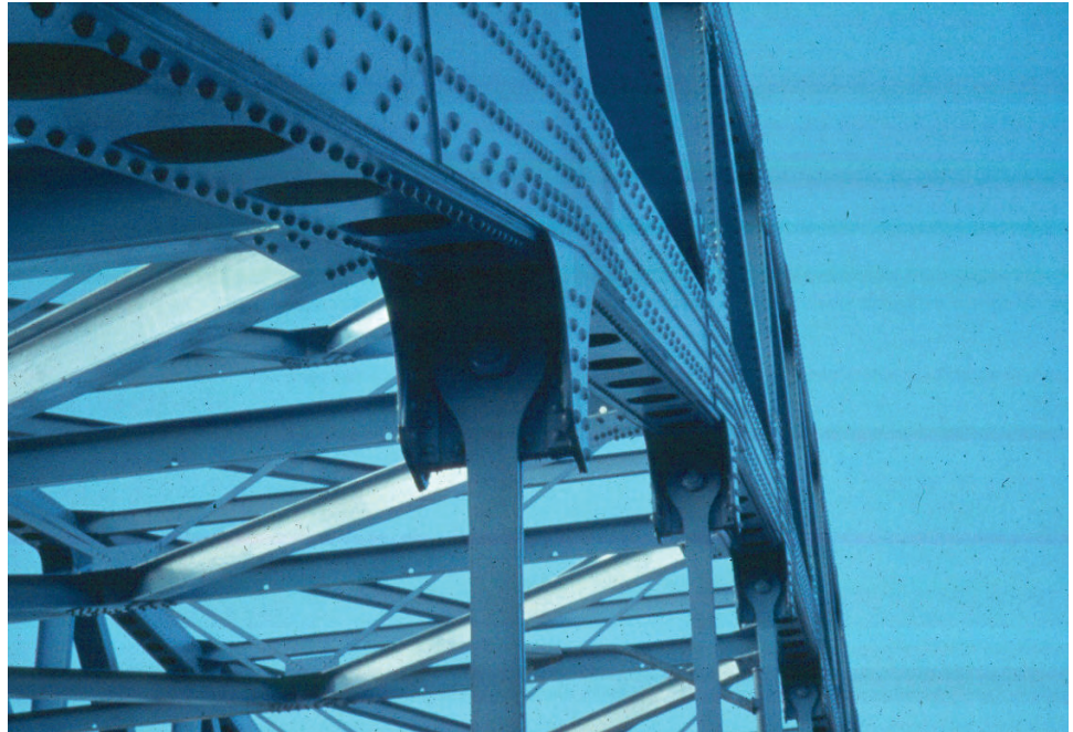
Figure 8.8.19 Hanger Connection on a Through Arch
