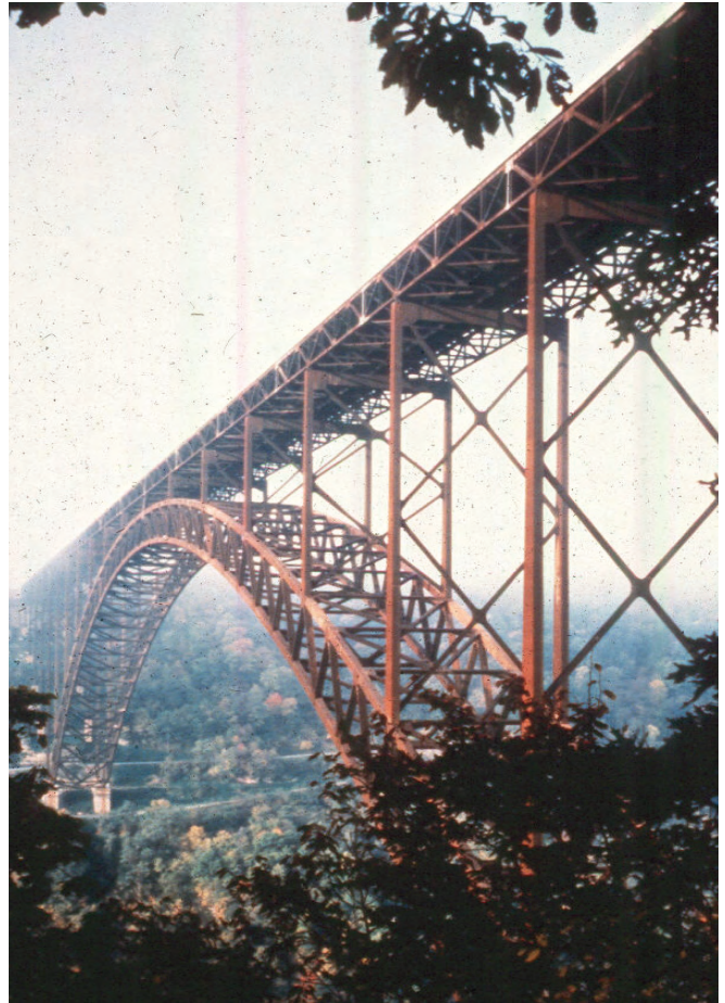
Figure 8.8.6 Braced Rib Deck Arch, New River Gorge, WV
