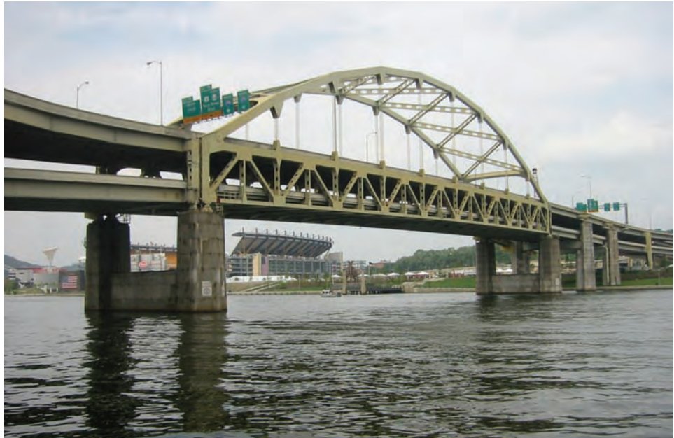
Figure 8.8.3 Tied Arch Bridge
