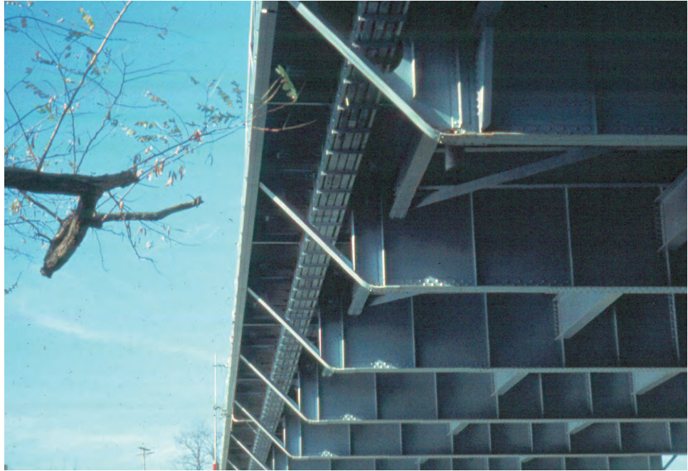
Figure 8.8.21 Floor System on a Through Arch
