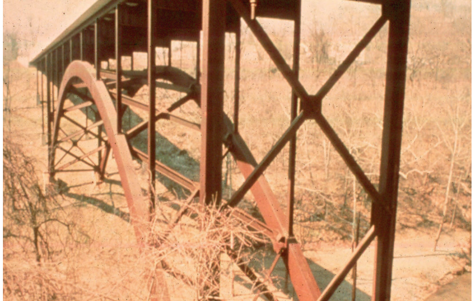
Figure 8.8.18 Solid Ribbed Deck Arch Showing Spandrel Columns
