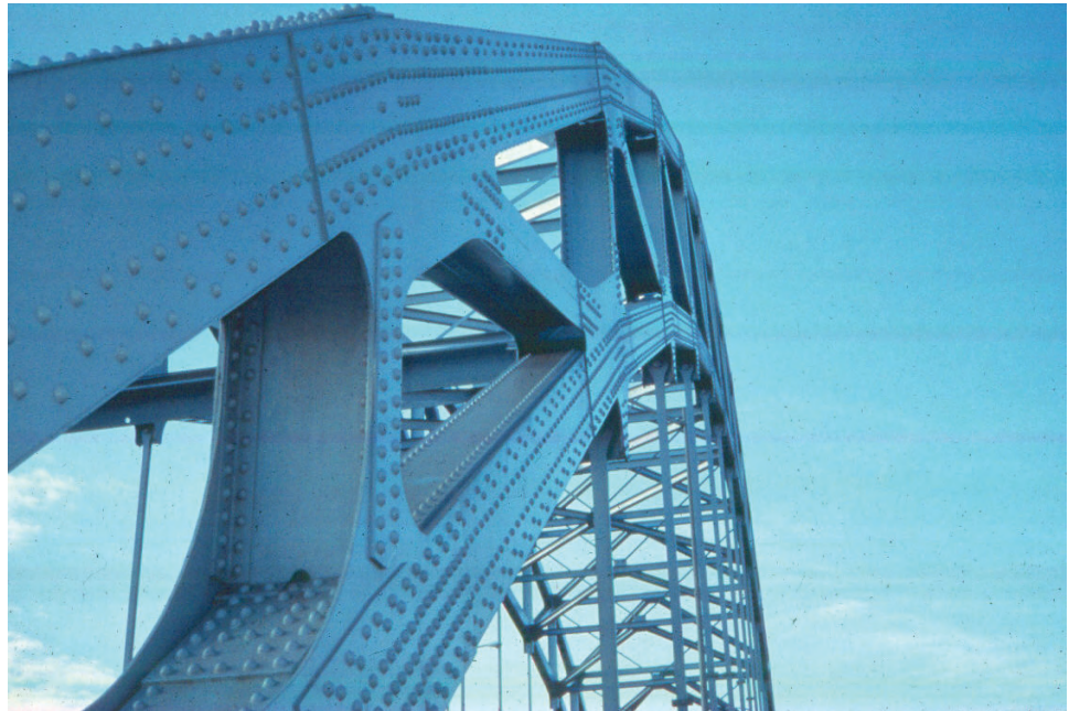
Figure 8.8.17 Through Truss Arch Members
