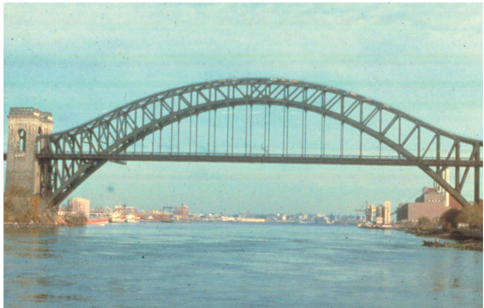
Figure 8.8.2 Through Arch Bridge
