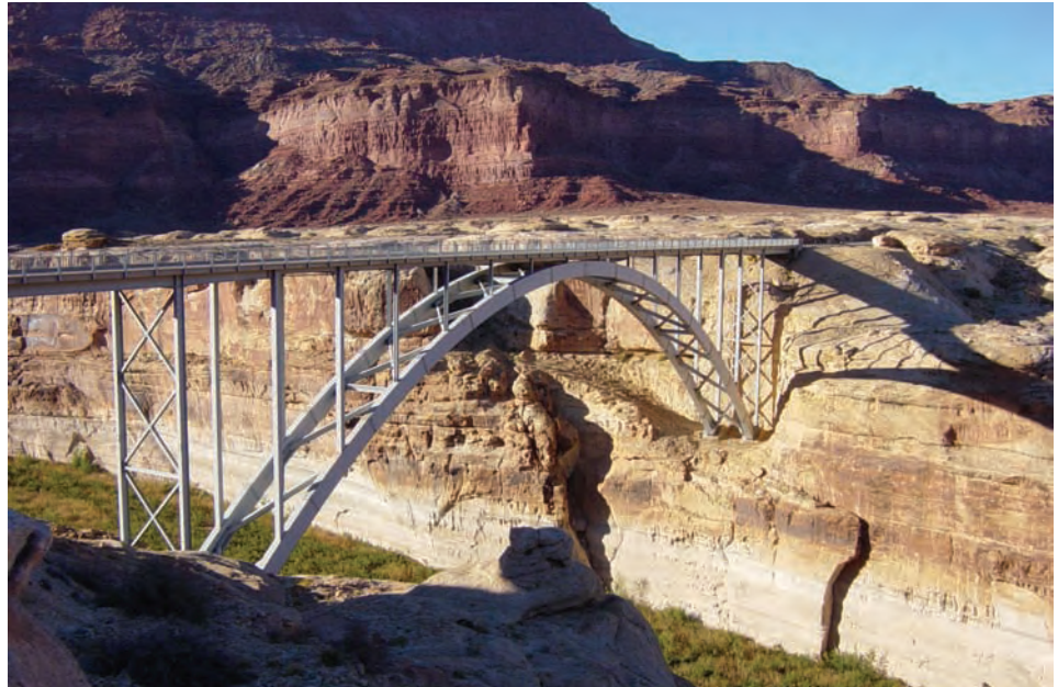
Figure 8.8.1 Deck Arch Bridge
