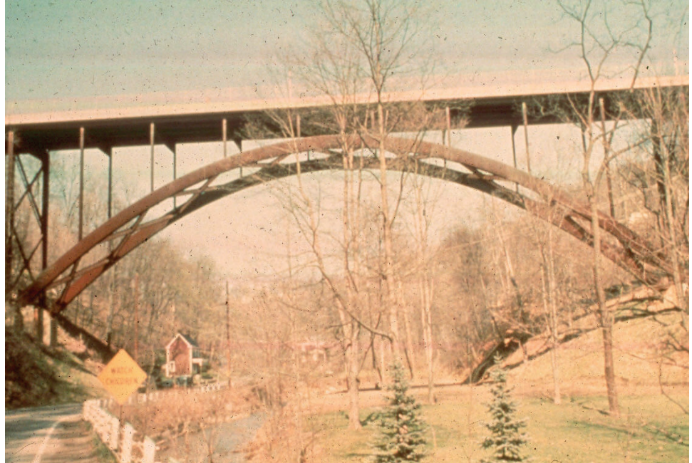
Figure 8.8.5 Solid Ribbed Deck Arch
