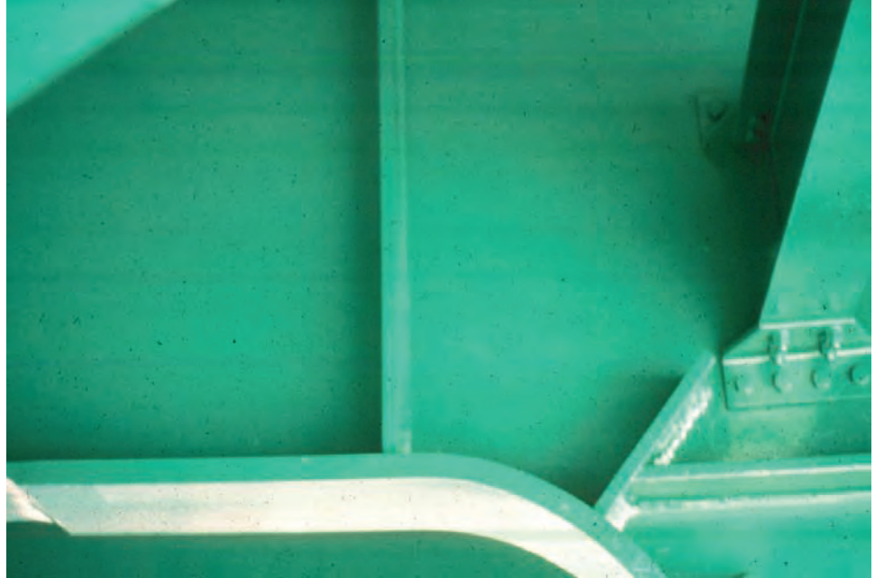
Figure 8.9.17 Knee Area: Fatigue Prone Details
