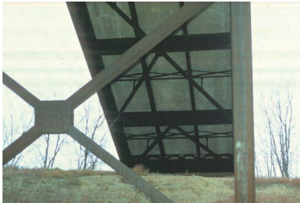
Figure 8.9.8 Two Frame Bridge with Floorbeam-Stringer Floor System
