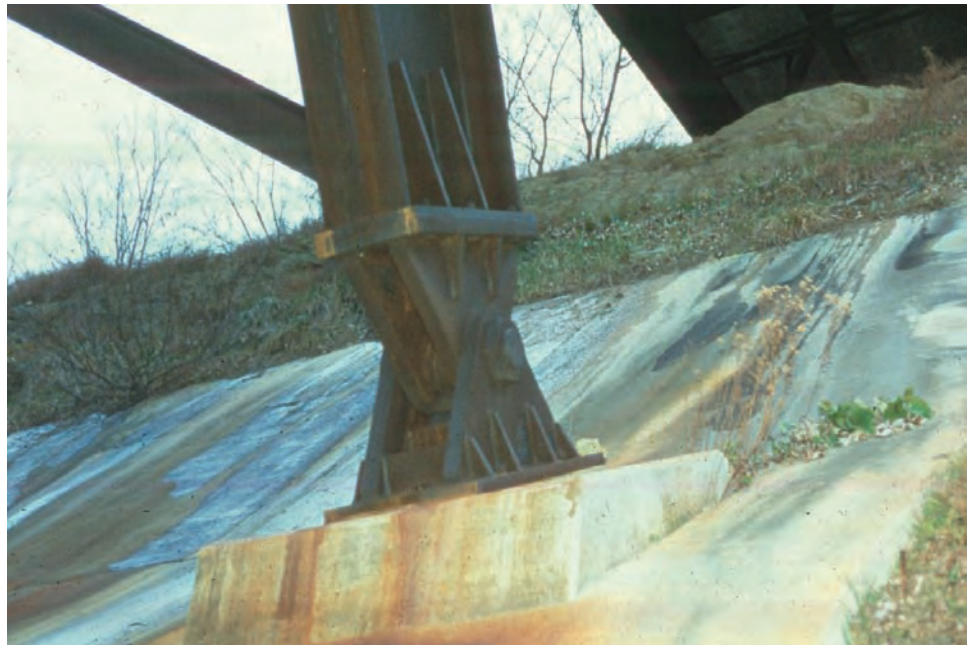
Figure 8.9.15 Bearing Area of a Two Frame Bridge
