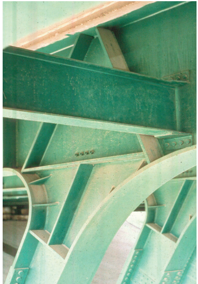
Figure 8.9.4 Connection Between Legs and Girder Portion
