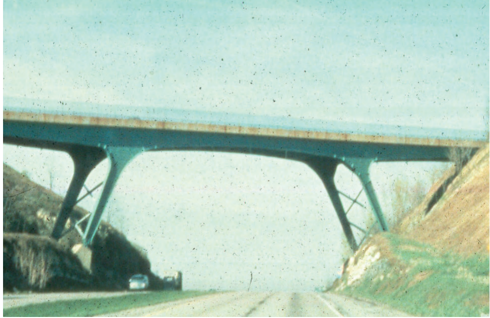
Figure 8.9.13 Dual Frame Rigid Frame – A Fracture Critical Structure
