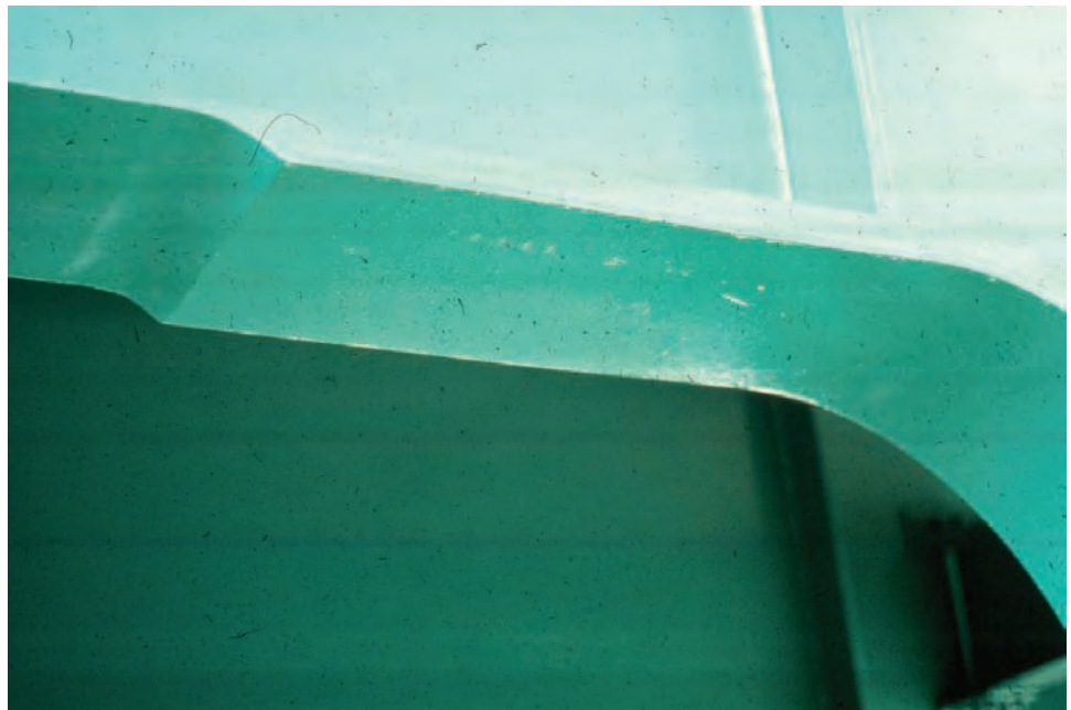
Figure 8.9.18 Welded Flange Splice
