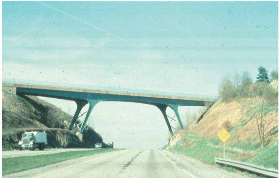
Figure 8.9.1 Typical Rigid K-frame Constructed of Two Frames
