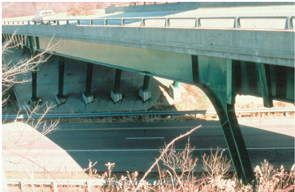
Figure 8.9.3 Typical K-frame
