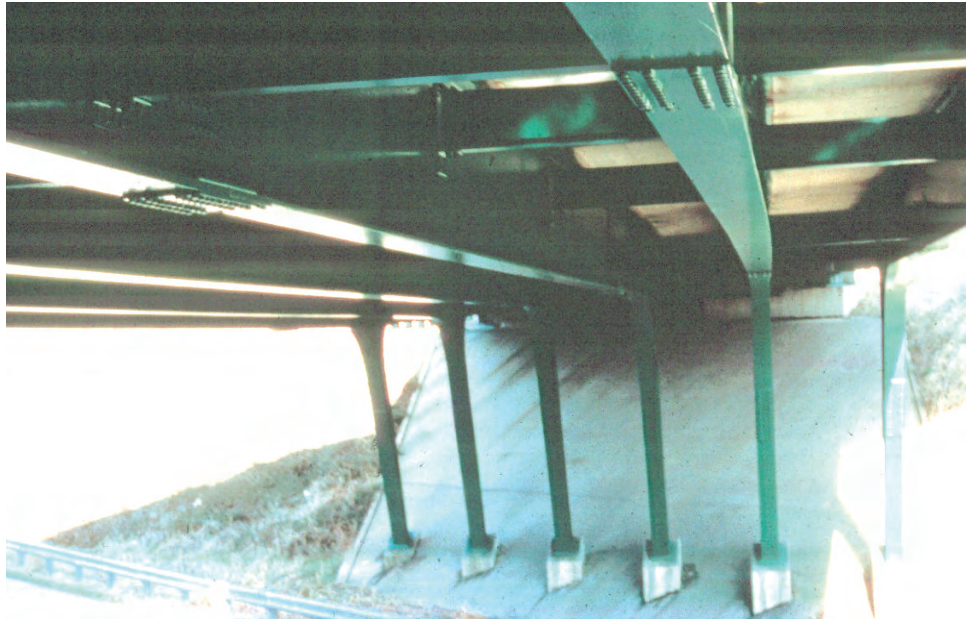
Figure 8.9.2 Typical Rigid Frame Constructed of Multiple Frames
