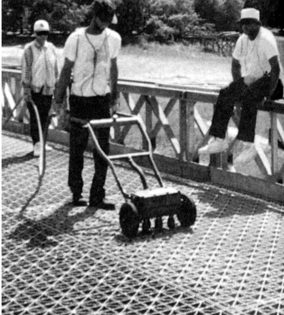
Exhibit X. 12 Scabbier Roughened Grid Deck
