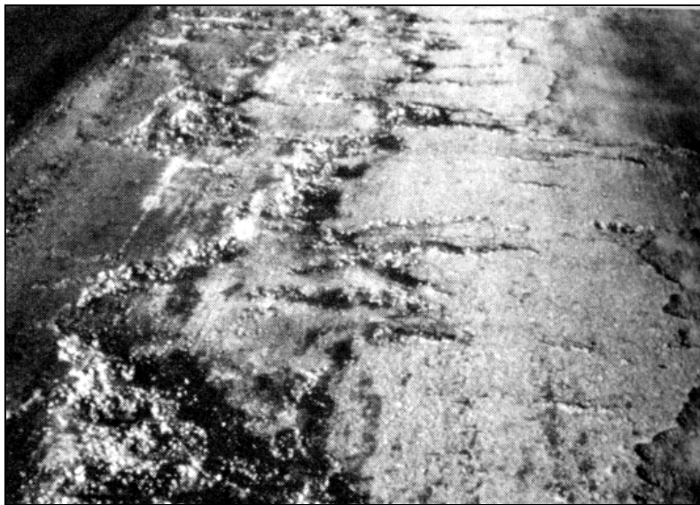
Exhibit X. 1 Deteriorated Deck
