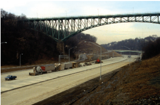
Figure 6-1. Highway embankment with fly ash structural fill.
