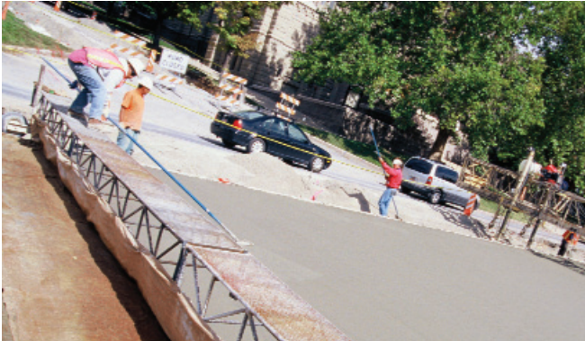
Figure 3-5. Fly ash concrete finishing
