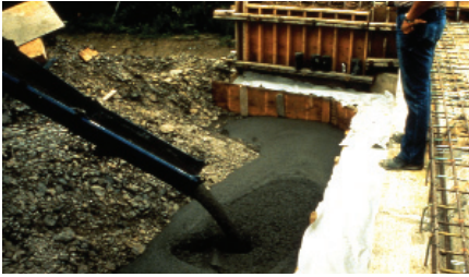
Figure 5-4. Bridge abutment backfill with flowable fill.
