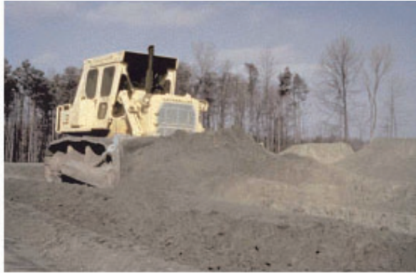
Figure 6-3. Spreading and compaction of fly ash structural fill.
