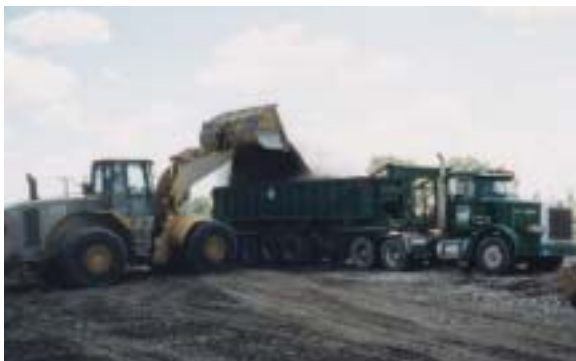
Figure 15. Supplying Foundry Sand for a road base
