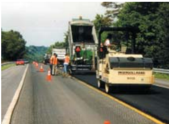
Figure 17. Construction of HMA pavement
