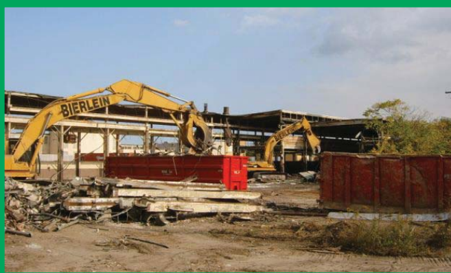
Recycling of steel at the former automotive site.
