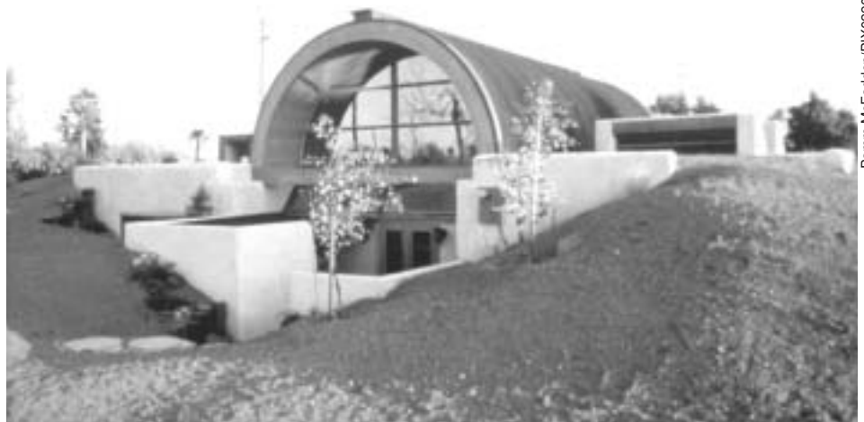
An example of an earth-sheltered building in Tempe, Arizona.
