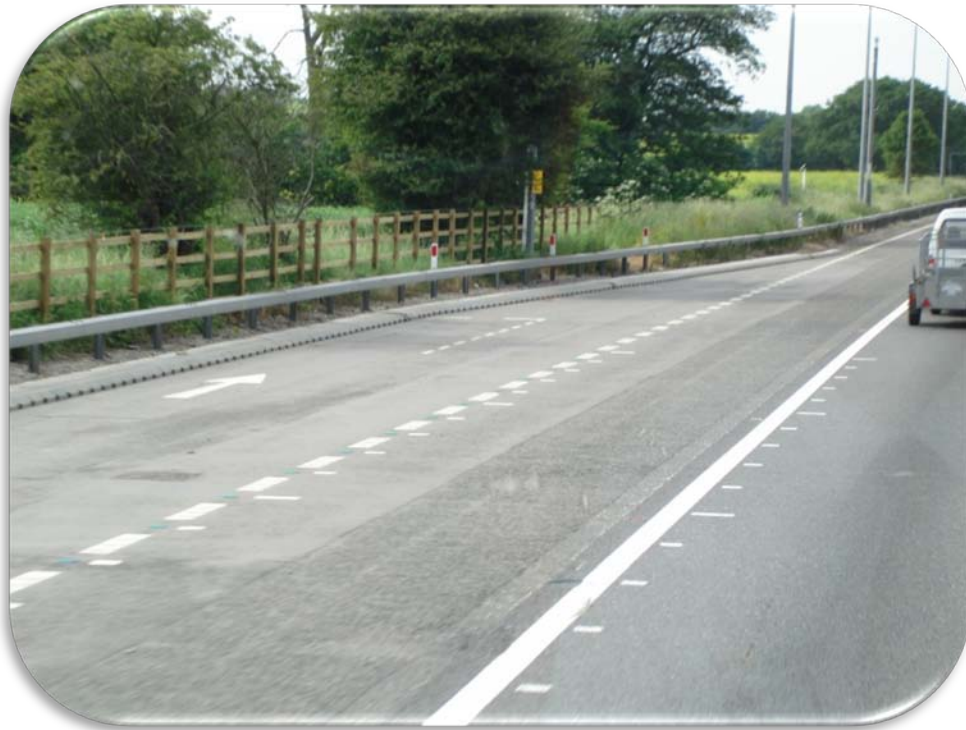
Figure 37. Photo. Emergency Refuge Area on Facility with Active Traffic Management—England.
