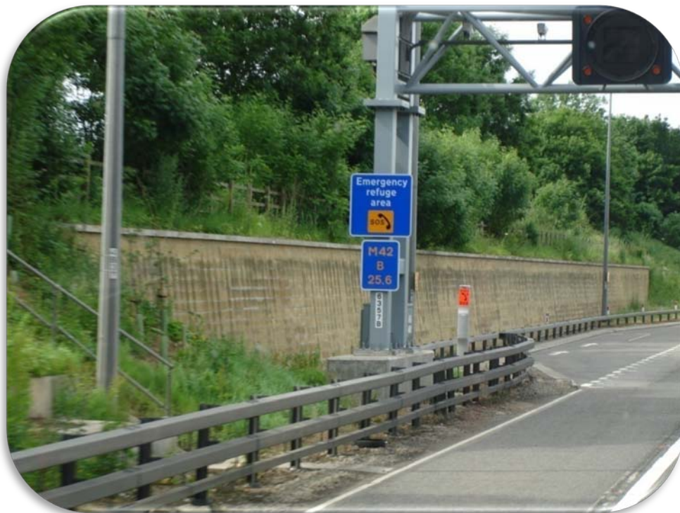
Figure 38. Photo. Emergency Call Box on Facility with Active Traffic Management—England.
