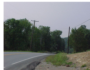
After slope flattening
