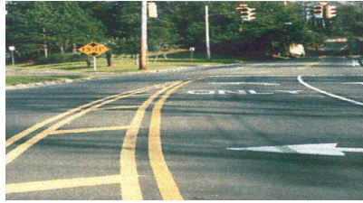
Night performance pavement markings
