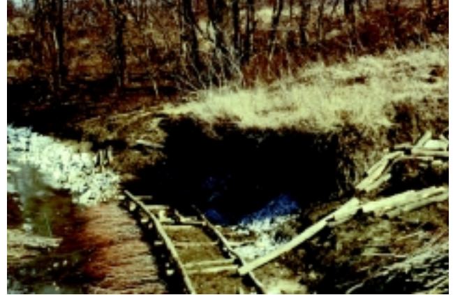
Figure 16-15b A live cribwall during installation
