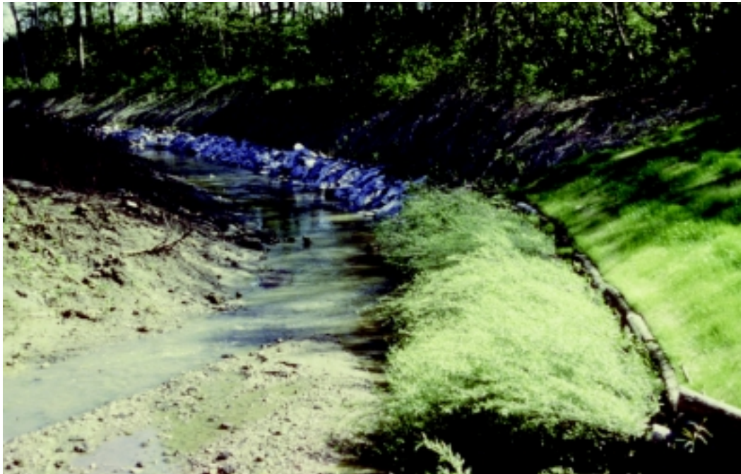
Figure 16-15c An established live cribwall system
