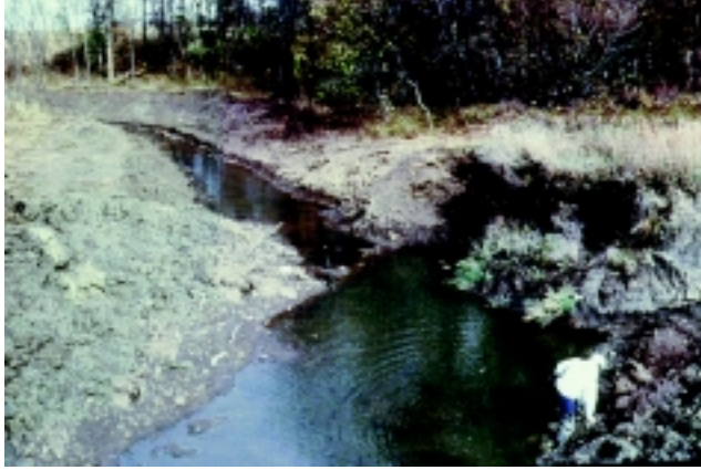
Figure 16-15a Pre-construction streambank conditions
