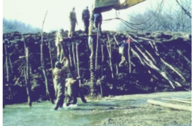
Figure 16-25b Installing dormant posts (Don Roseboom photo)
