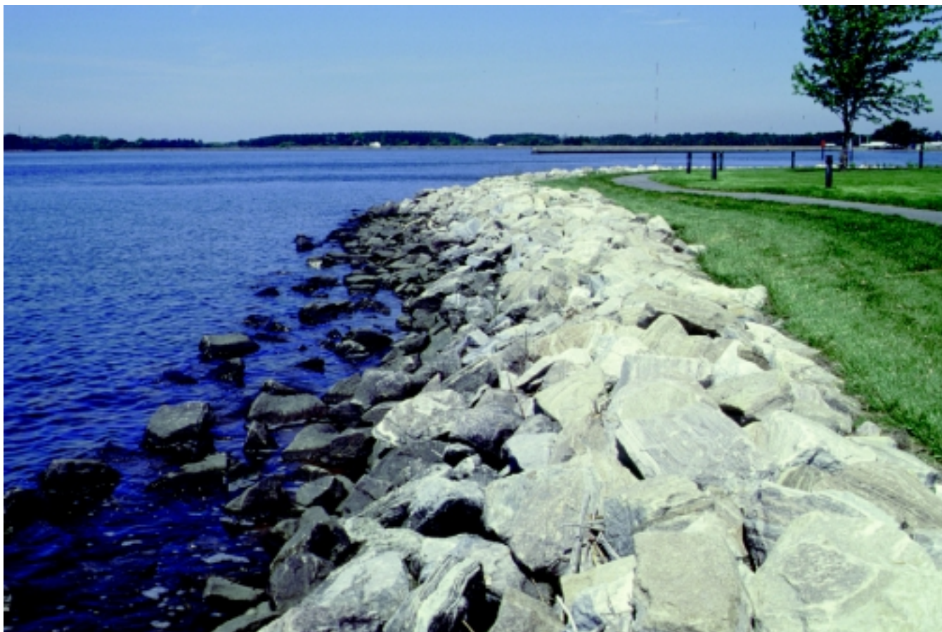
Figure 16-51 Rock riprap revetment
