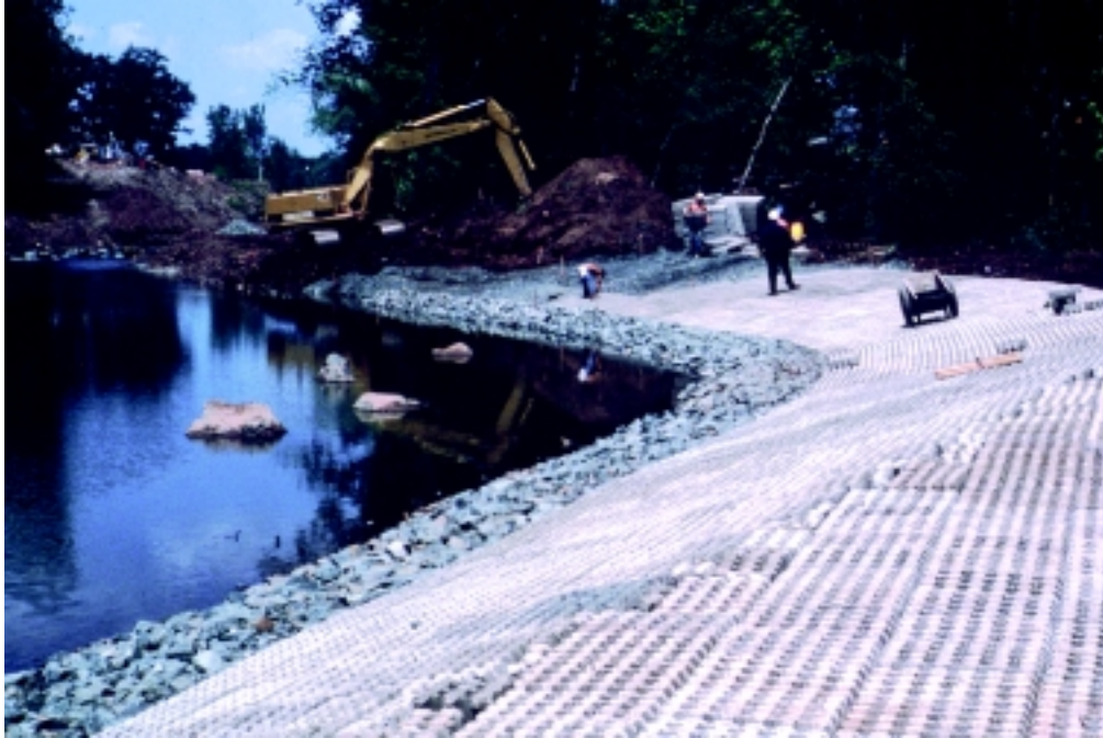
Figure 16-35a Concrete cellular block system before backfilling
