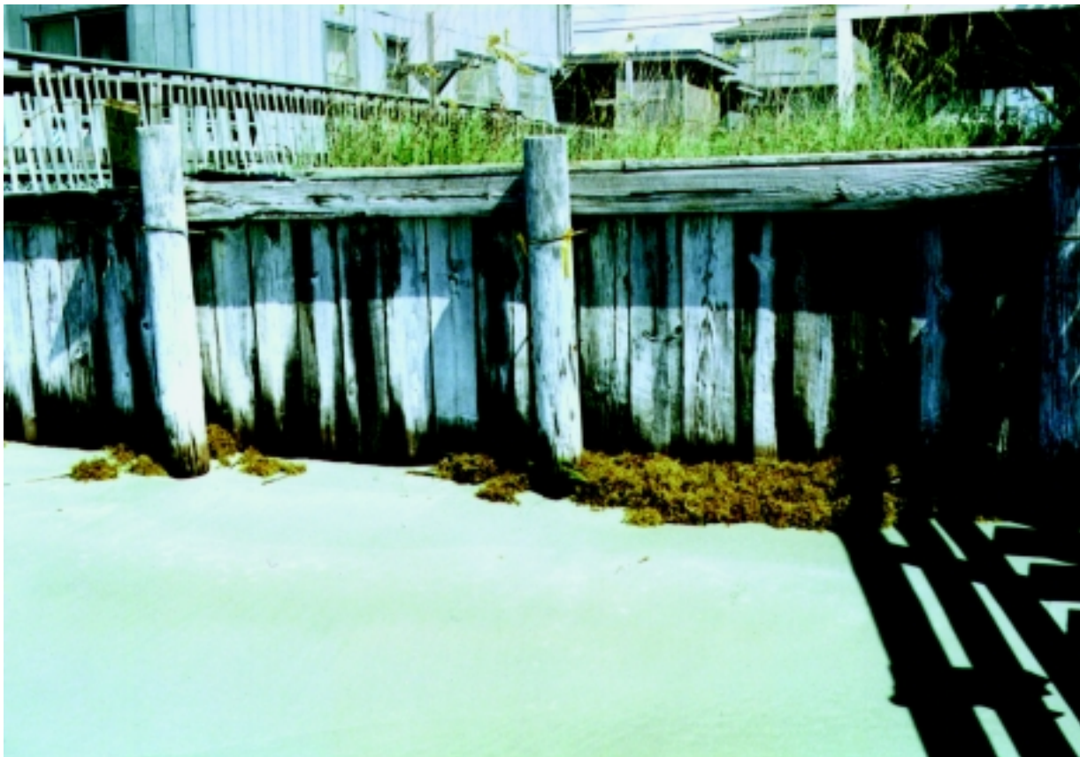
Figure 16-46 Timber bulkhead system
