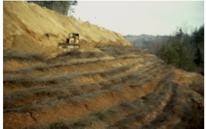
Figure 18-1b Measures being installed
