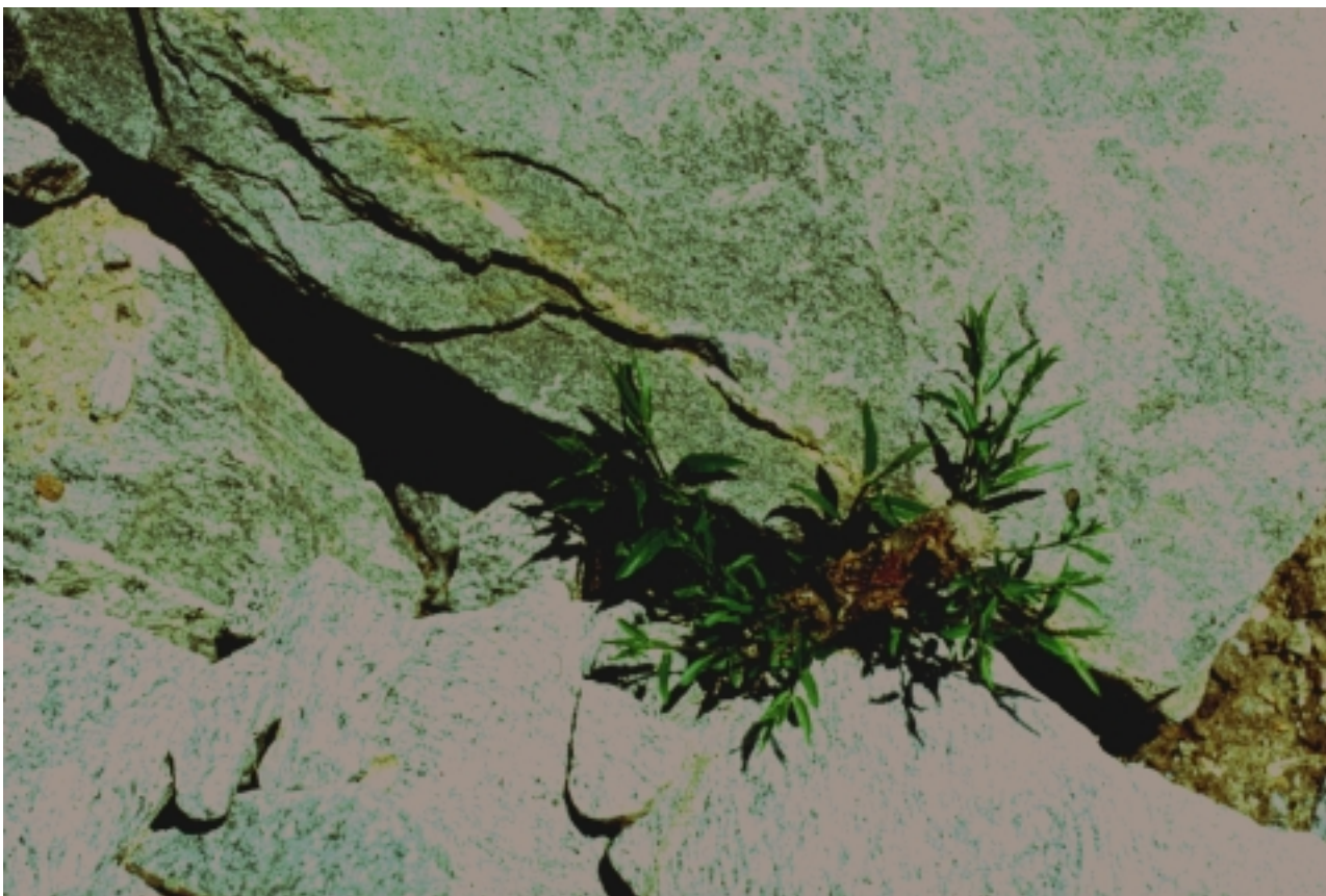
Figure 18–22 A newly established joint planting stake (H.M. Schiechl photo)
