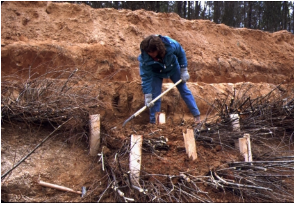
Figure 18–13 A branchpacking system being installed (Robbin B. Sotir & Associates photo)
