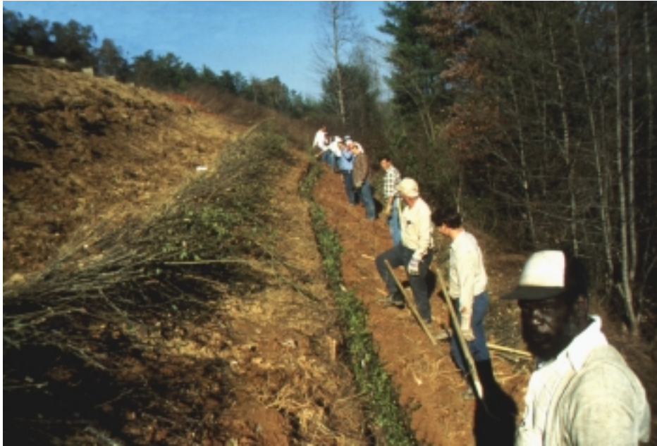
Figure 18-8a During installation (note size and depth of trench to size of live fascine bundle)
