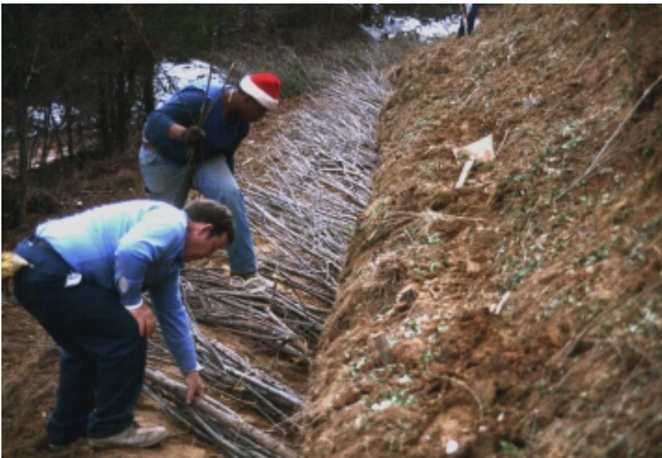
Figure 18-12b Placing live branch cuttings (Note crisscross configuration)
