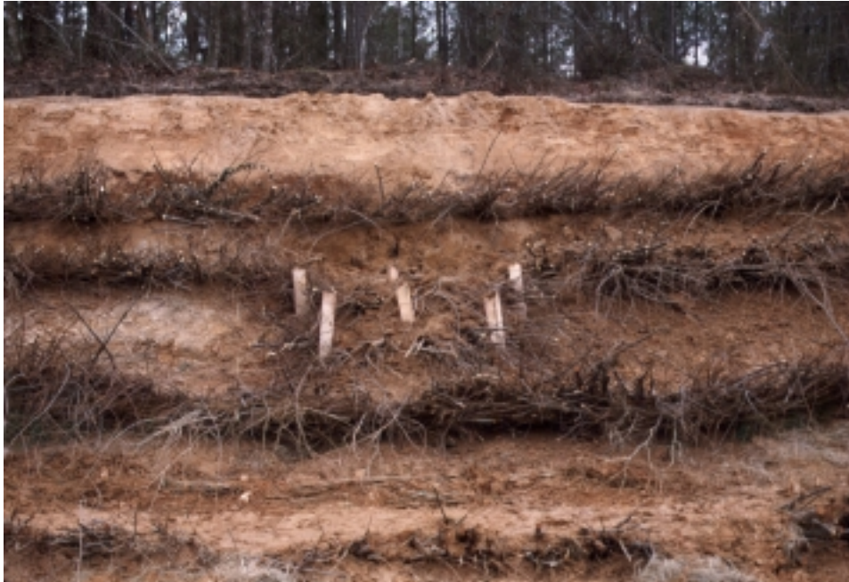
Figure 18-15a Newly installed system
