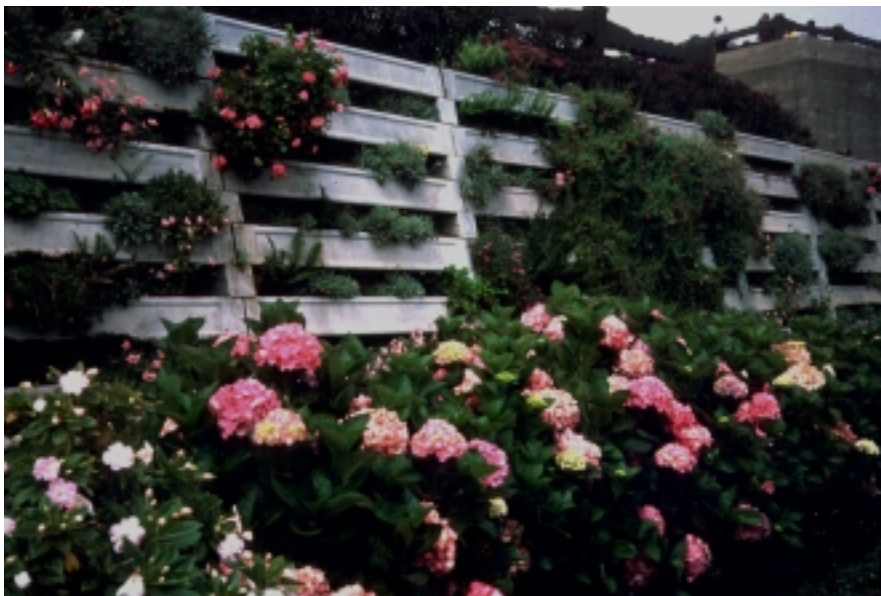
Figure 18-28b Open-front concrete cribwall with plantings in openings
