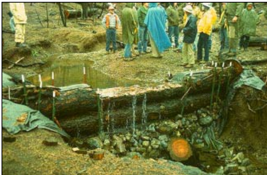
Photo 14.2 Logs being used to build gully stabilization structures in a fire damaged area. Physical or vegetative dams (dikes or debris retention structures) may be used to control sediment and stabilize gullies. Prevent water concentration before gullies form.
