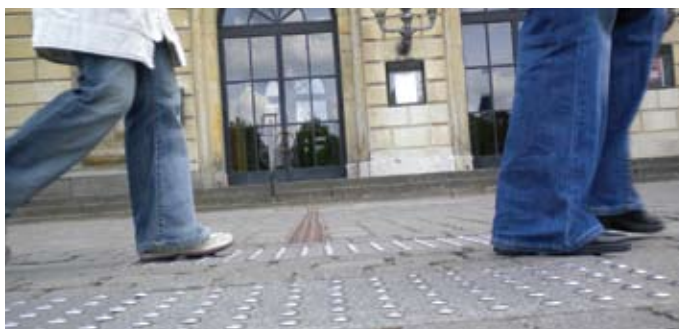
Figure 18. Tactile sidewalk strips leading to front door of public building in Copenhagen, Denmark.
