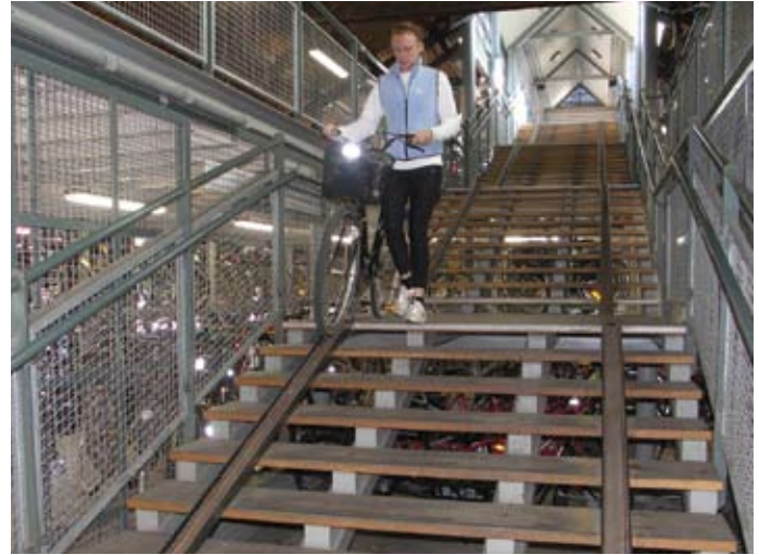
Figure 37. Bike-friendly steps in a multilevel transit station in Lund, Sweden.
