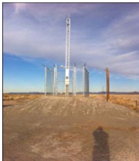
Figure NM-2. La Playa I-10 RWIS mile post 12.
