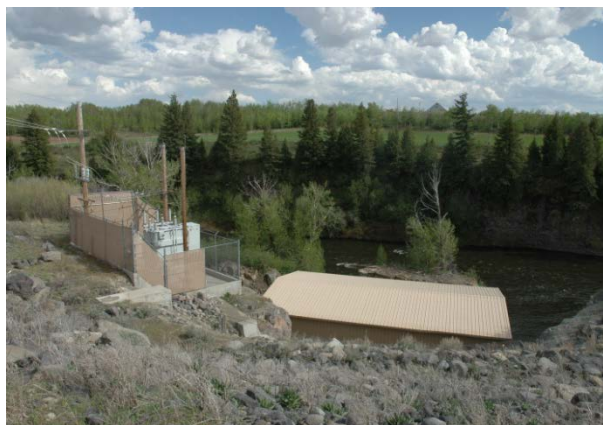
Figure 8-8. Small hydroelectric plant
