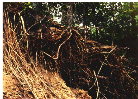
Figure 8. Exposed tree roots in overtopped dam.
