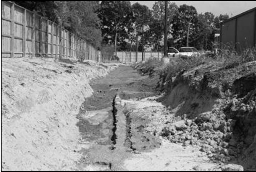
Fig. 1.8: Pea gravel diaphragm installation
