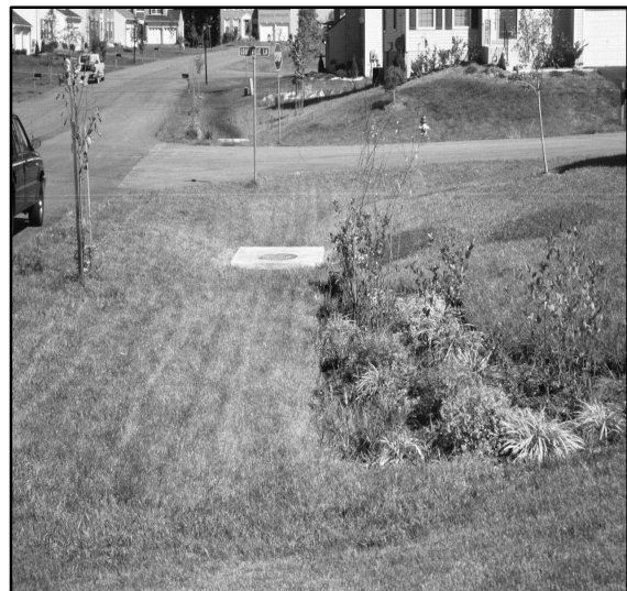
Figure 1.14: Swale-side bioretention
